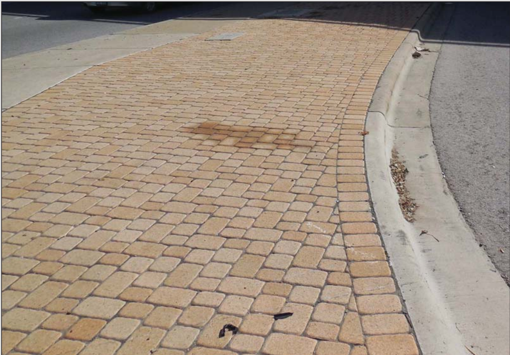
Fig 2.20- Concrete Pavers at Traffic Median
