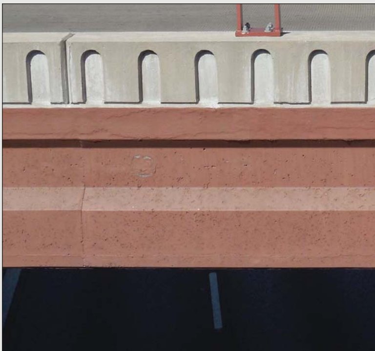
Fig. 2.7- Concrete “I” Beam
