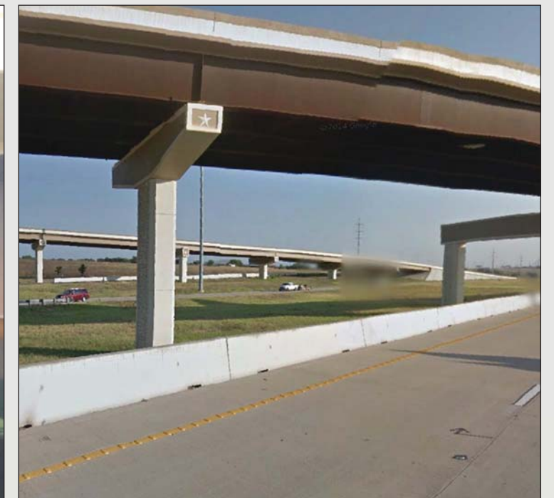
Fig. 4.10- Weathered Steel Beam, No Opaque Sealer
