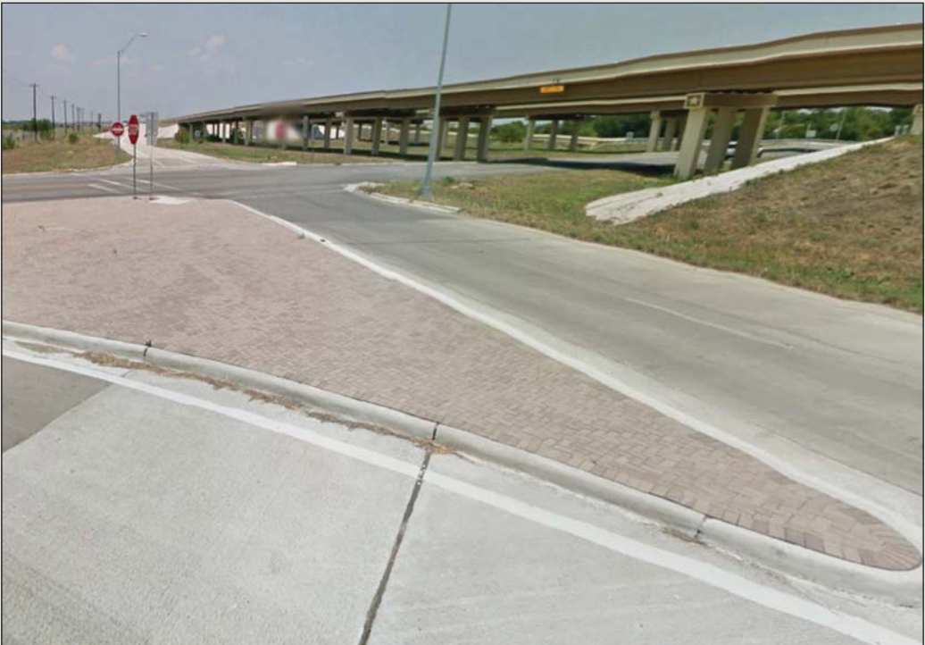
Fig 4.19- Concrete Pavers at Traffic Islands
