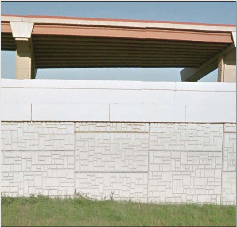
Fig 2.17- Concrete Traffic Barrier with Coping
