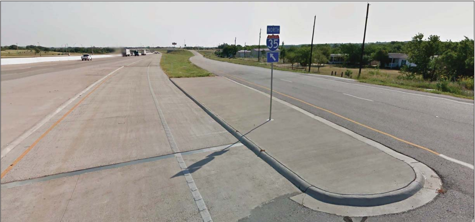
Fig 6.11- Concrete Rip Rap at Ramp Gore
