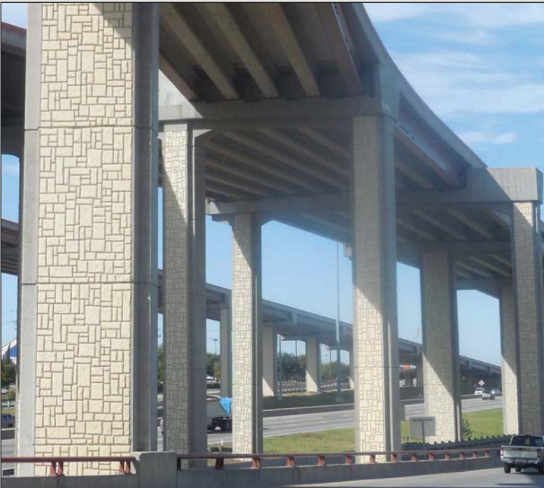
Fig. 2.6- Straddle Bent
