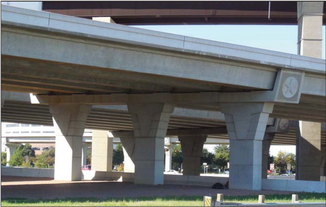
Fig. 3.4- Inverted "T", Multi-Column Bent, with Square "Longhorn" Columns and Five Point Star Bent Cap
