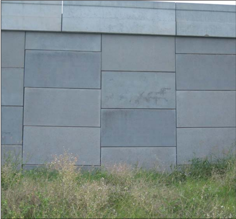
Fig 6.8- Concrete Traffic Barrier and Coping
