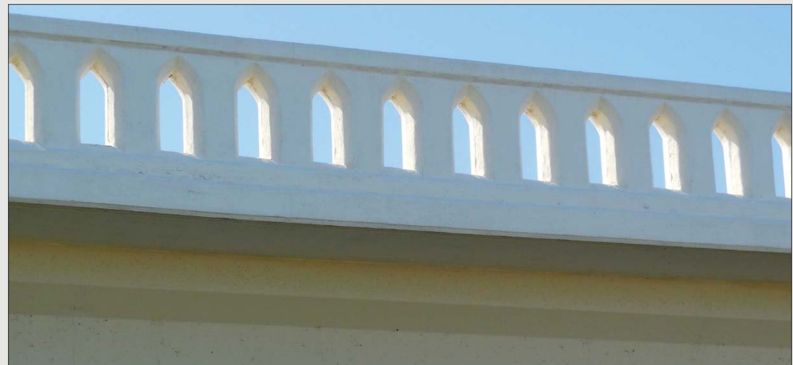
Fig. 1.13- Concrete Traffic Barrier with Arch Openings
