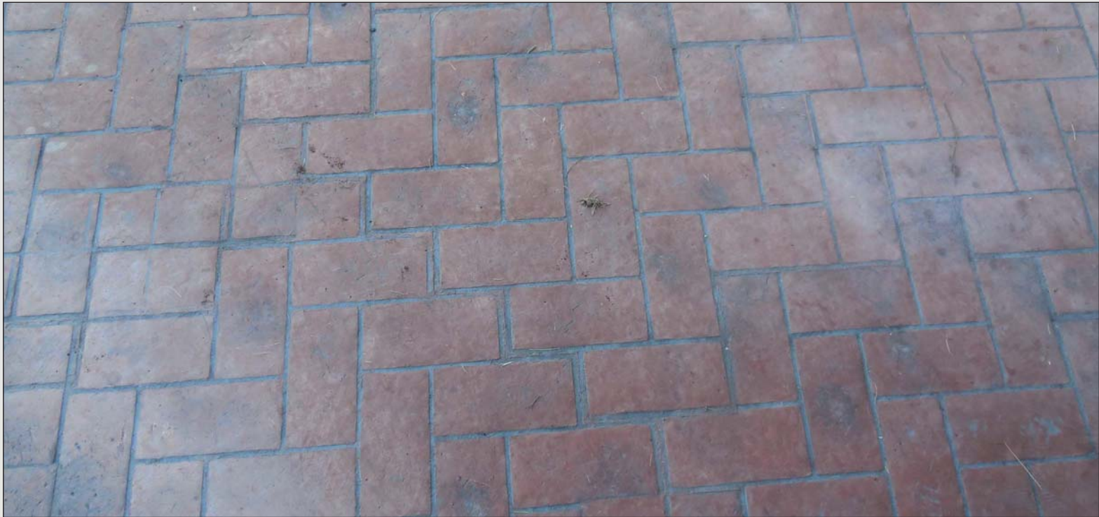
Fig 3.20- Terra Cotta Stamped Concrete, Herringbone Brick Pattern
