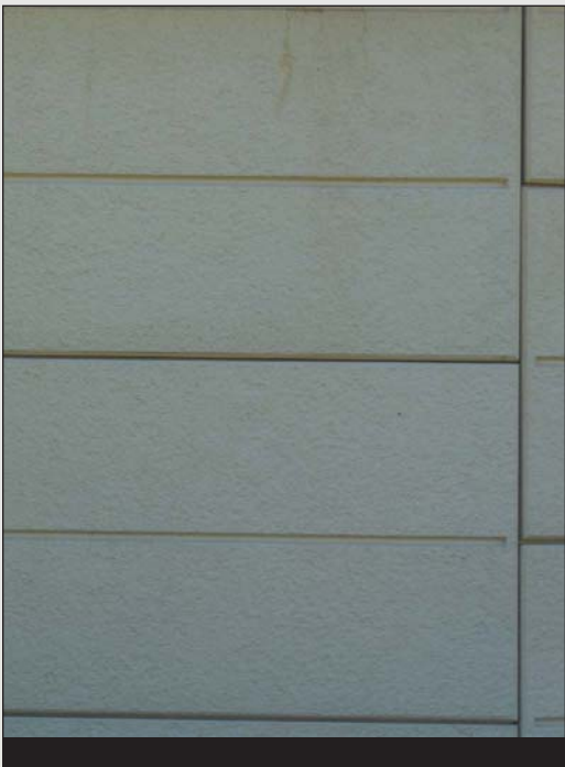
Fig 1.10- Retaining Wall Reveals
