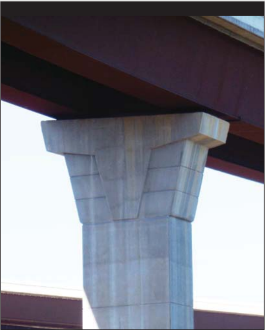
Fig. 3.1- Typical Hammerhead Bent with Rectangular "Longhorn" Column
