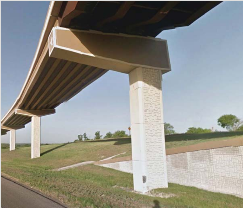
Fig. 2.7- Cantilever Bent (Mod.): Cantilever Bent to complement aesthetic of Existing Bents (Figure 2.1, From SH 45SE)
