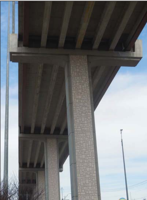
Fig. 2.4- Inverted "T" Bent
