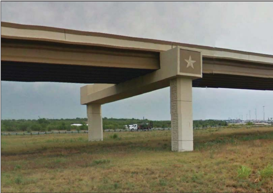
Fig. 4.4- Inverted "T", Multi-Column Bent
