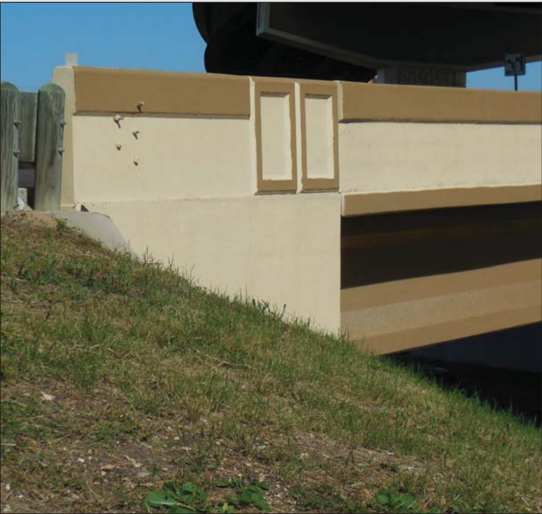
Fig 4.18- Concrete Traffic Barrier Bridge End Detail
