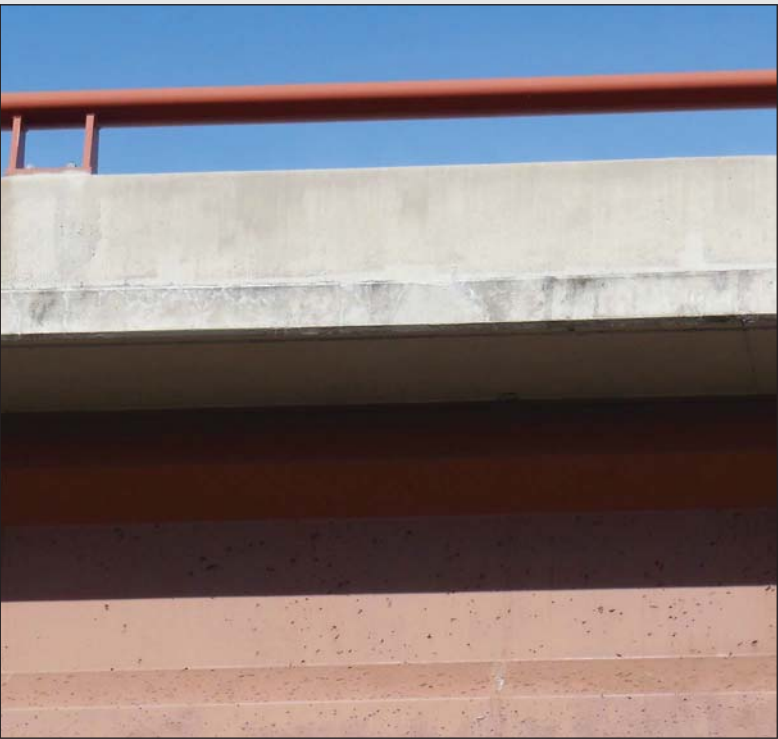
Fig 2.18- Concrete Traffic Barrier with Bridge Railing
