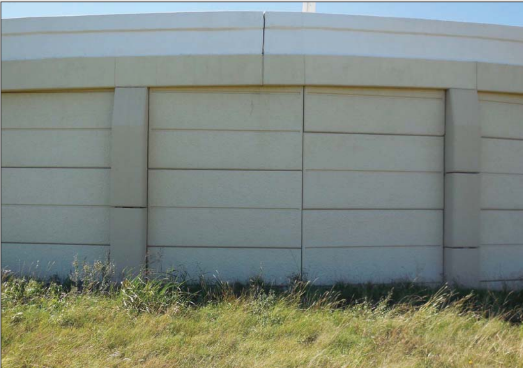
Fig 1.7- MSE Retaining Wall with Reveals and Concrete Columns
