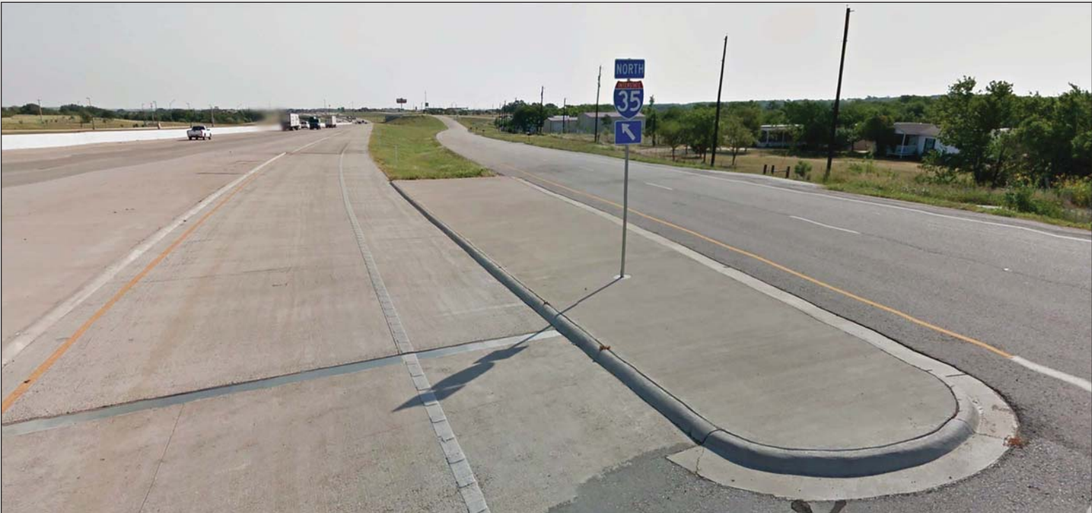
Fig 2.21- Concrete Rip Rap at Ramp Gore
