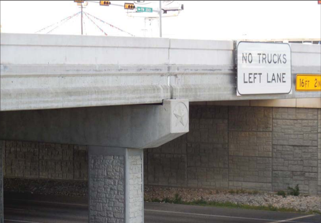
Fig. 4.16- Concrete Traffic Barrier
