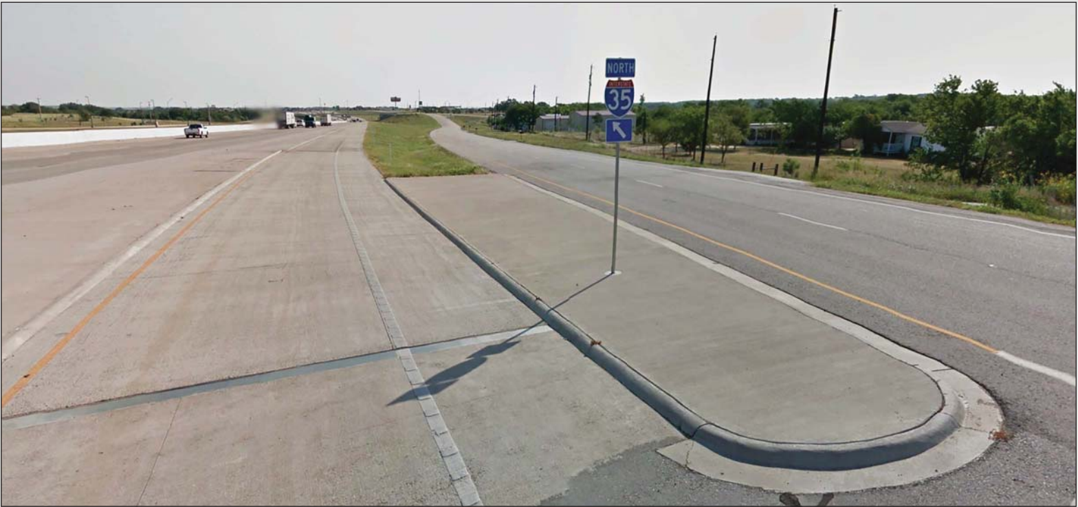
Fig 4.21- Concrete Rip Rap at Ramp Gore
