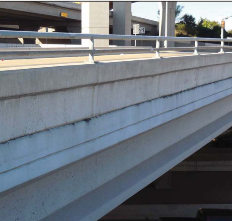
Fig 3.17- Traffic Barrier with Bridge Railing
