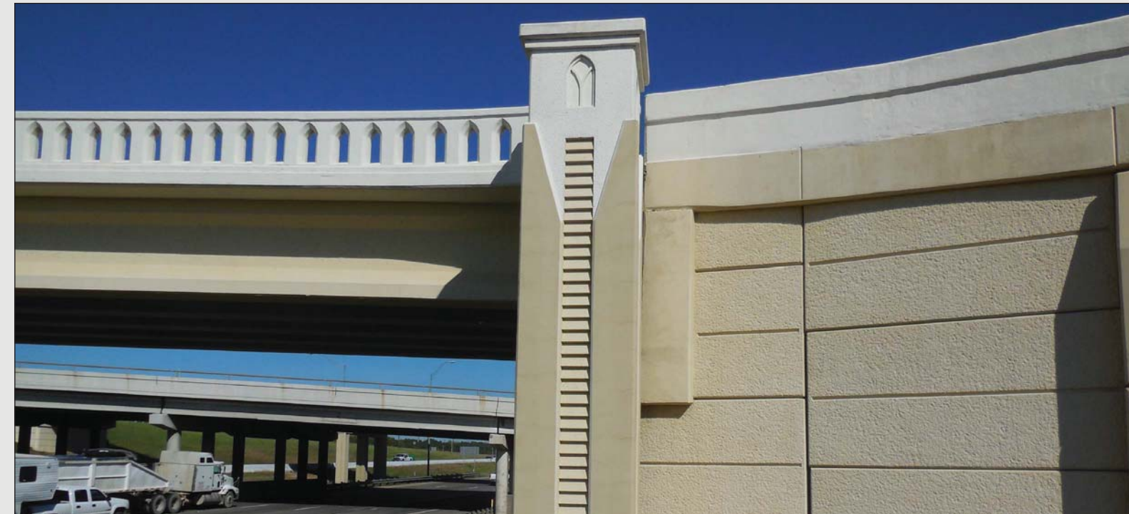
Fig 1.5- Square Belltower Bridge End Detail, tan and white sealer
