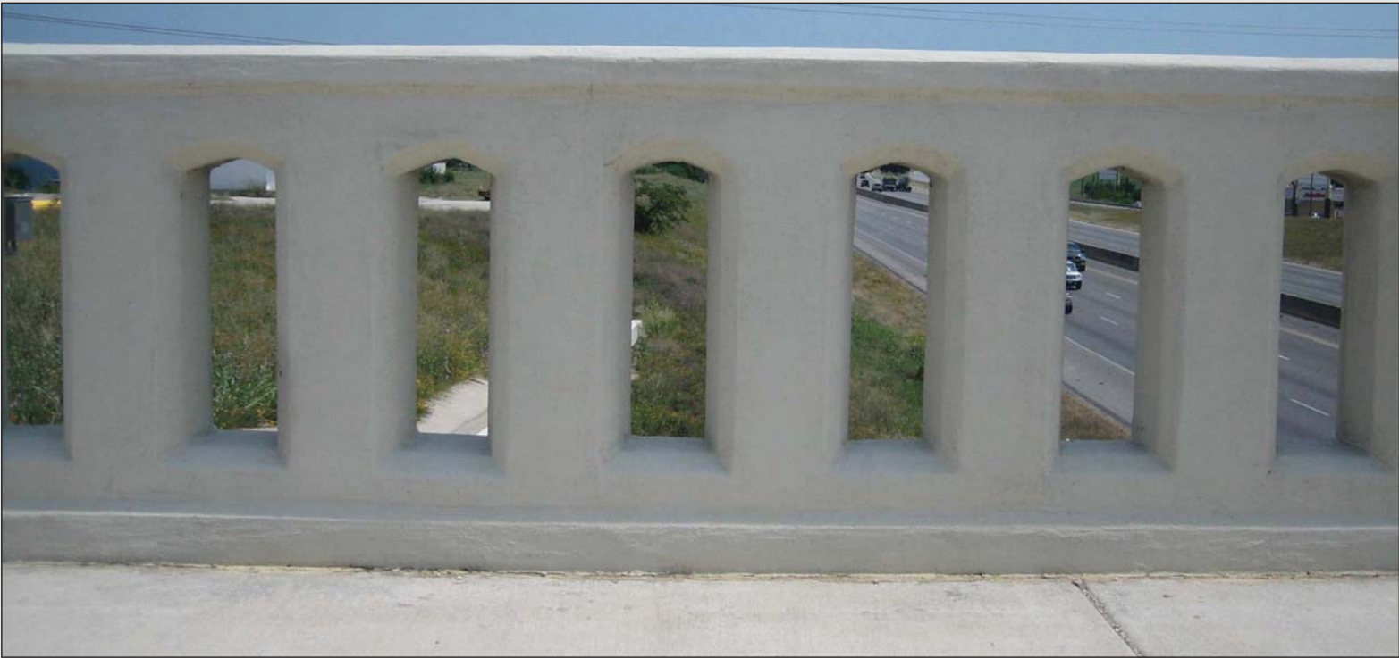
Fig 5.12- Concrete Traffic Barrier with Arch Openings
