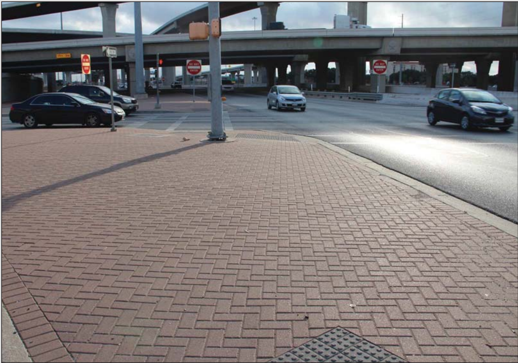
Fig 3.19- Concrete Pavers at Traffic Island
