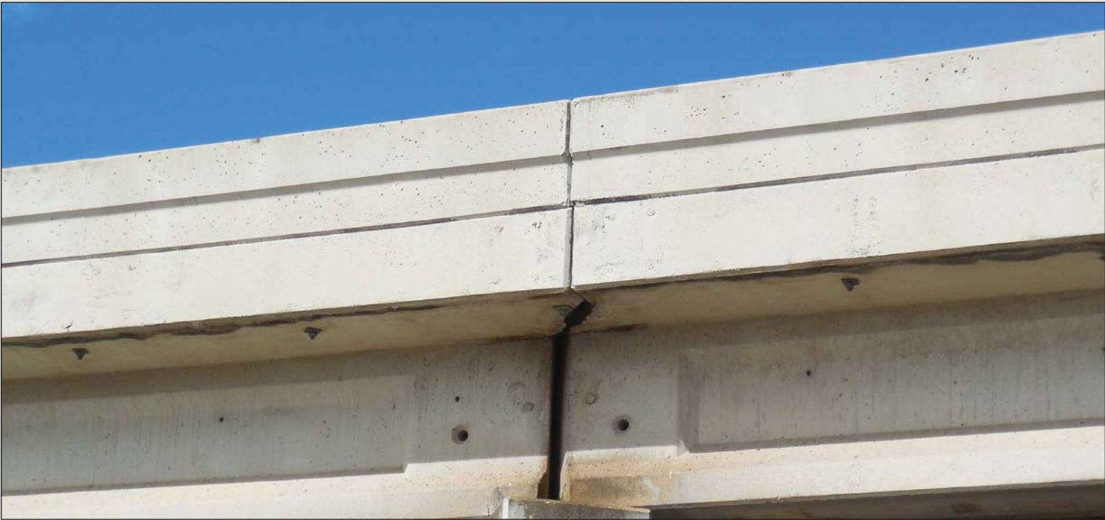
Fig 6.9- Concrete Traffic Barrier
