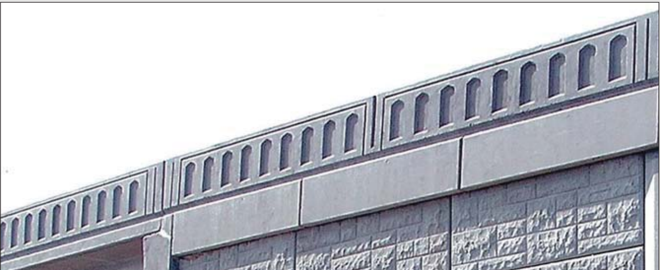
Figure 3.48 - Modified SSTR Traffic Barrier
