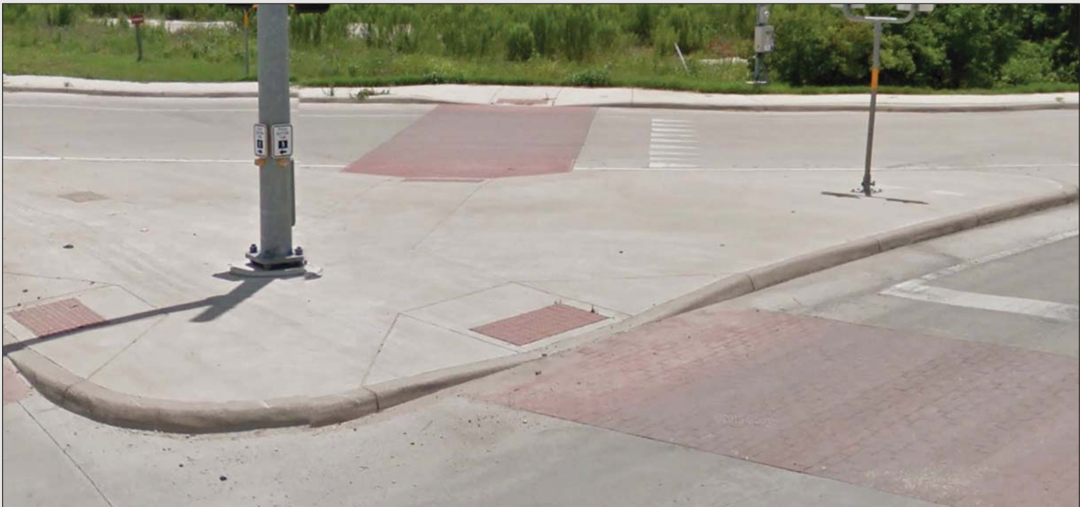
Fig 5.13- Concrete Rip Rap at Median
