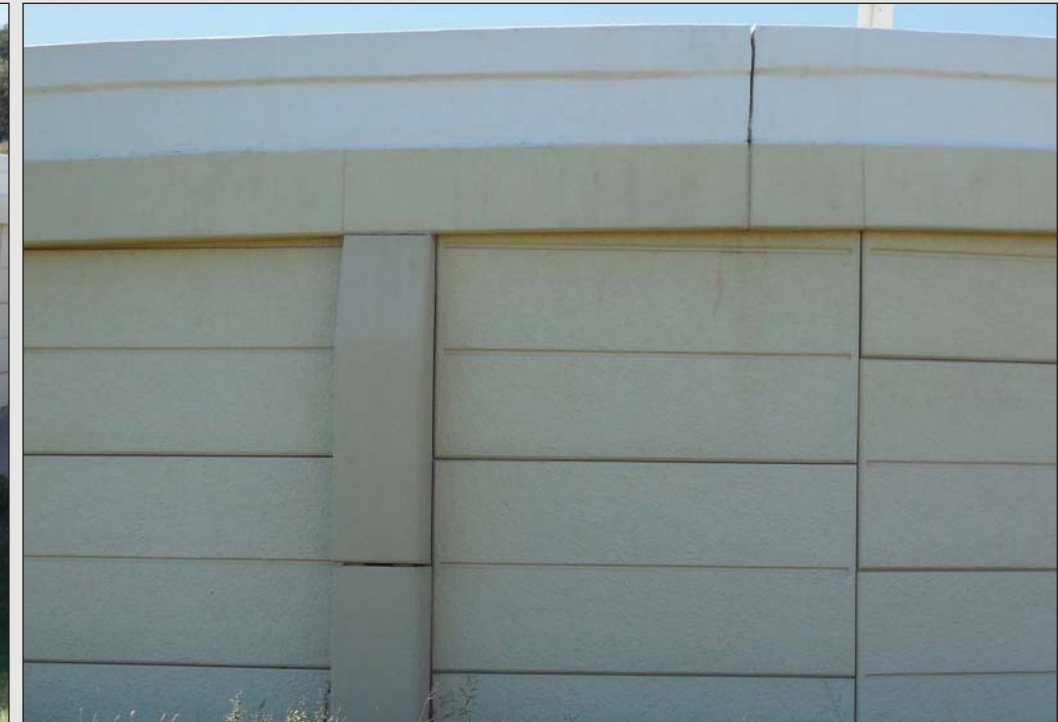
Fig 1.12- Concrete Traffic Barrier with Concrete Coping
