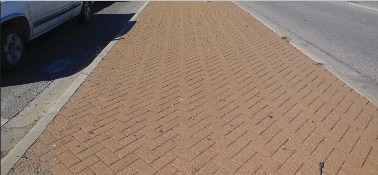
Fig 1.14- Concrete Pavers at Traffic Median
