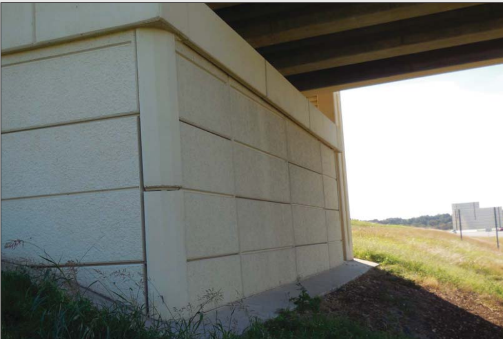
Fig 1.9- MSE Panel Abutment Wall, Concrete Panel Bridge Ends, and Coping
