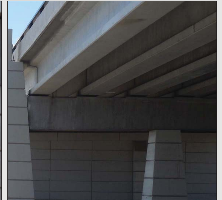
Fig. 4.8- Concrete “I” Beam, Brown Opaque Sealer Along Underside of Beam
