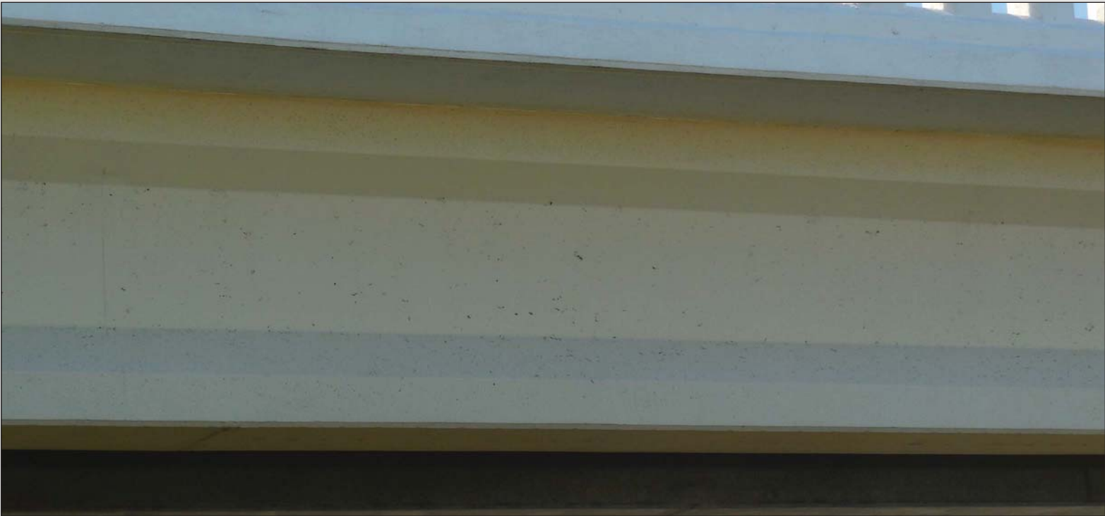
Fig. 1.6- Concrete “I” Beam, Tan Sealer Along Outer Face of Beam
