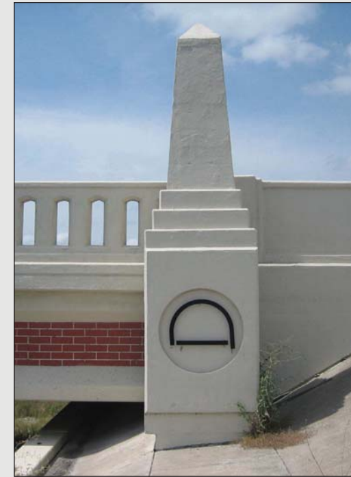
Fig 5.3- Bridge Bent End Detail with Ranch Symbol
