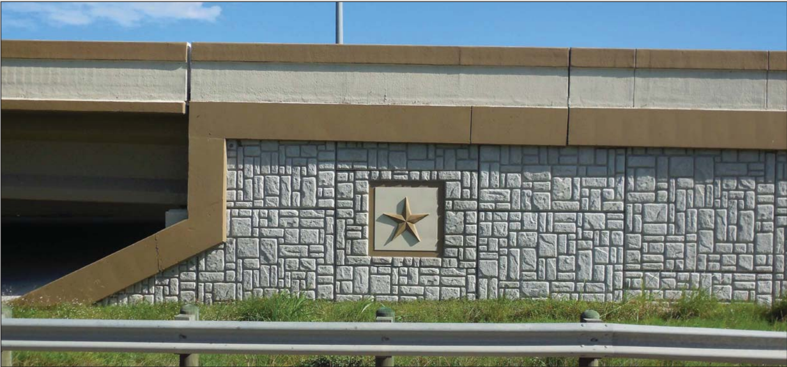
Fig 4.14- MSE Panels with Signature MSE Panel
