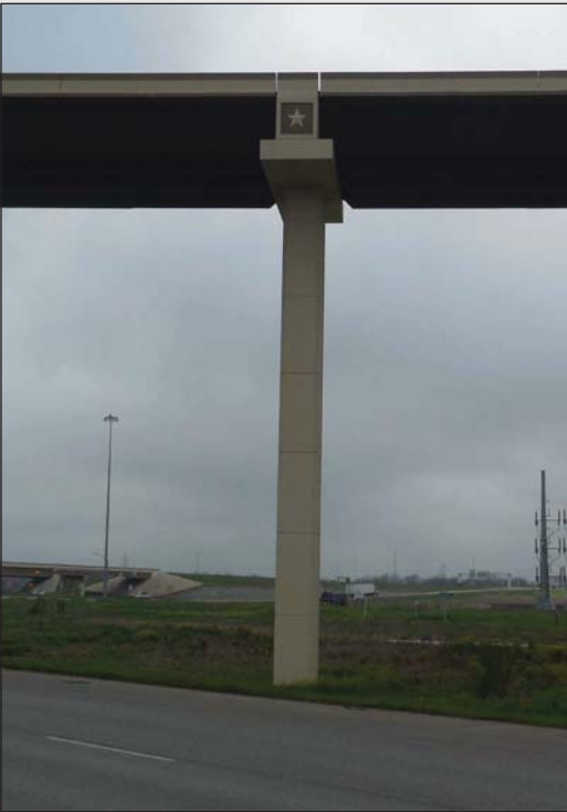
Fig. 4.3- Inverted "T" Bent
