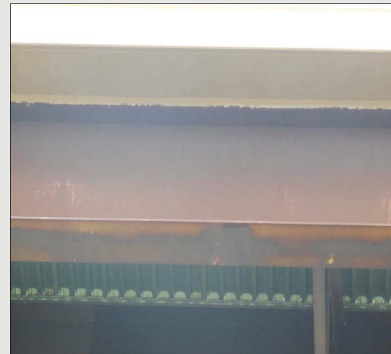
Fig. 4.9- Weathered Steel Beam, No Opaque Sealer
