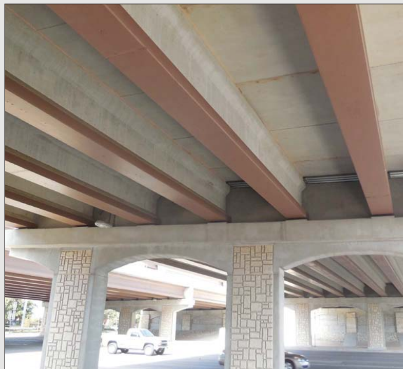
Fig. 2.8- Concrete “I” Beam
