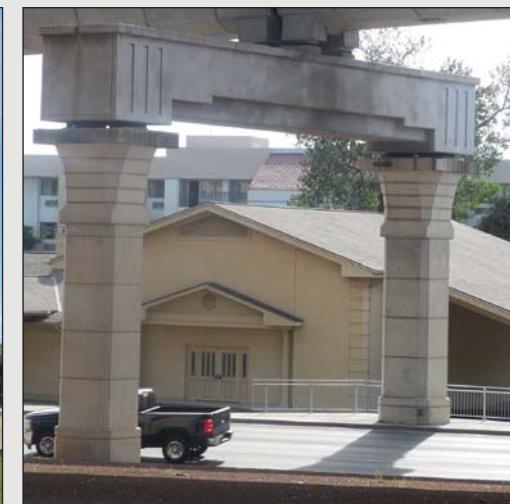
Fig 3.22 - Straddle Bent
