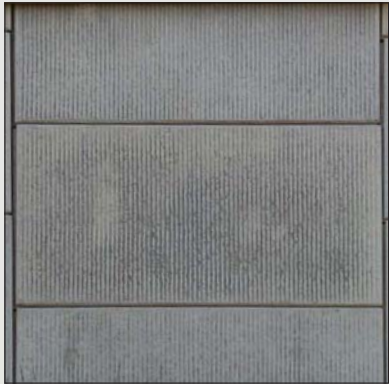
Fig 3.11- Ben White Blvd., Fractured Fin, MSE Panels
