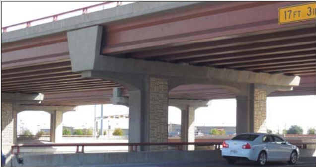
Fig. 2.2- Multi-Column Bent with Mask Wall (Direct Connector Underpass)
