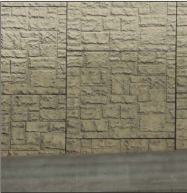
Fig 3.10- Yager Ln., Ashlar, MSE Panels
