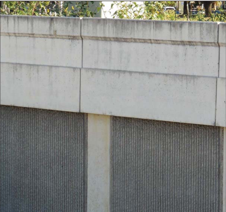
Fig 3.15- Concrete Traffic Barrier with Coping
