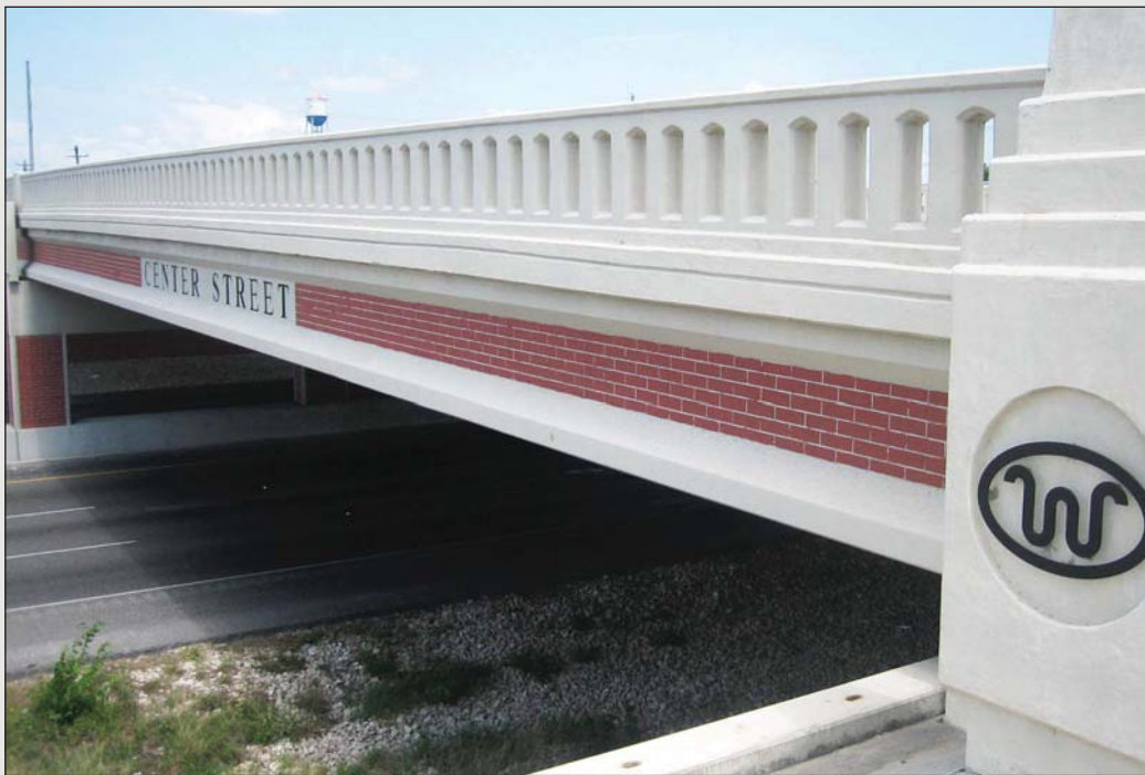
Fig. 5.5- Concrete "I" Beams
