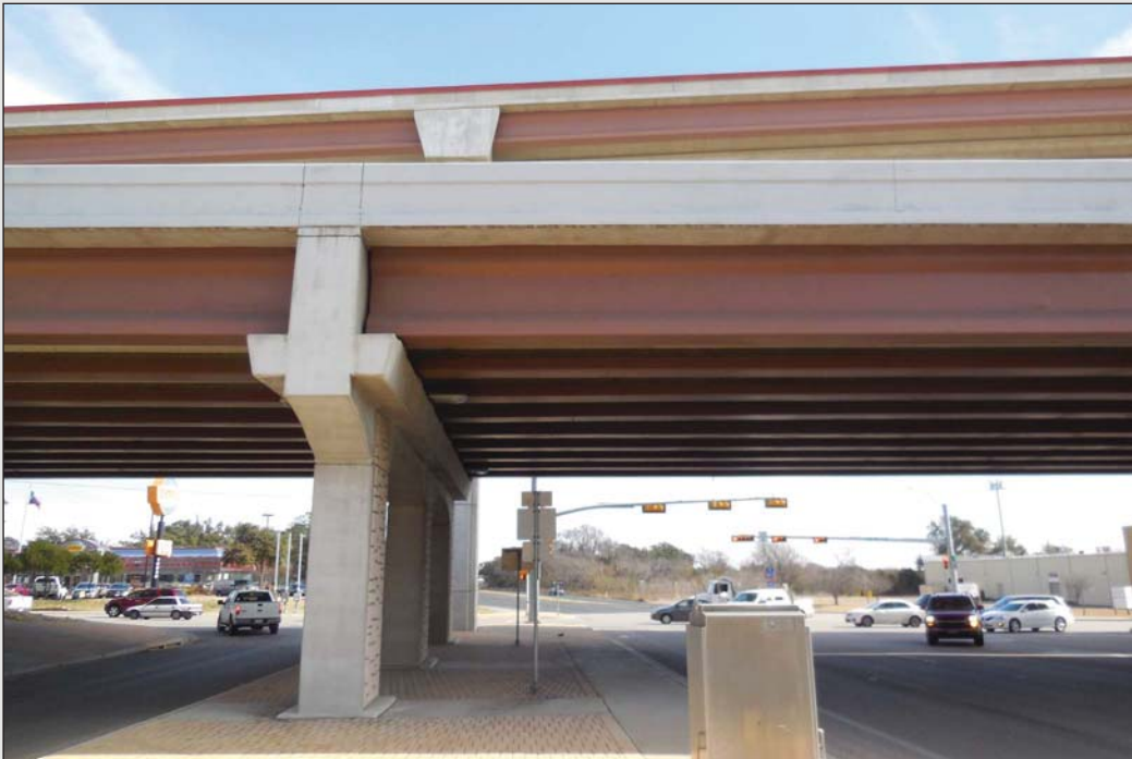
Fig. 2.5- Multi-Column Inverted "T" Bent
