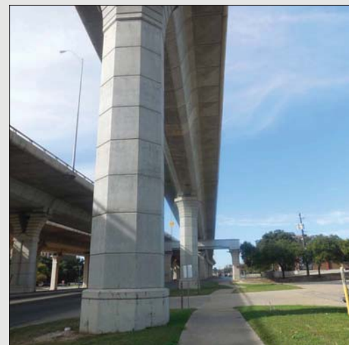
Fig 3.21- Single Column Bent
