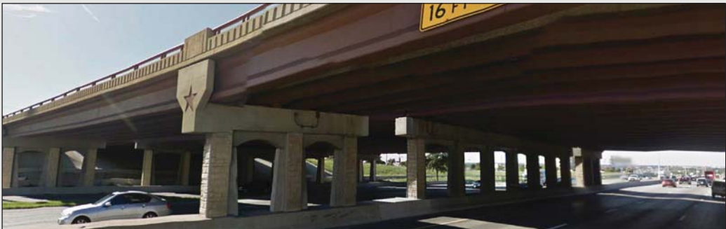
Fig. 2.3- Multi-Column Bent with Mask Wall (Standard Bridge Underpass)
