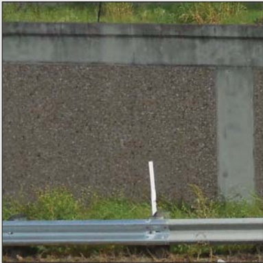
Fig 3.13- US 290, Exposed Aggregate, CIP with Concrete Banding
