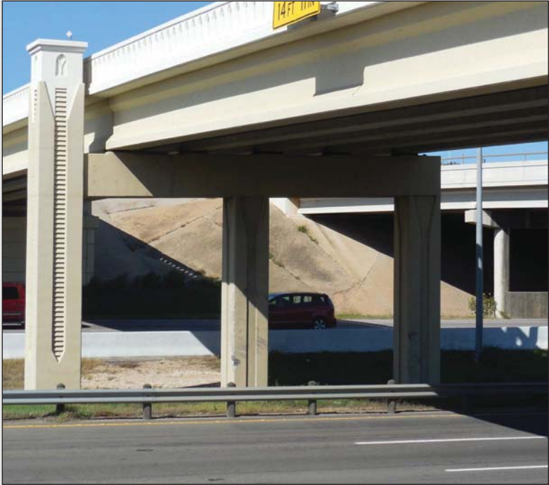
Fig 1.2- Multi-Column Bent with a Single Bell Tower Detail
