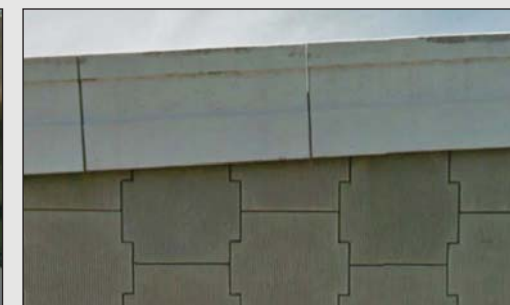
Fig 3.25- Concrete Traffic Barrier with Coping
