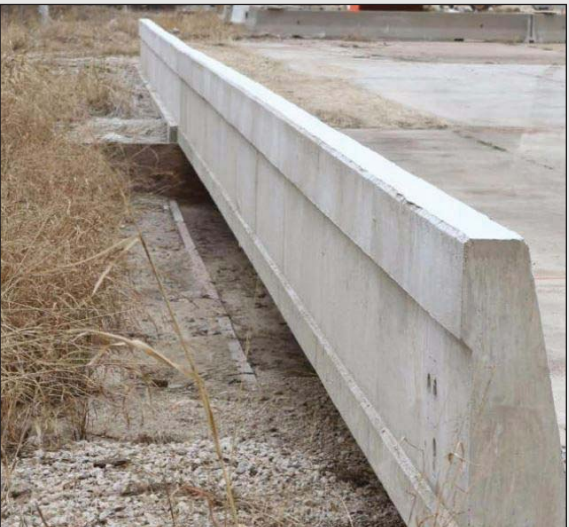
Figure 3.49 - SSTR Traffic Barrier
