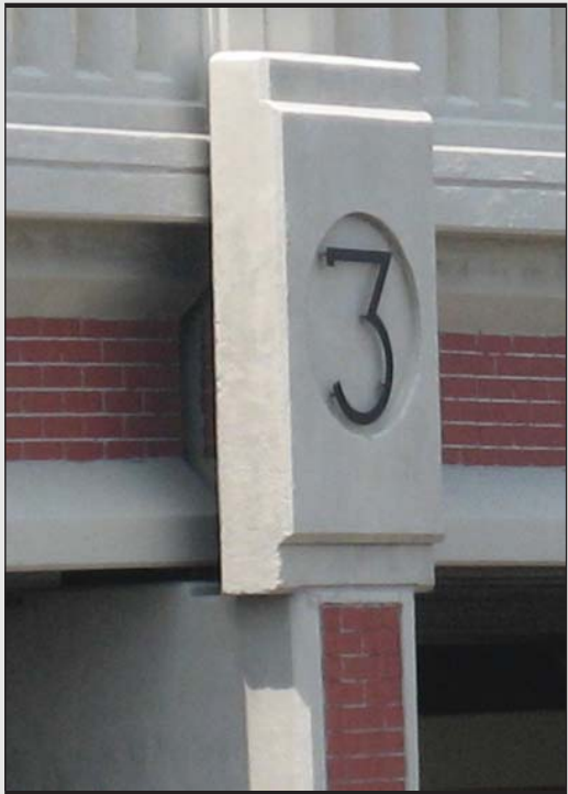
Fig. 5.1- Bent Cap with Mask Wall
