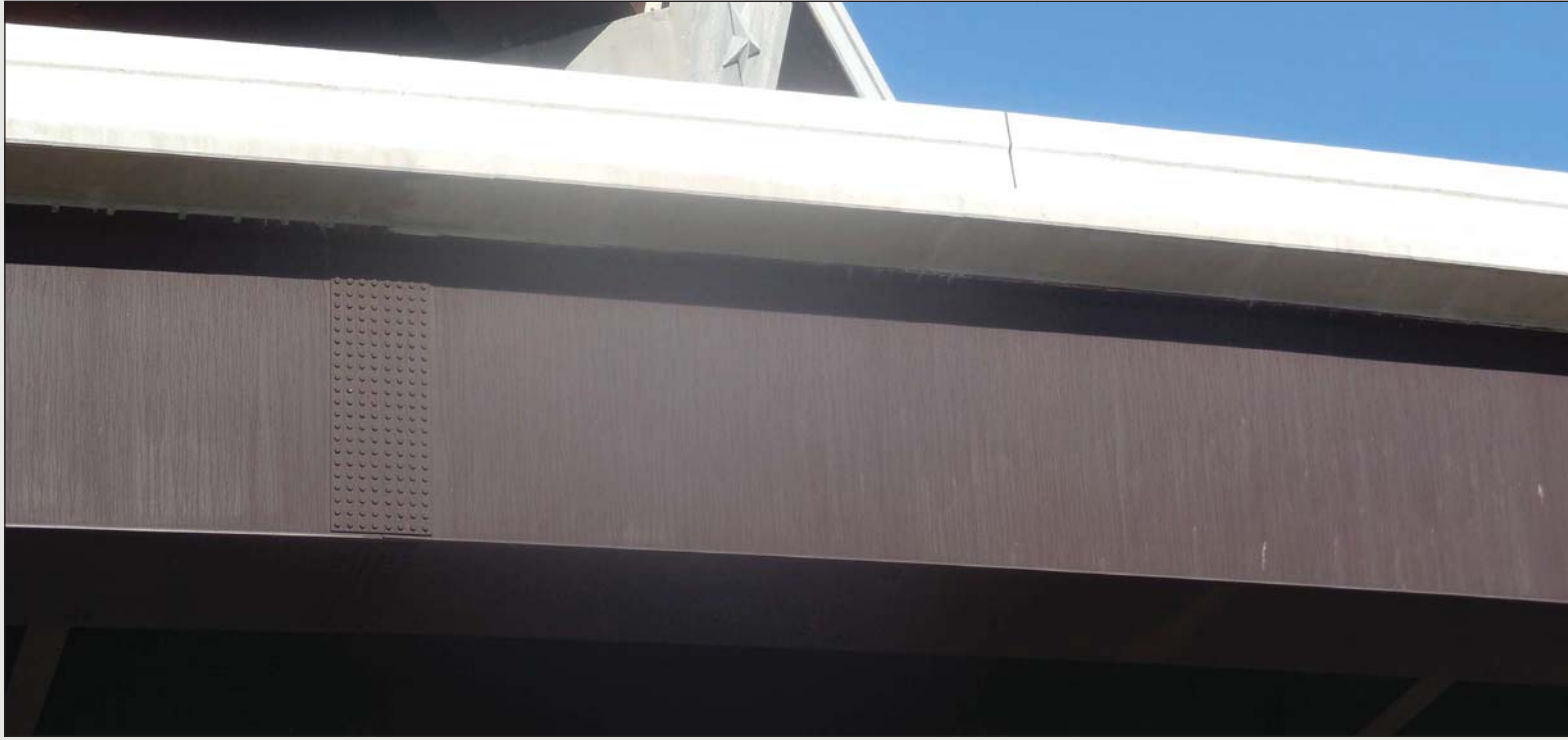
Fig. 2.9- Existing Weathered Steel Beam
