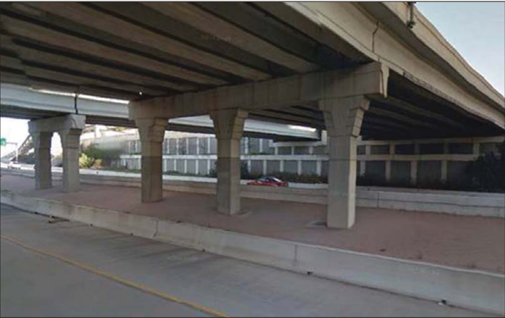
Fig. 3.2- Multi-Column Bent with Rectangular "Longhorn" Column
