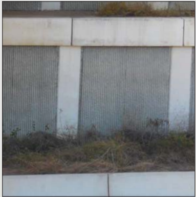
Fig 3.12- Ben White Blvd., Fractured Fin, CIP with Concrete Banding
