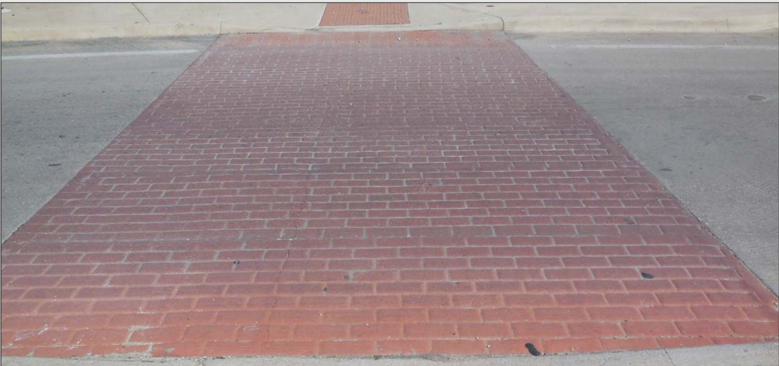
Fig 5.15- Terra Cotta Stamped Concrete, Running Bond Brick Pattern at Crosswalks
