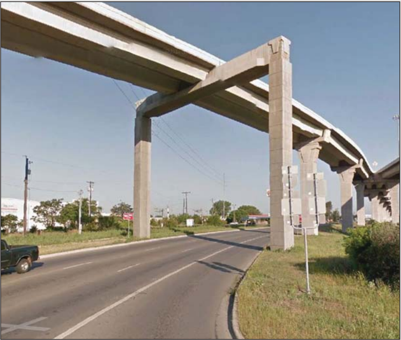
Fig. 3.5- Straddle Bent with "Longhorn" Column
