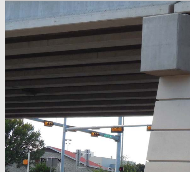
Fig. 4.7- Concrete “I” Beam
