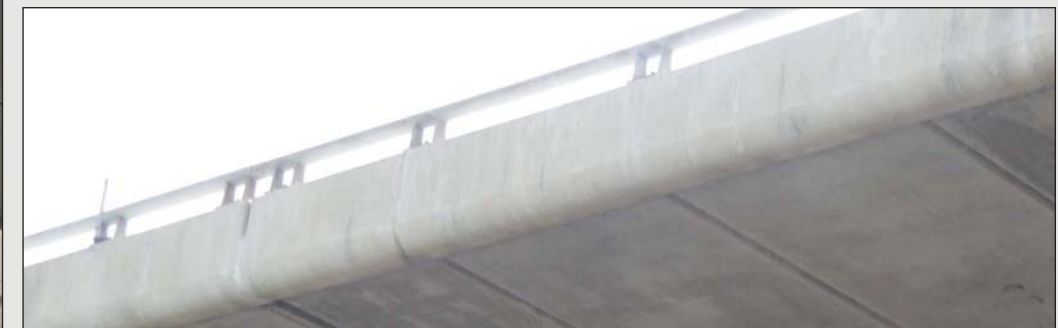
Fig 3.27- Traffic Barrier and Bridge Rail
