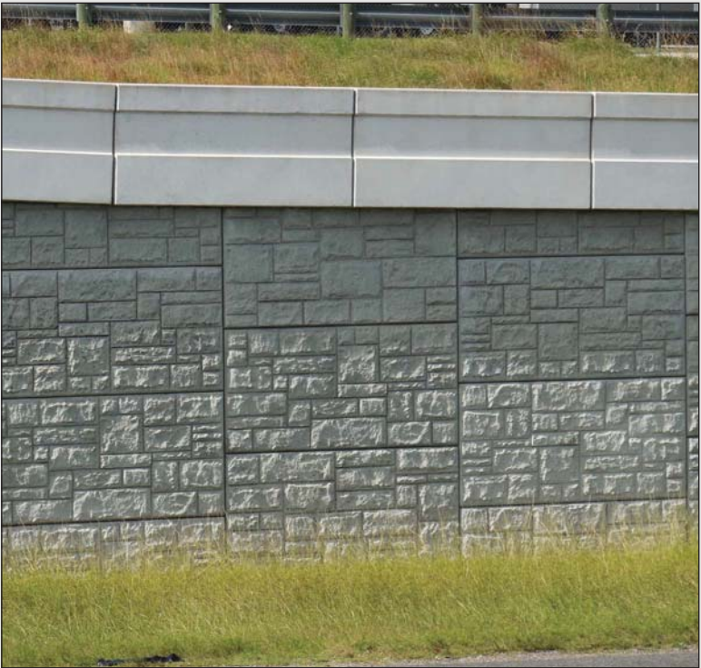
Fig 4.17- Concrete Traffic Barrier with Coping
