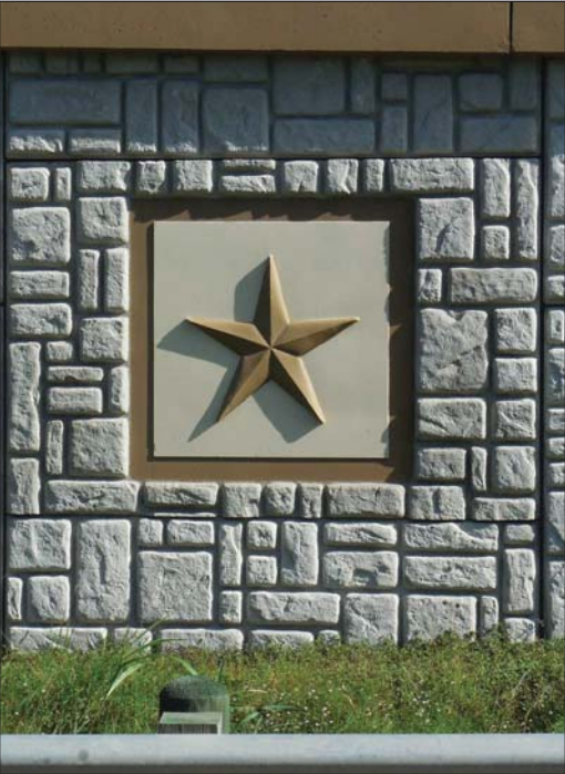
Fig 4.13- Signature MSE Panel Detail
