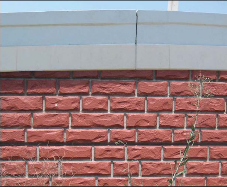
Fig 5.11- Concrete Traffic Barrier with Concrete Coping
