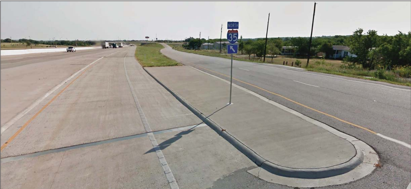
Fig 5.14- Concrete Rip Rap at Ramp Gore
