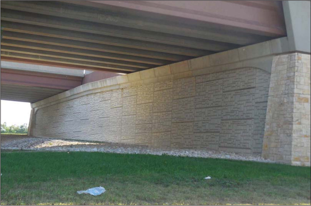
Fig 2.13- MSE Abutment Wall, (Image modified to reflect the removal of the wall base panel)
