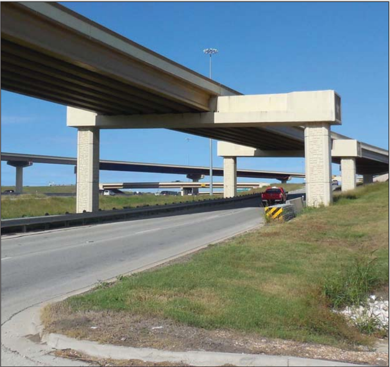
Fig. 4.5- Straddle Bent
