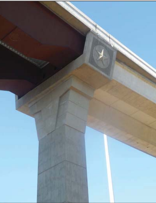
Fig. 3.3- Inverted "T" Bent, with "Longhorn" Column and Five Star Bent Cap
