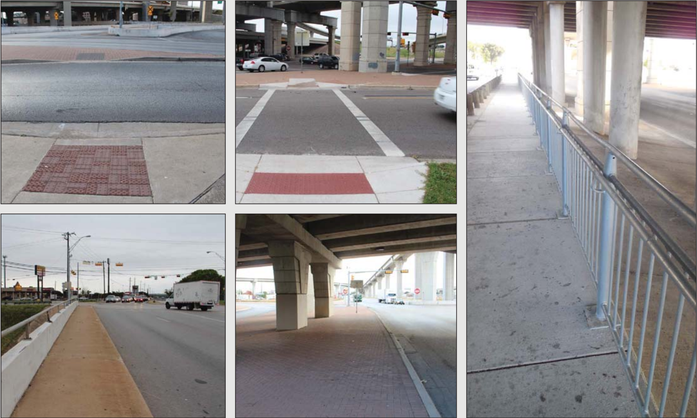
Figs A.8-A.12 Pedestrian Facilities Include ADA Ramps, Crosswalks, Sidewalks, and Hardscape Paving (clockwise from upper left)
