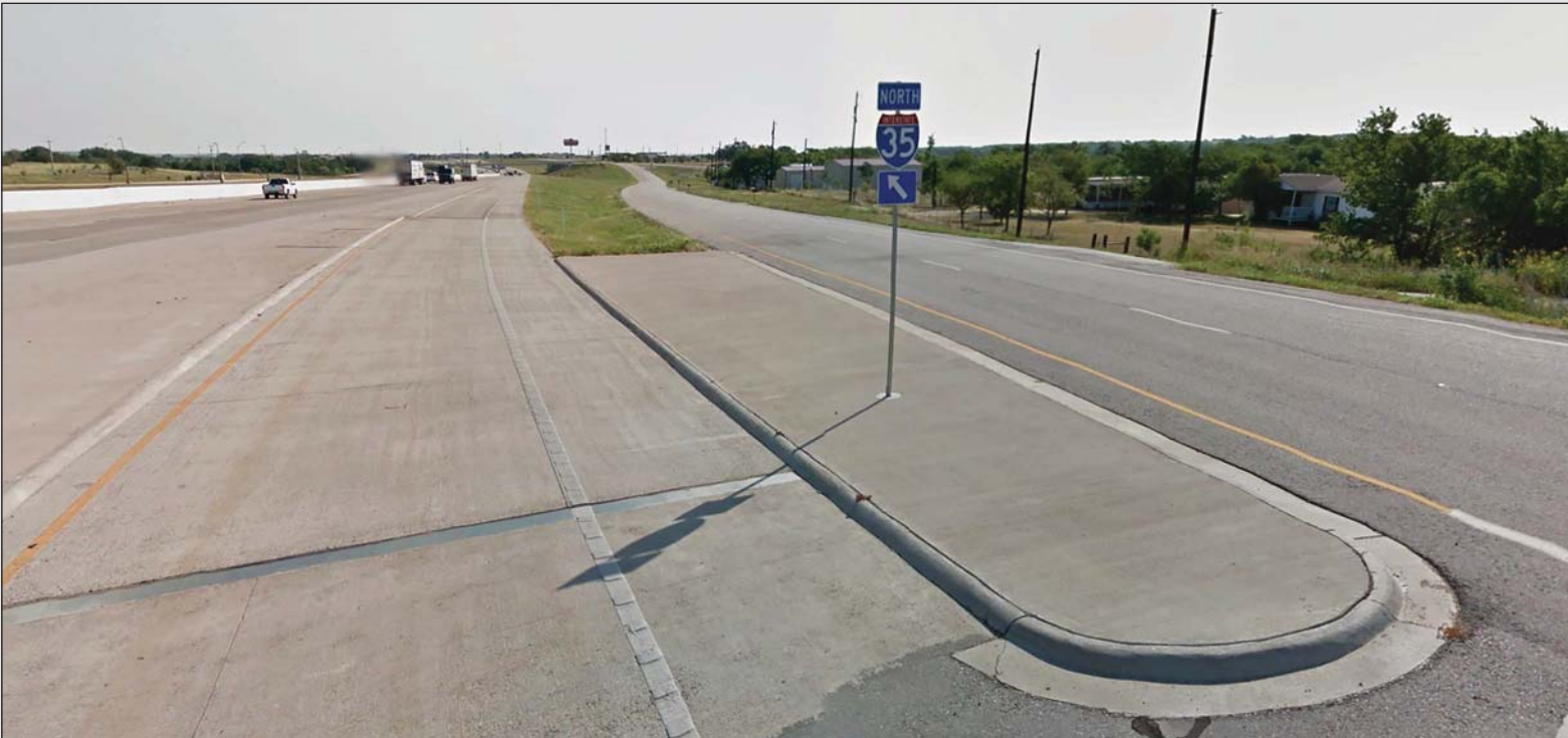
Fig 1.16- Concrete Rip Rap at Ramp Gore
