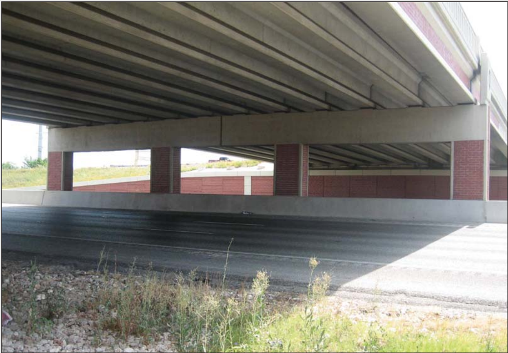
Fig. 5.2- Multi-Column Bent with Mask Wall
