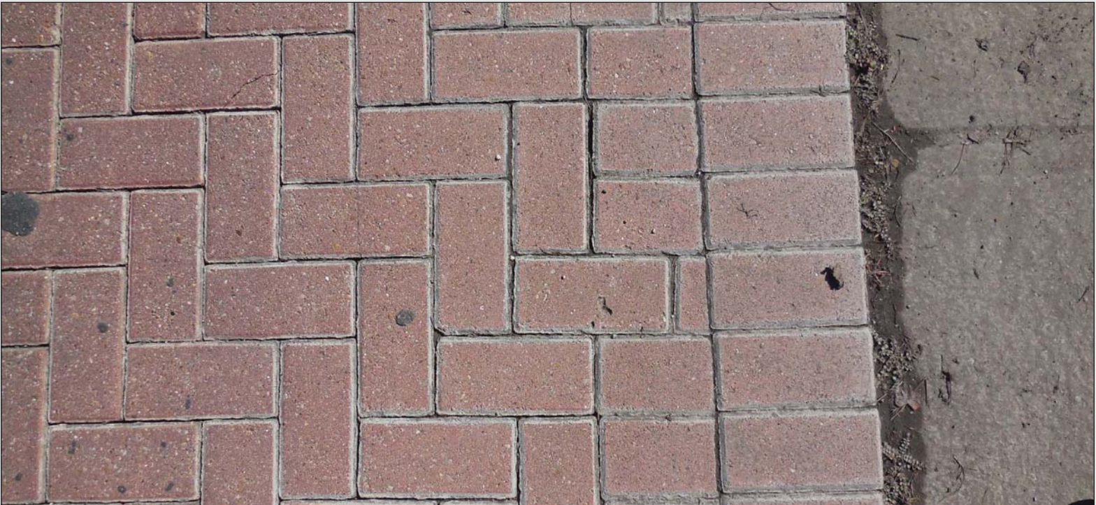
Fig 6.10- Concrete Pavers, Herringbon Pattern with a Solider Course
