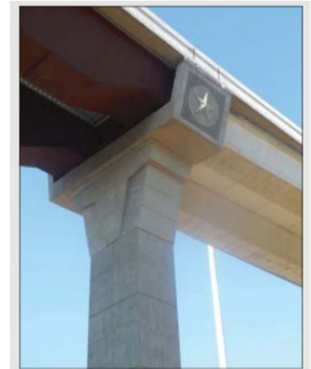
Fig. 3.3- Inverted "T" Bent, with "Longhorn" Column and Five Star Bent Cap
