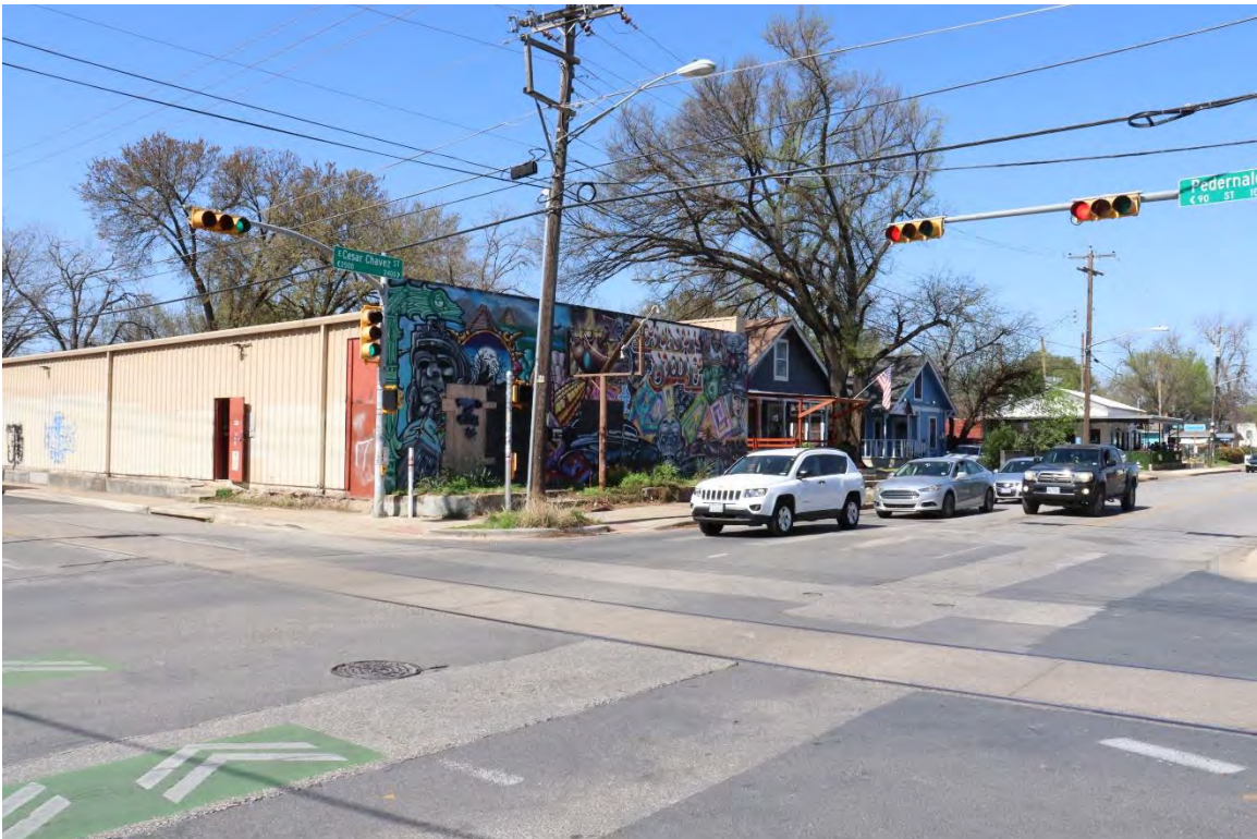
2400 block, view facing southwest. Resource 1120 visible at center.
