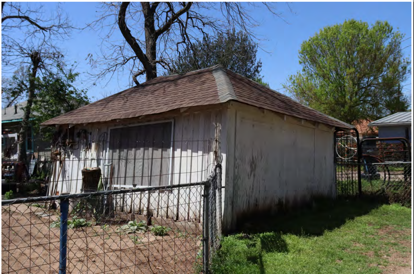
View facing southwest.
