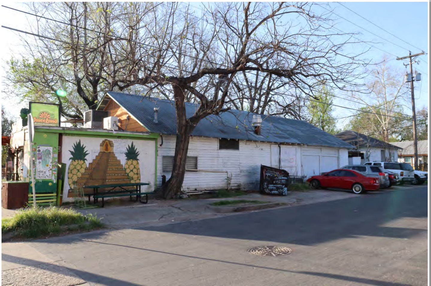
View facing southeast.
