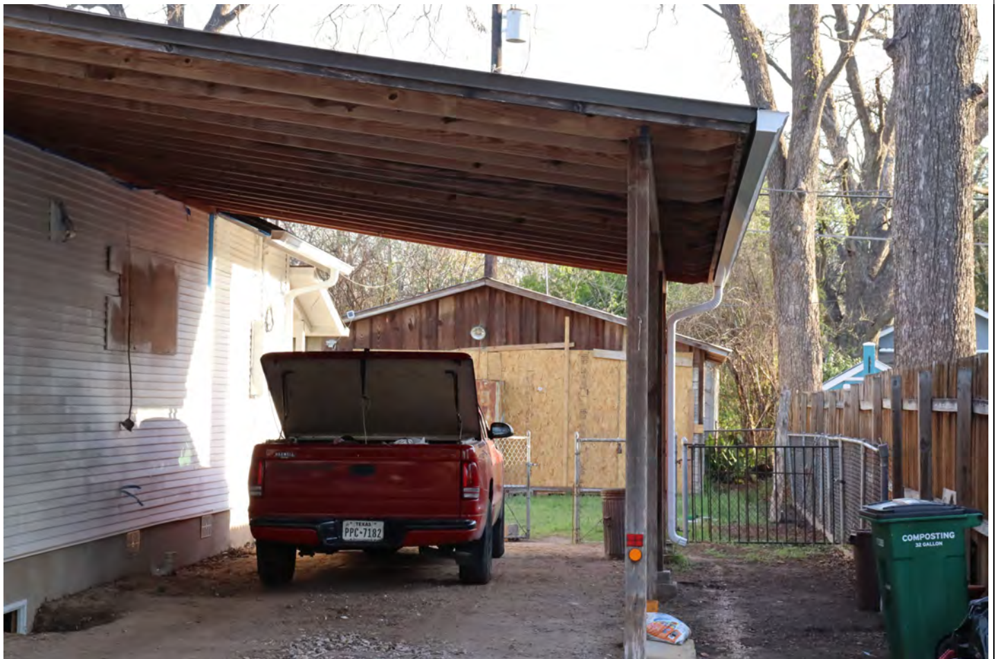
View facing north.
