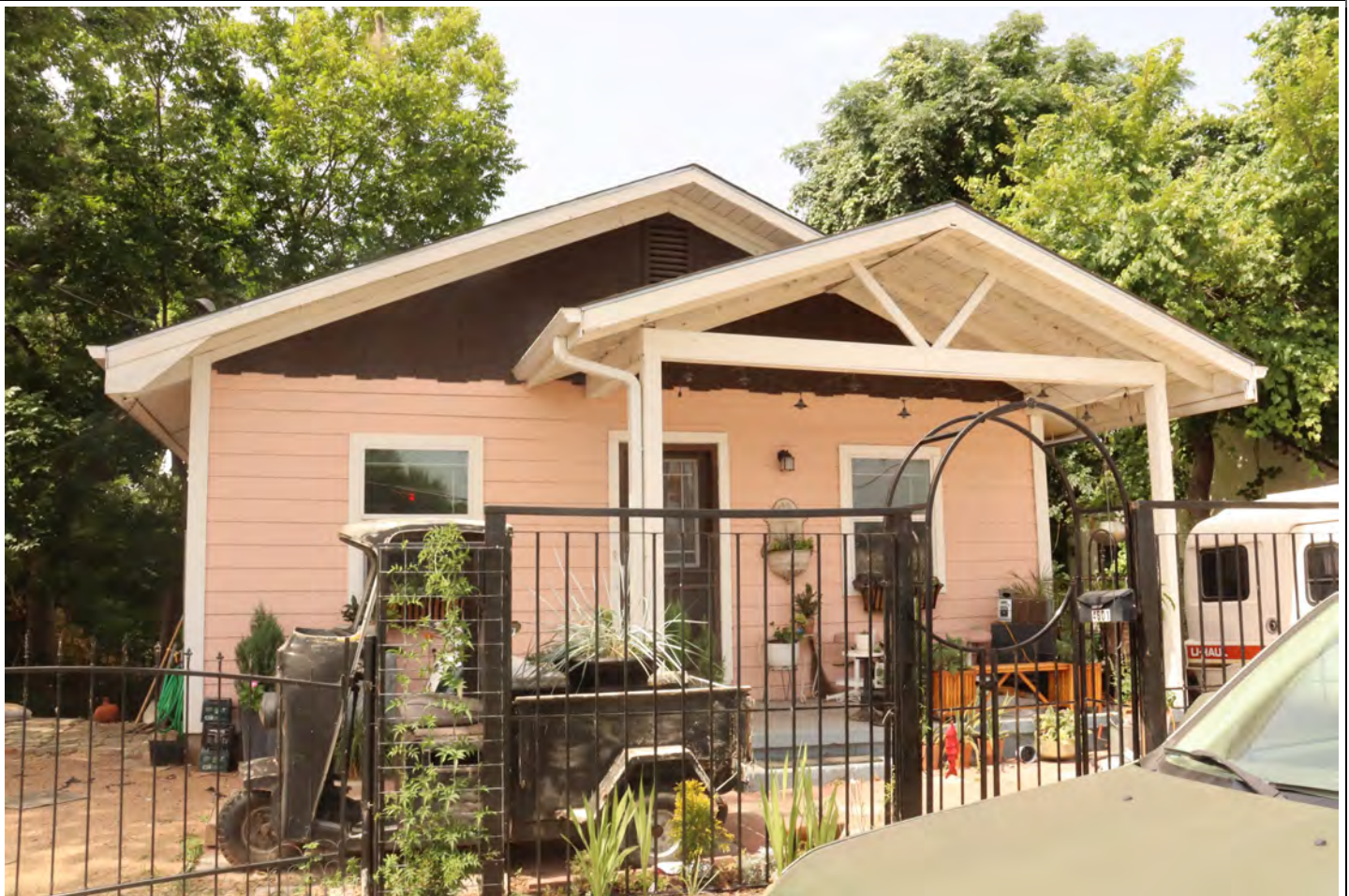
View facing southwest.
