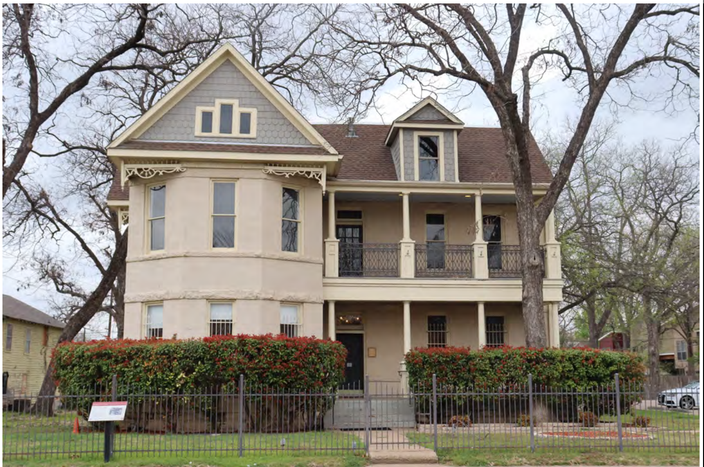
View facing north.
