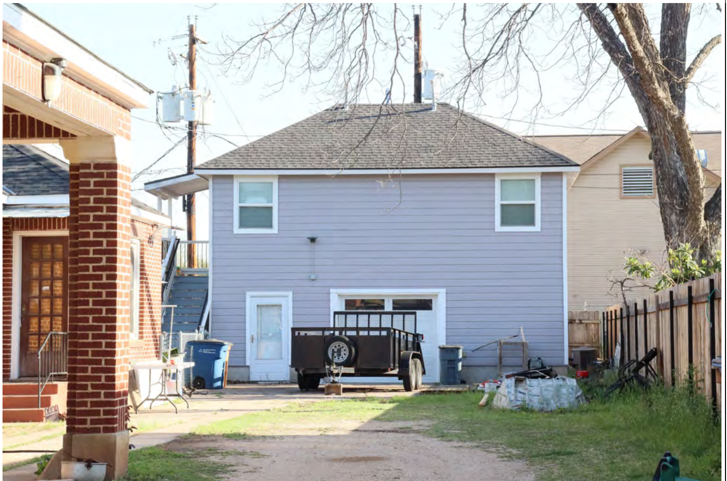
View facing north.
