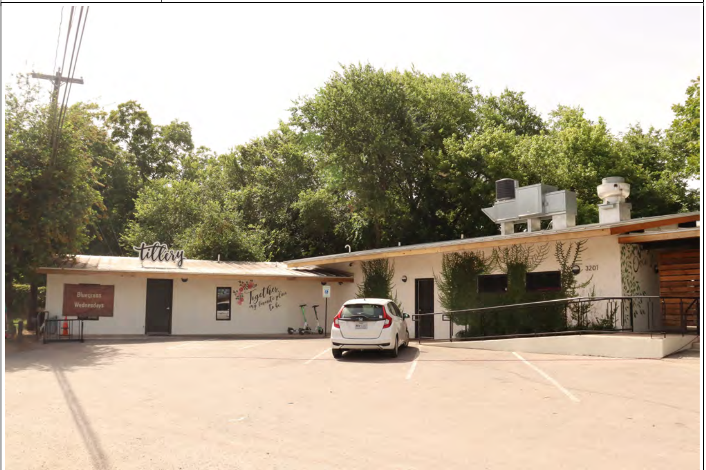
View facing southeast.
