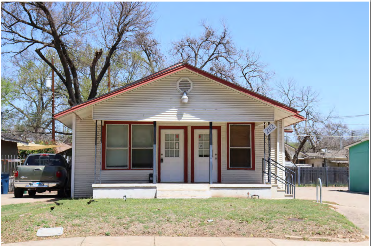
View facing north.
