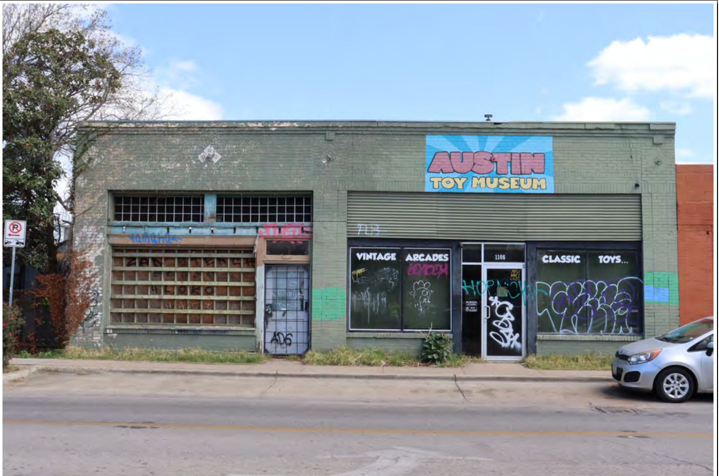
View facing north.
