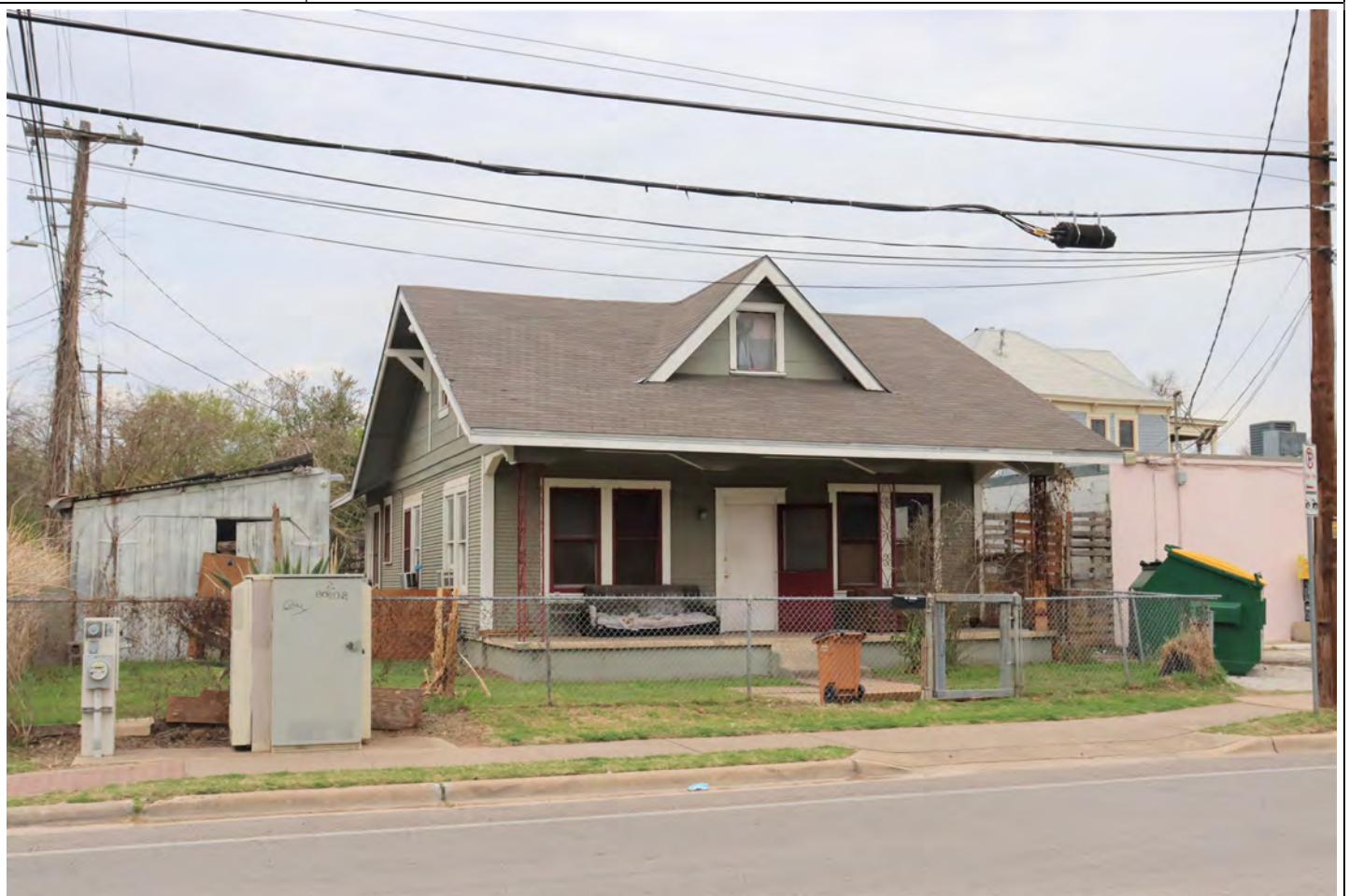
View facing north.
