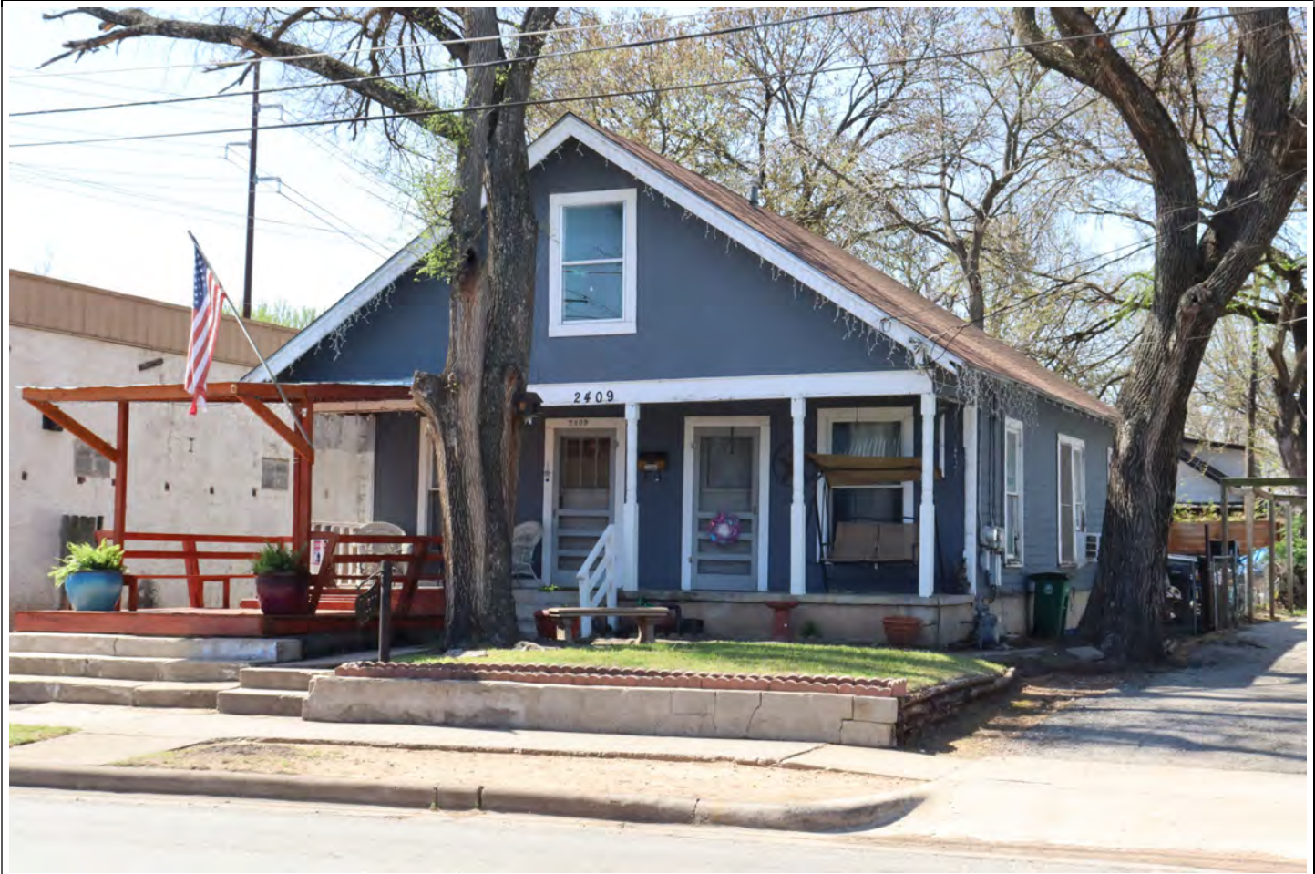
View facing southeast.
