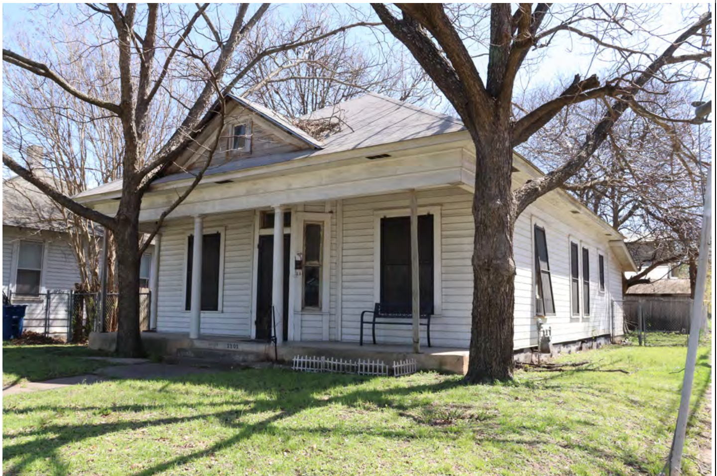
View facing southeast.
