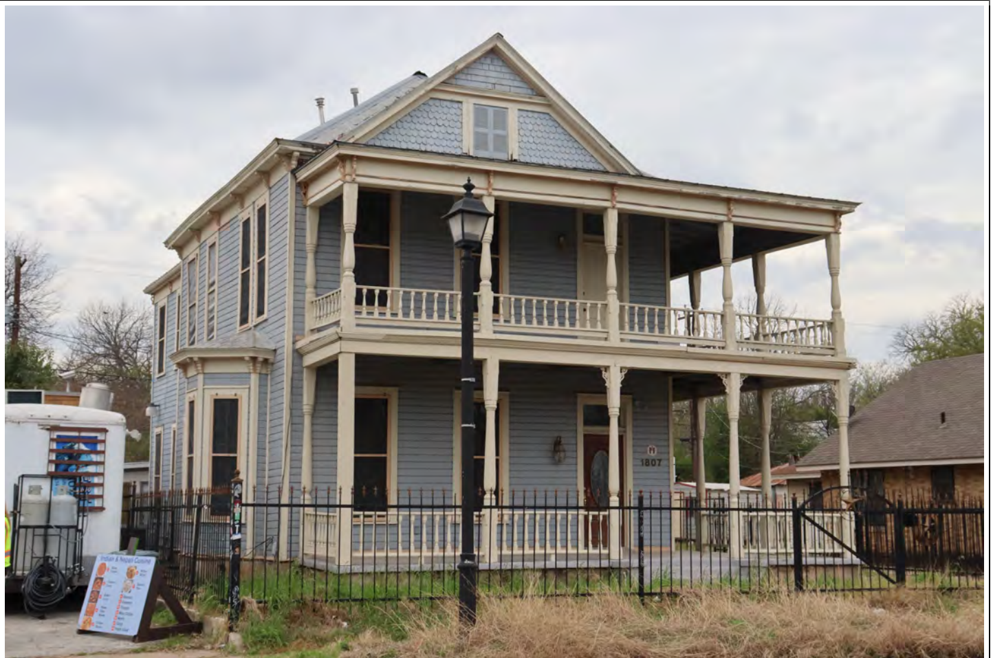
View facing southwest.
