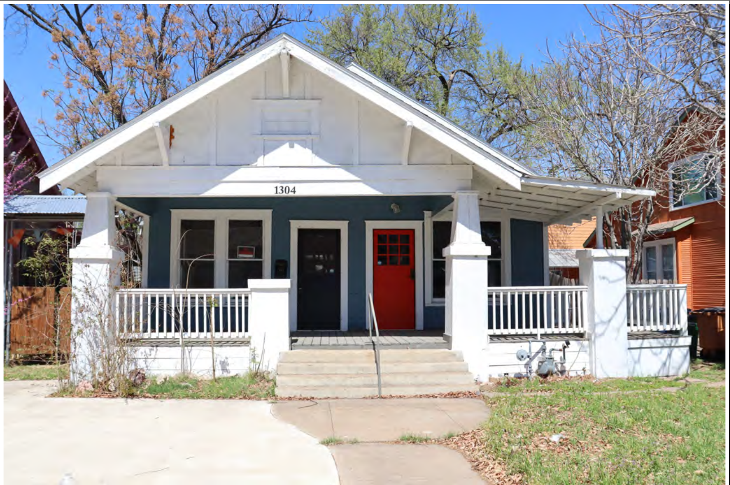
View facing north.
