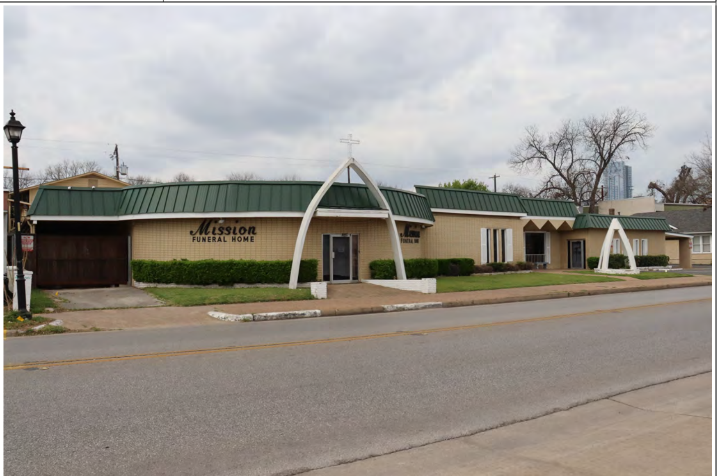
View facing southwest.
