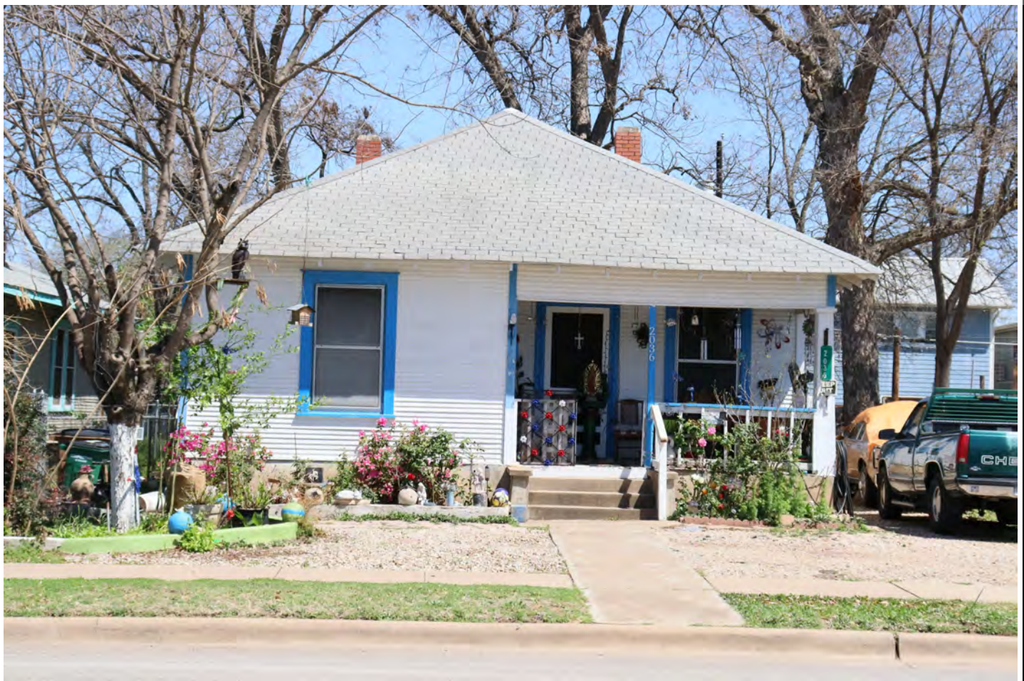
View facing north.
