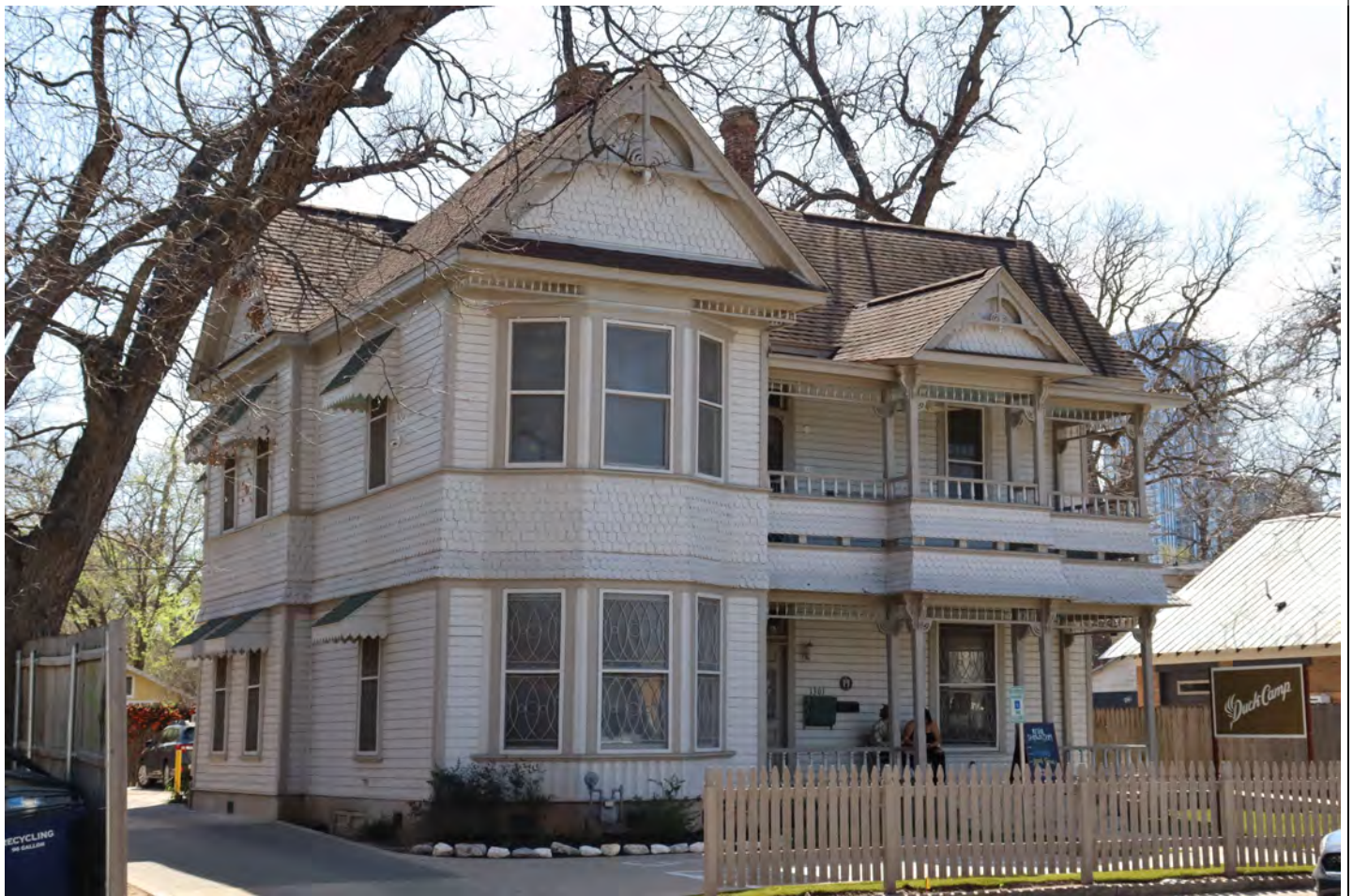
View facing southwest.
