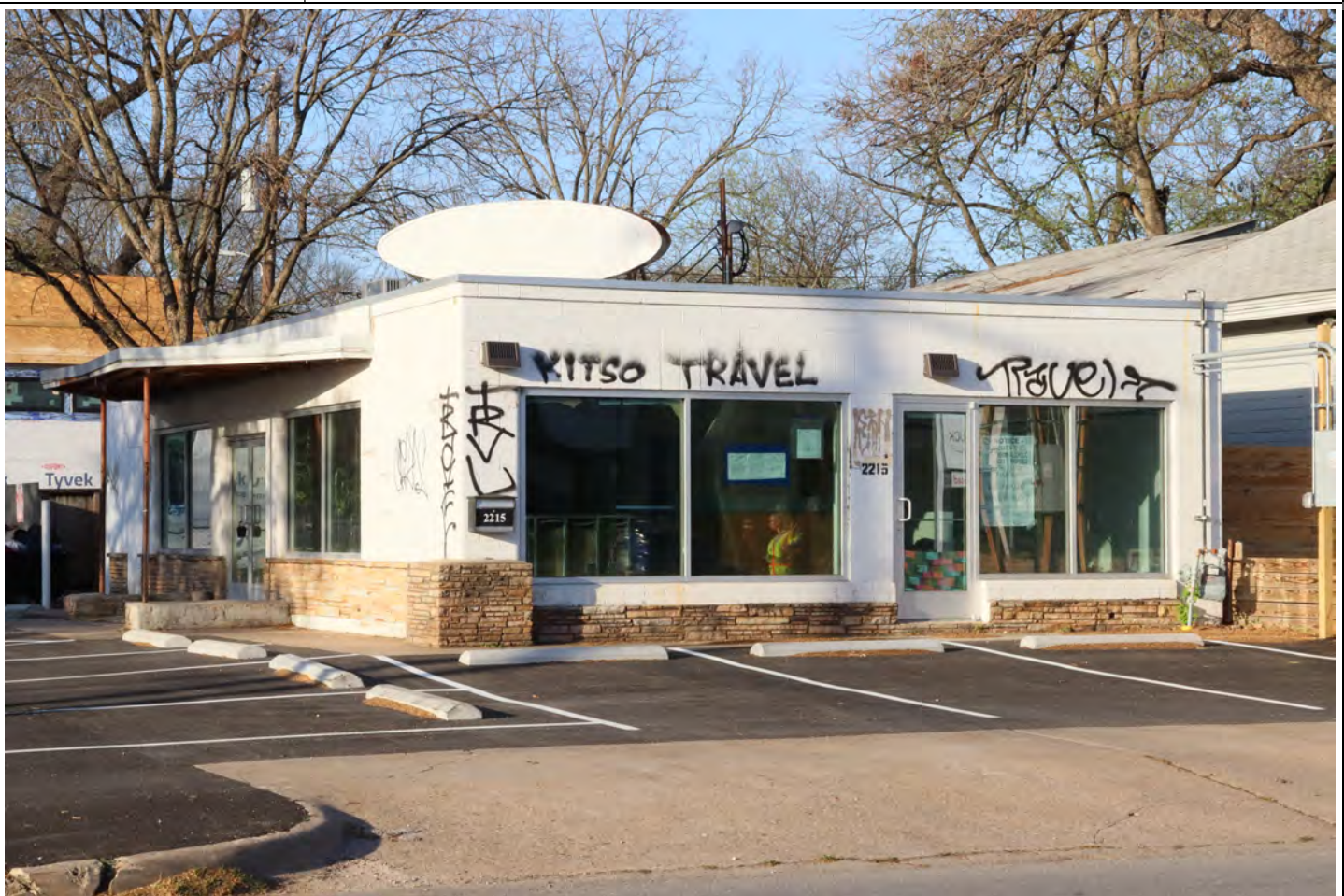
View facing southwest.
