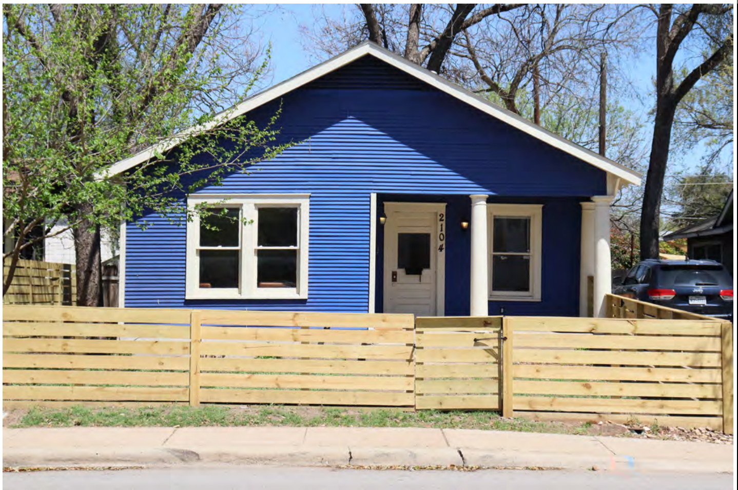
View facing north.
