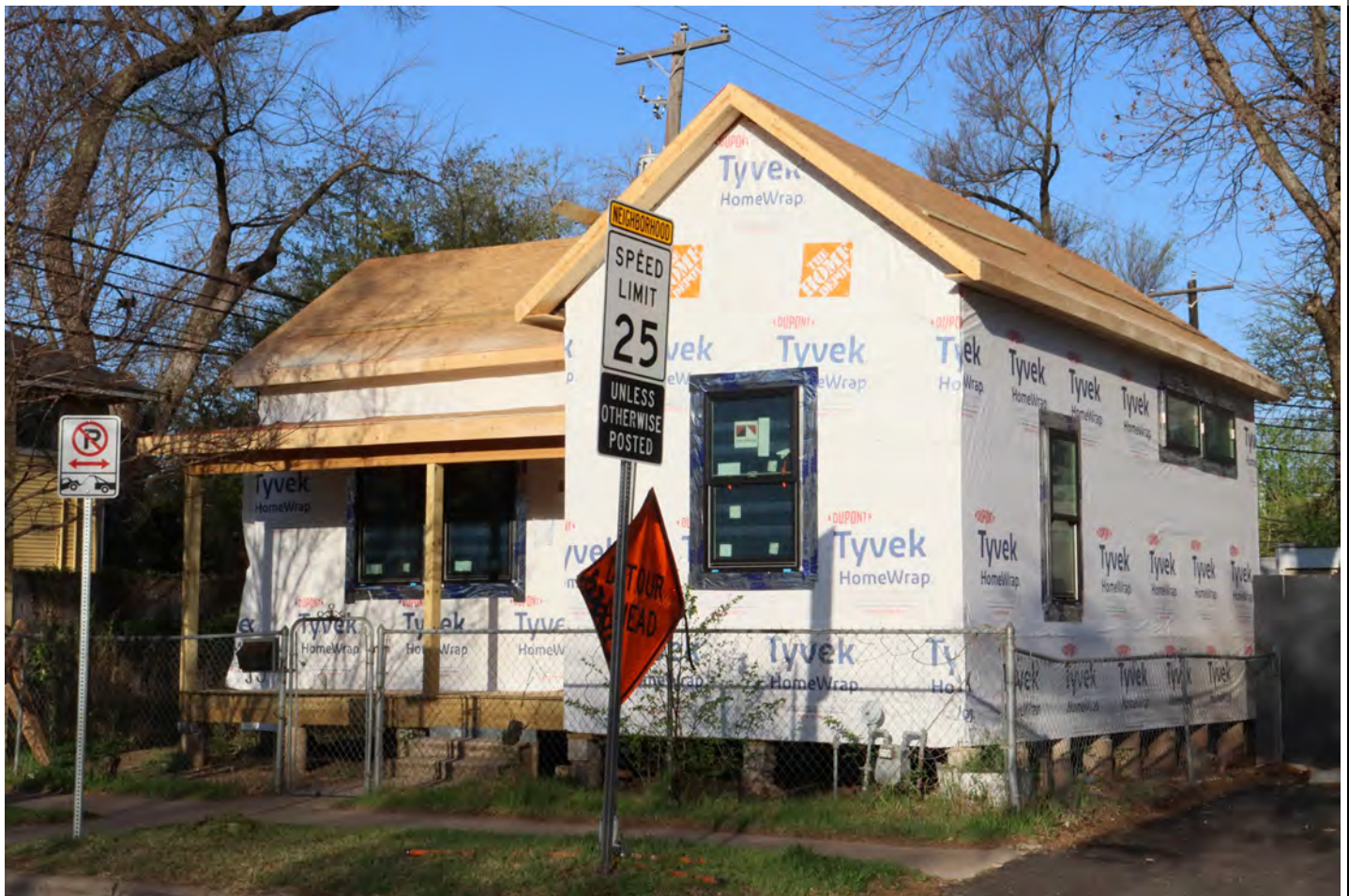
View facing southwest.
