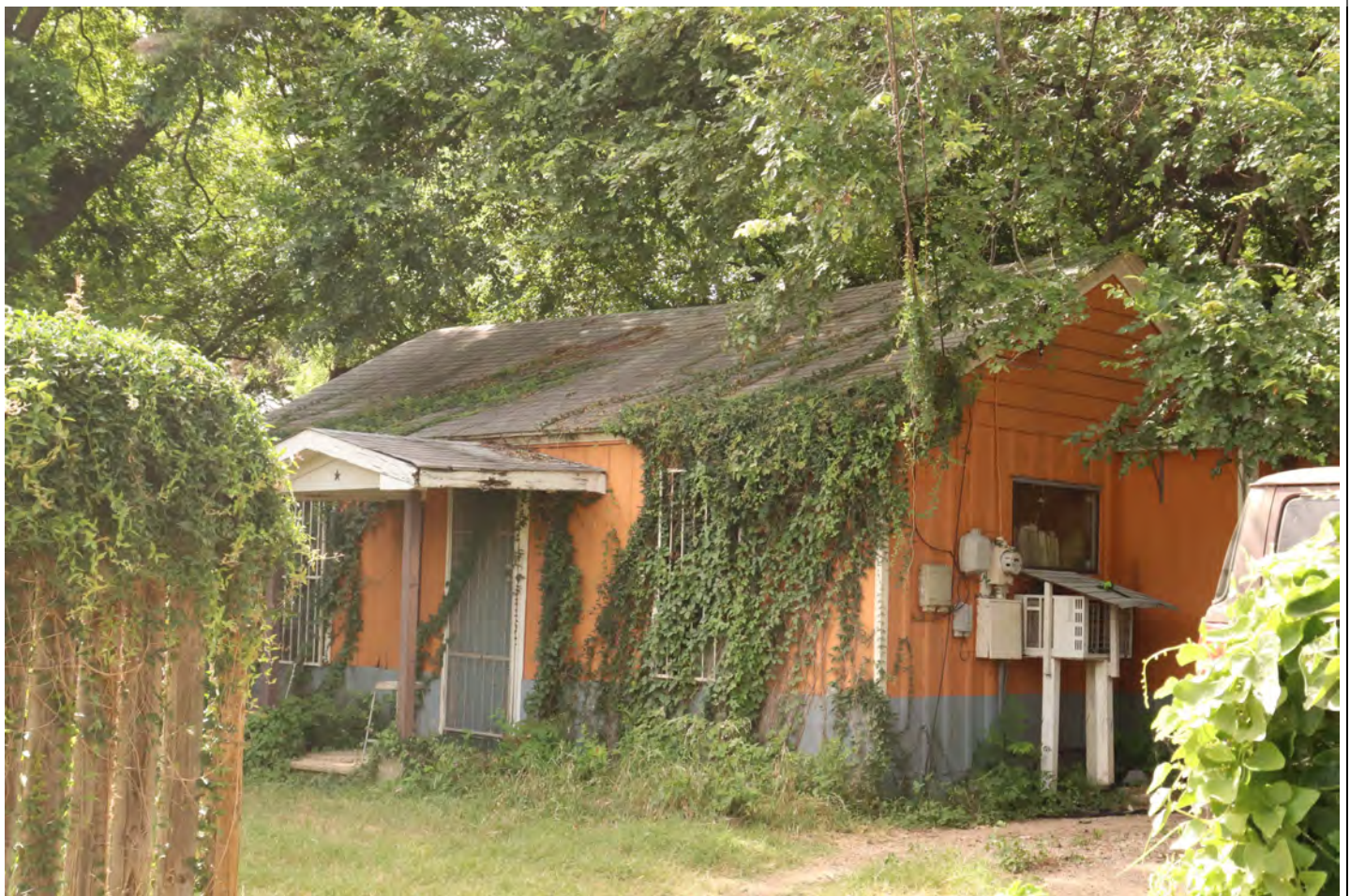
View facing southeast.
