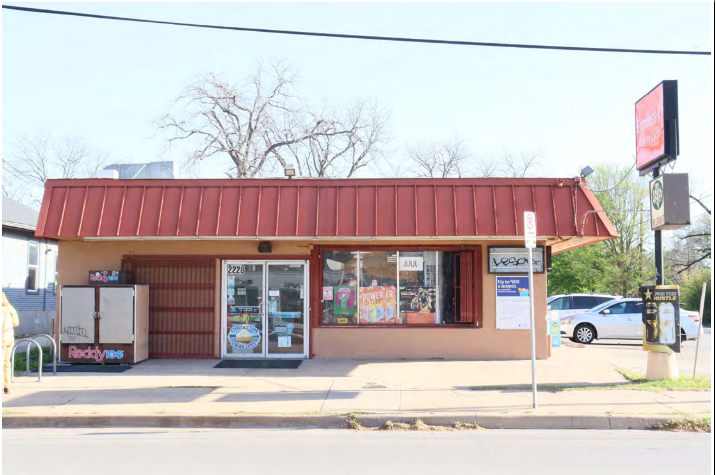
View facing north.
