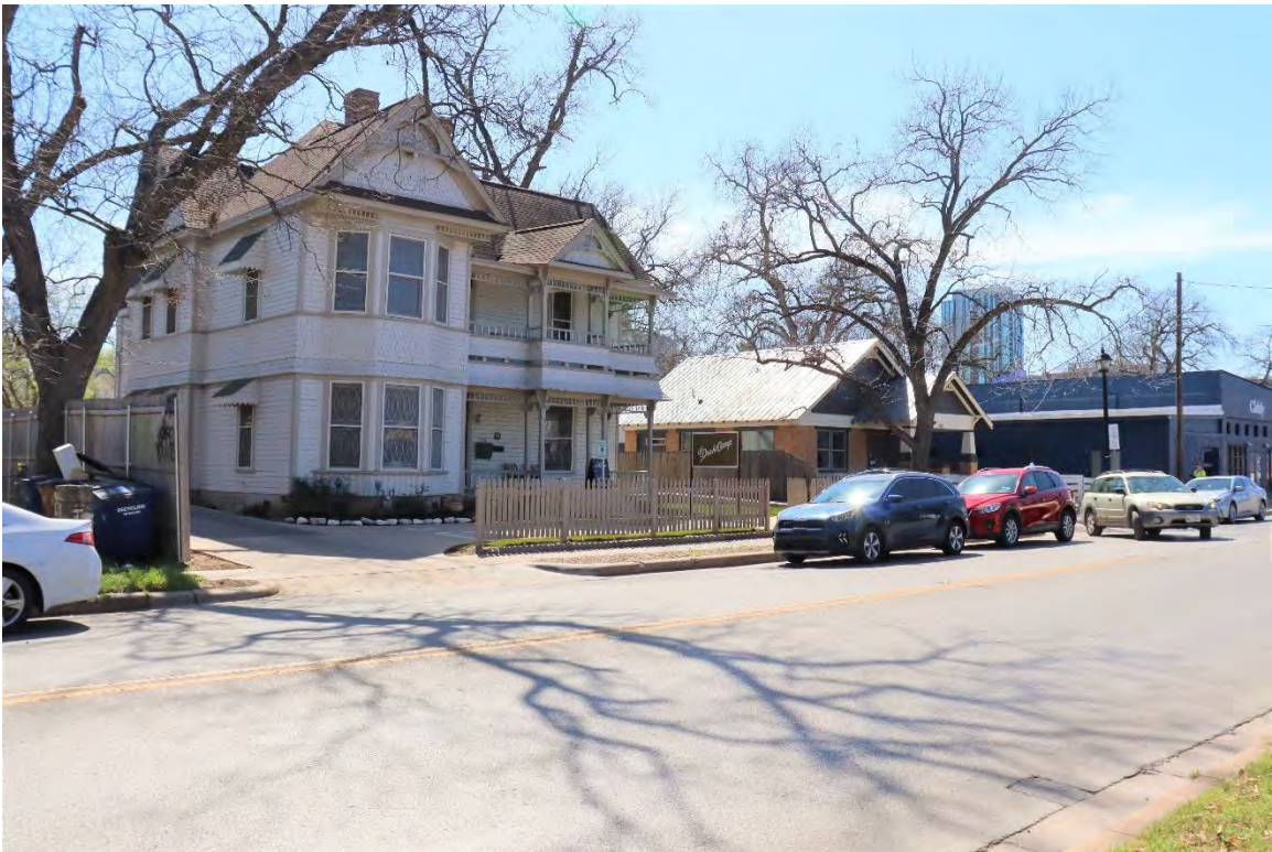
1300 block, view facing southwest. Resources 1026, 1019, and 1018 (left-right) visible.
