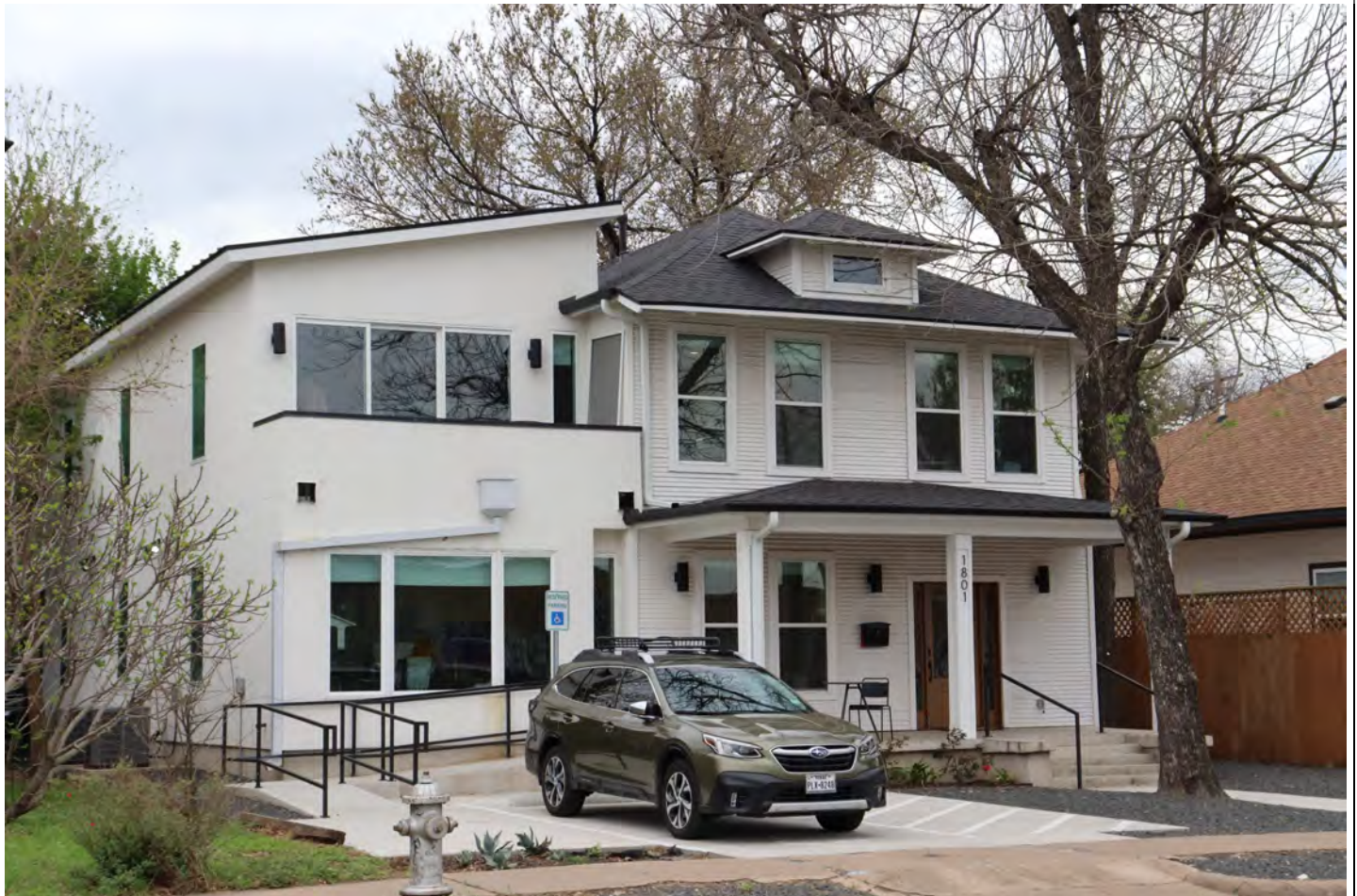
View facing southwest.
