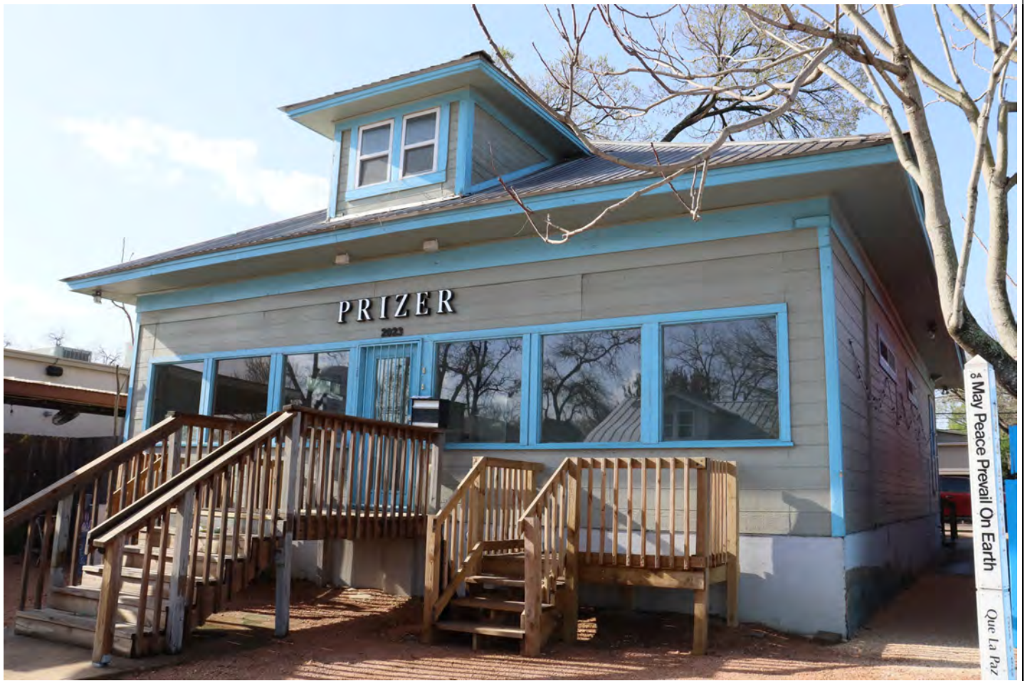
View facing southeast.
