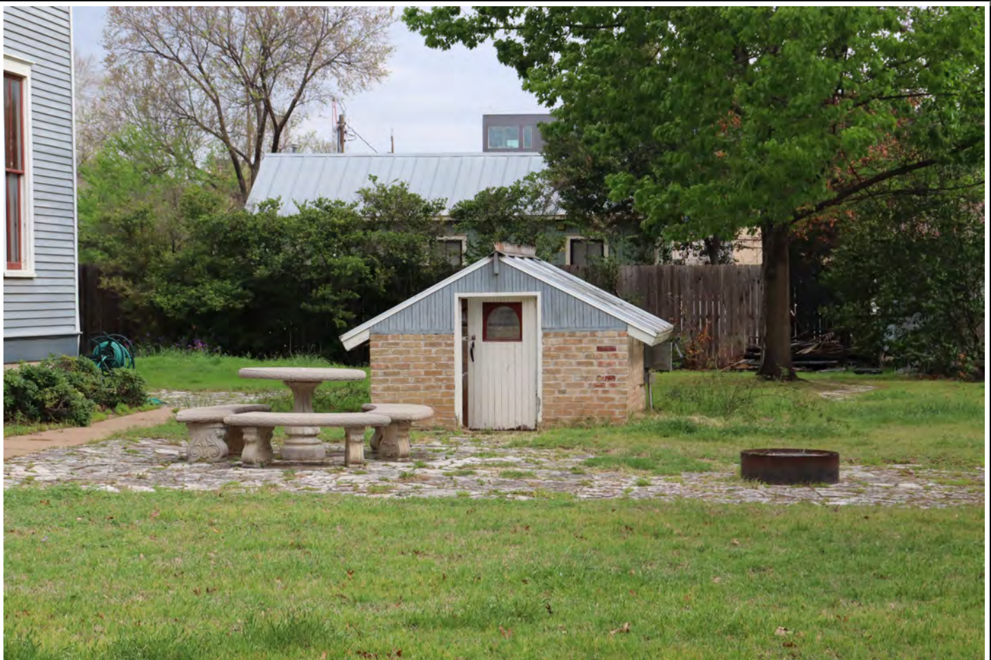
View facing northwest. Showing relationship between 1041A (left) and 1041D (right).
