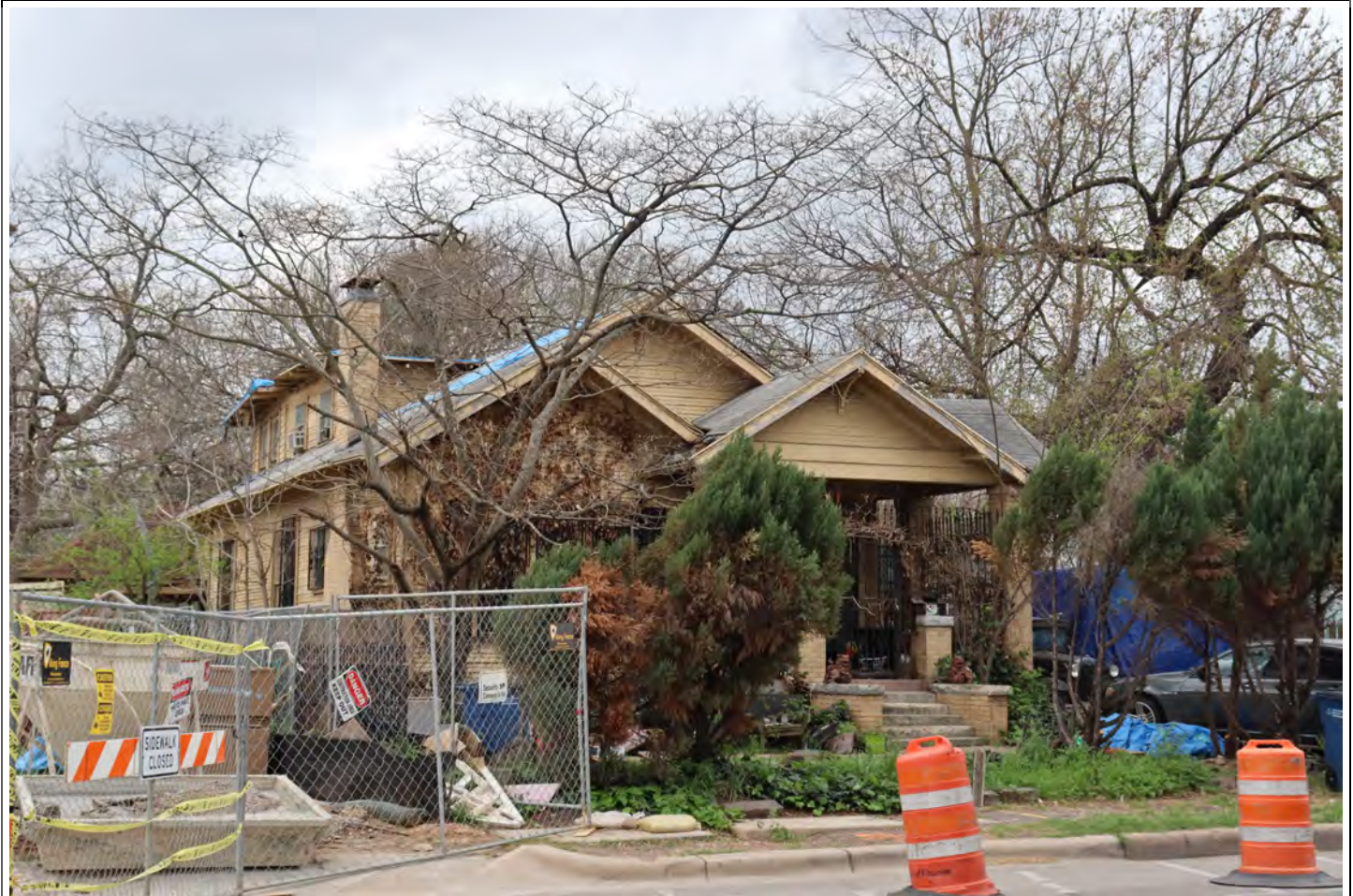
View facing southwest.
