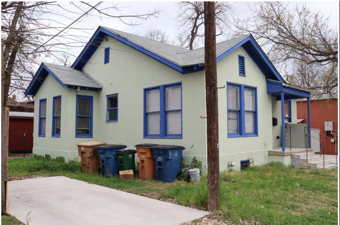
View facing north.
