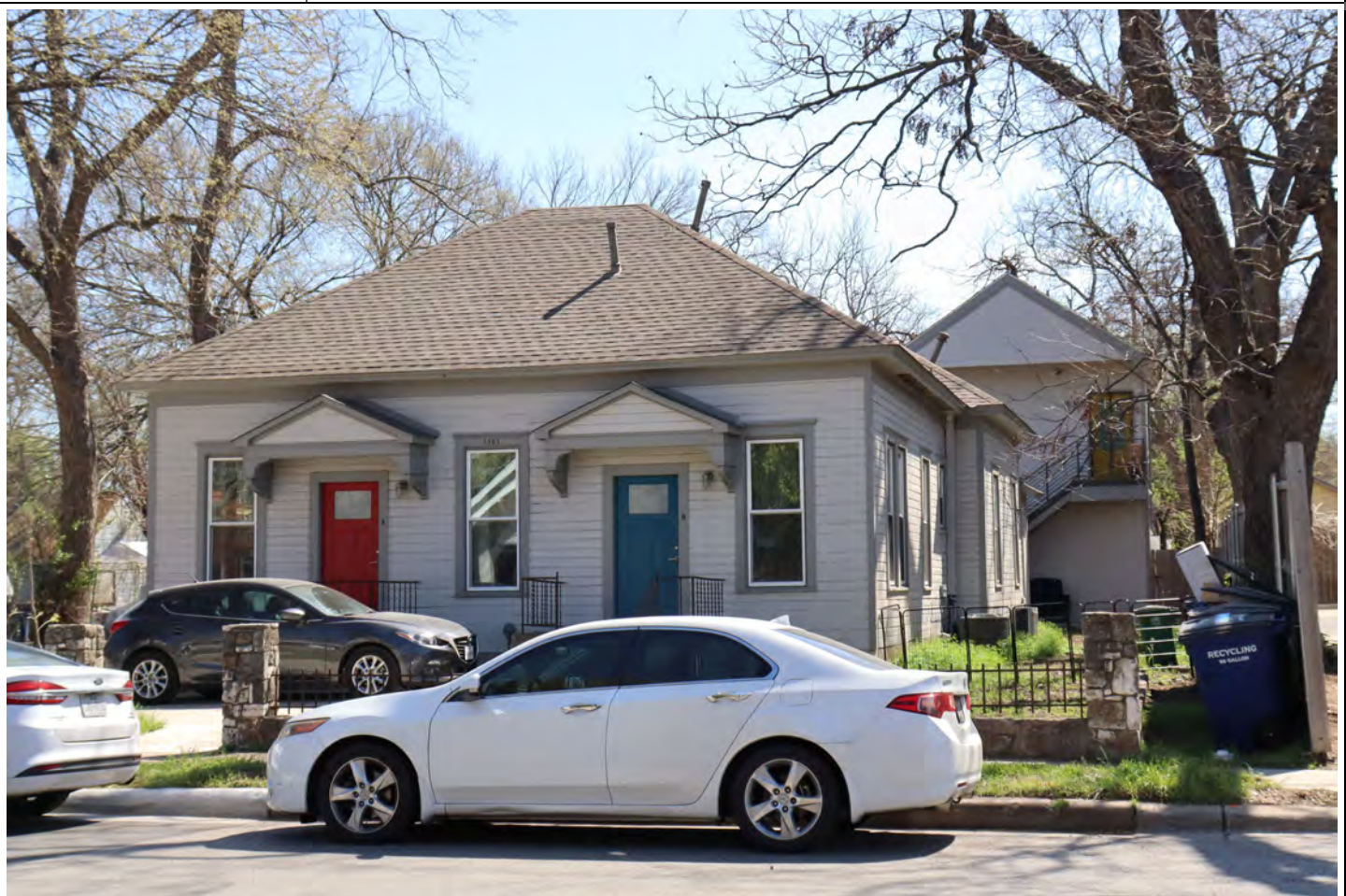
View facing southeast.
