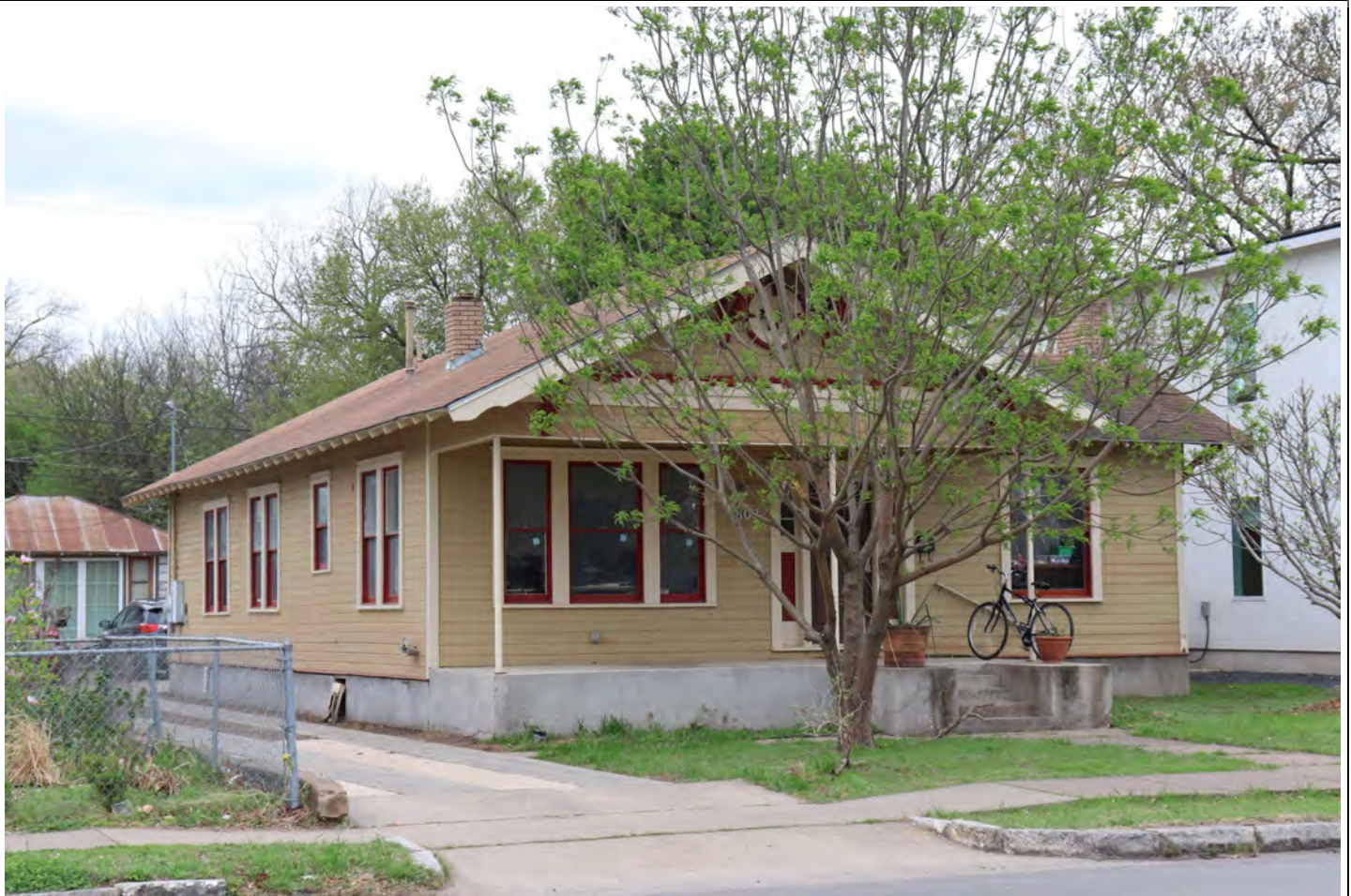
View facing southwest.
