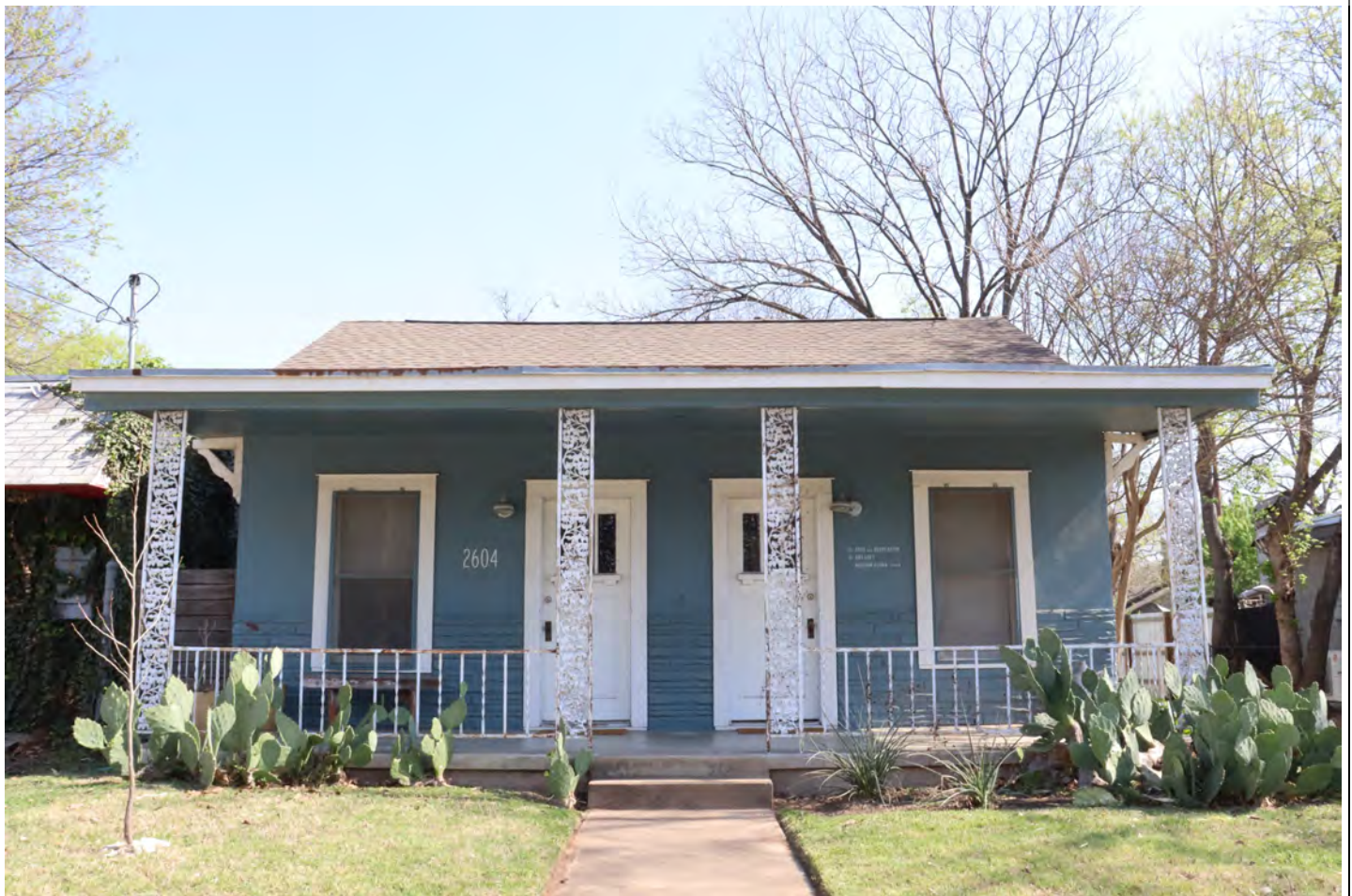
View facing north.
