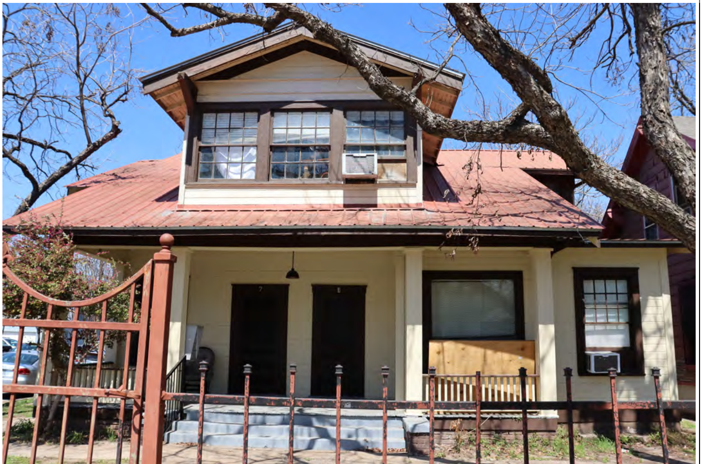
View facing north.
