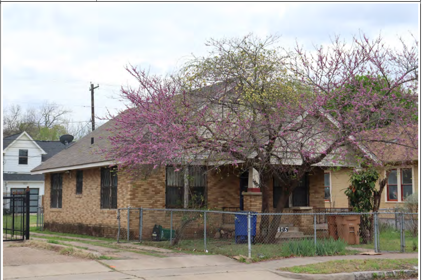
View facing southwest.
