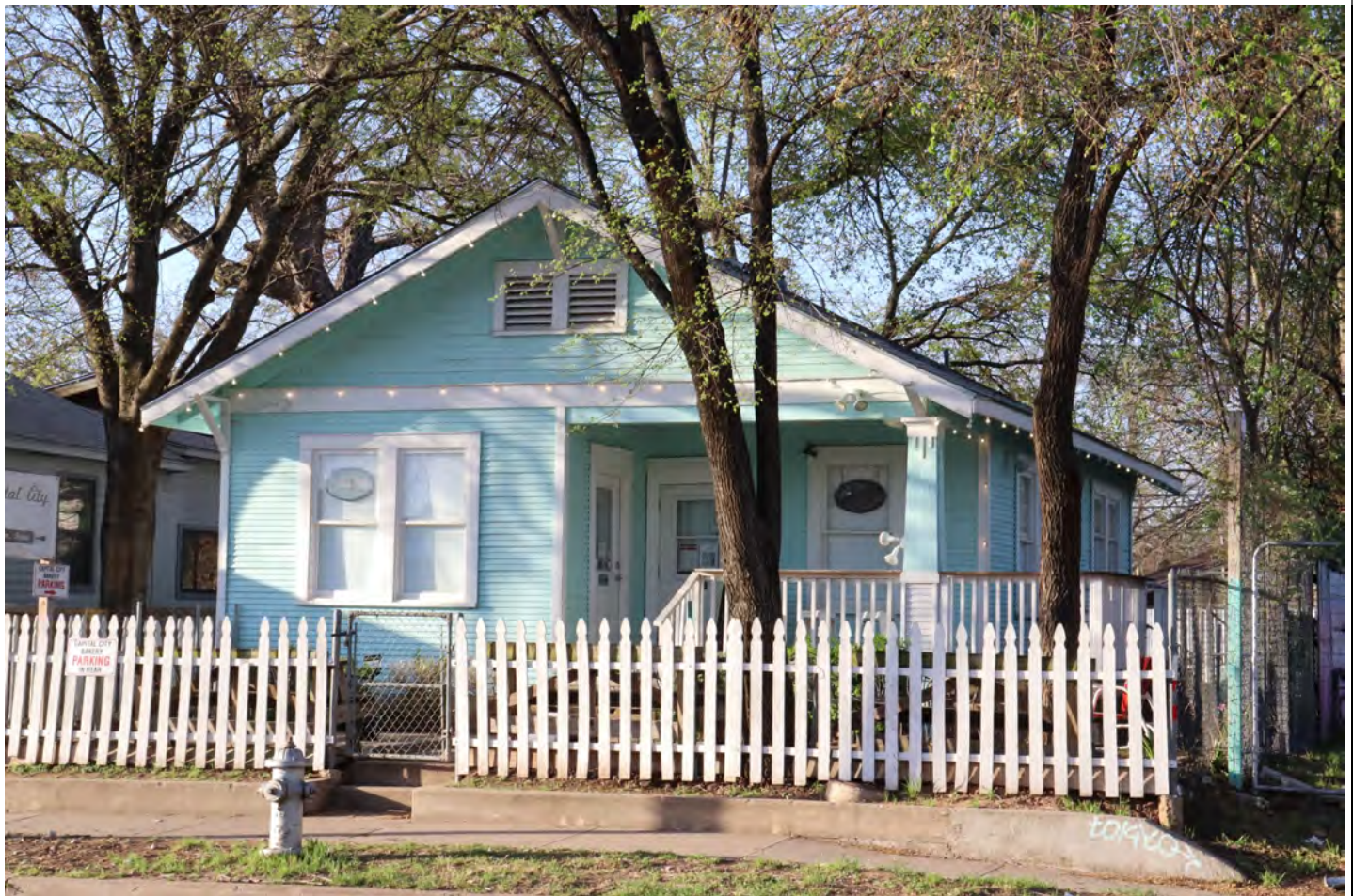
View facing southeast.
