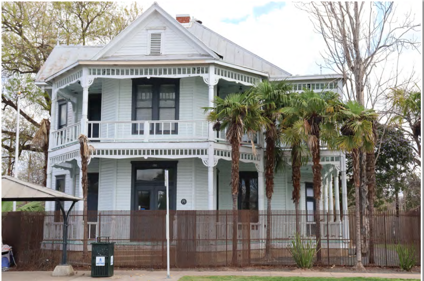
View facing north.
