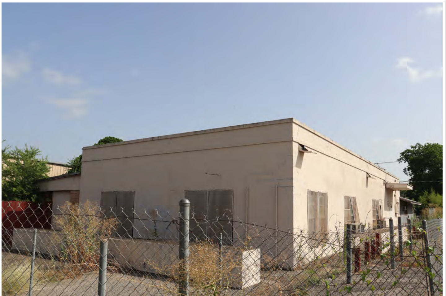
View facing northwest. Showing facade and east elevation.
