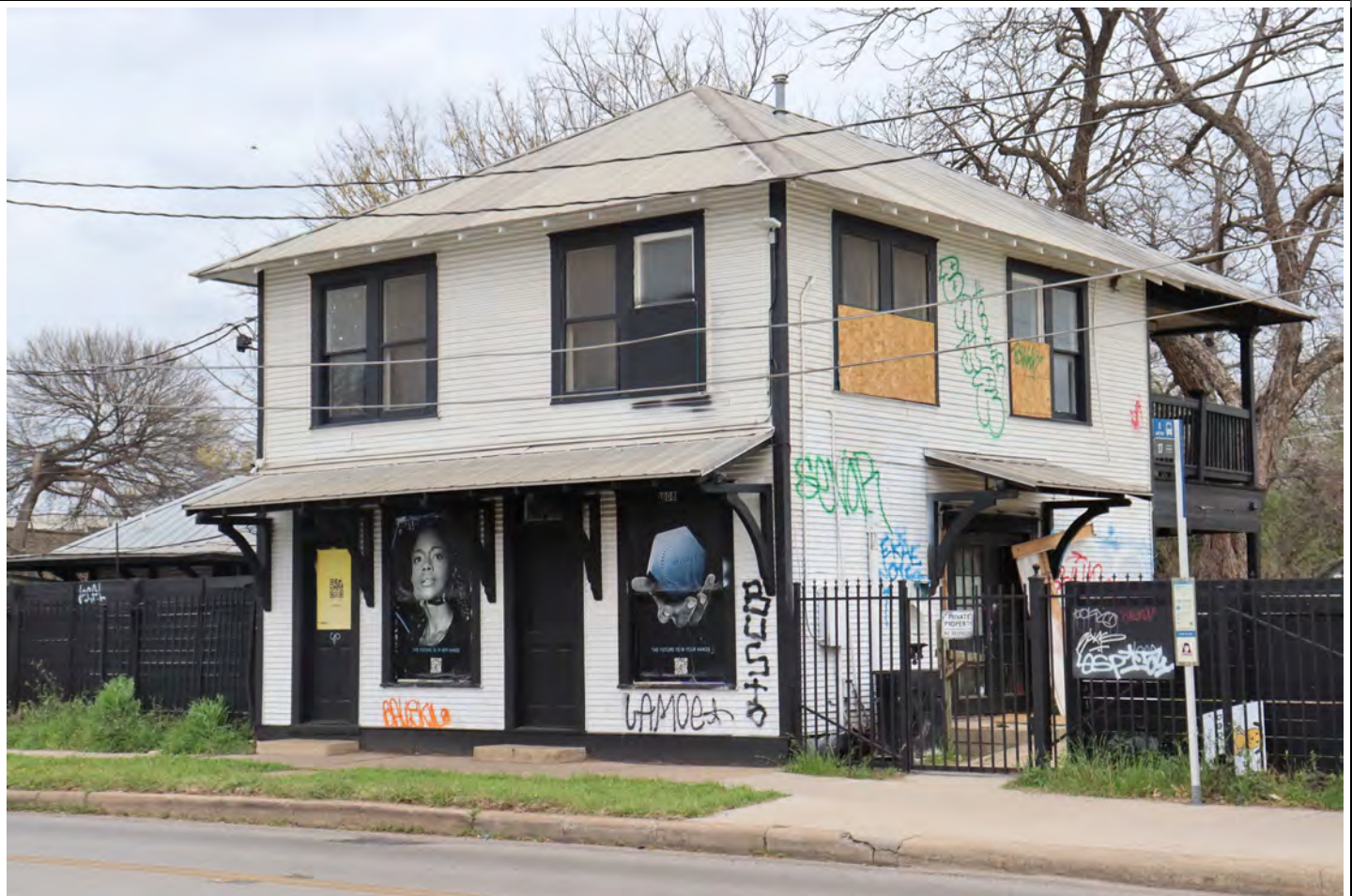
View facing north.
