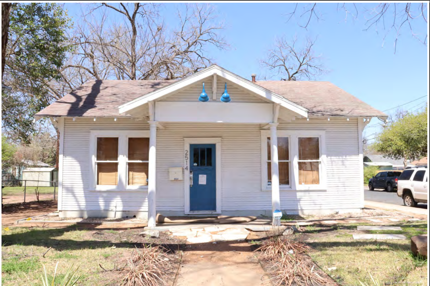
View facing north.
