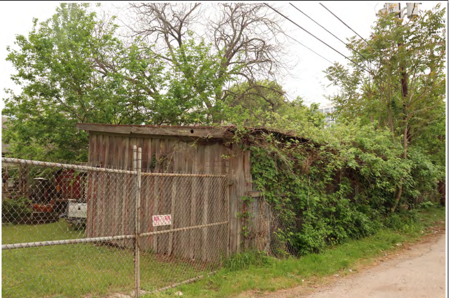
View facing southwest.
