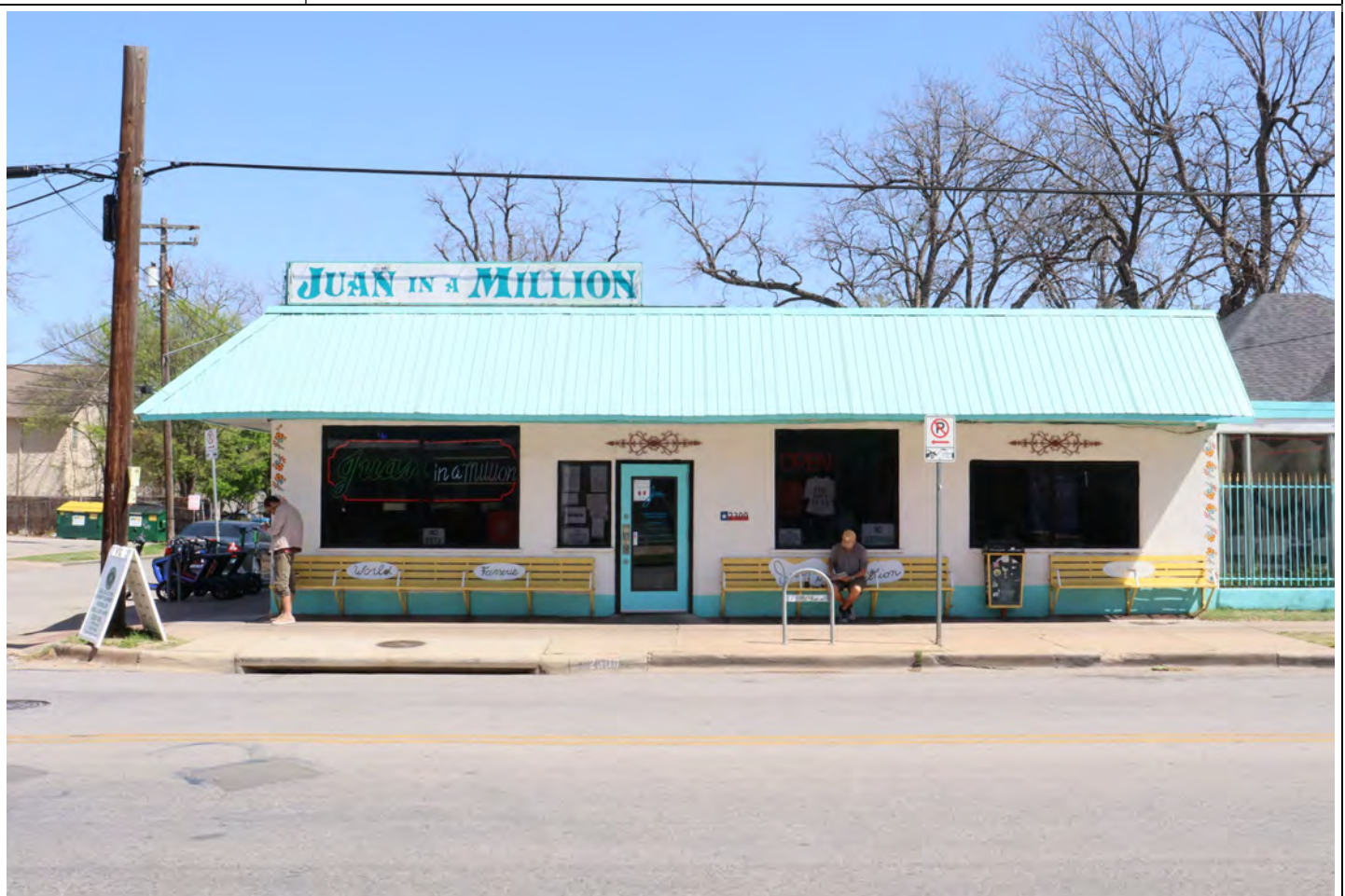
View facing north.
