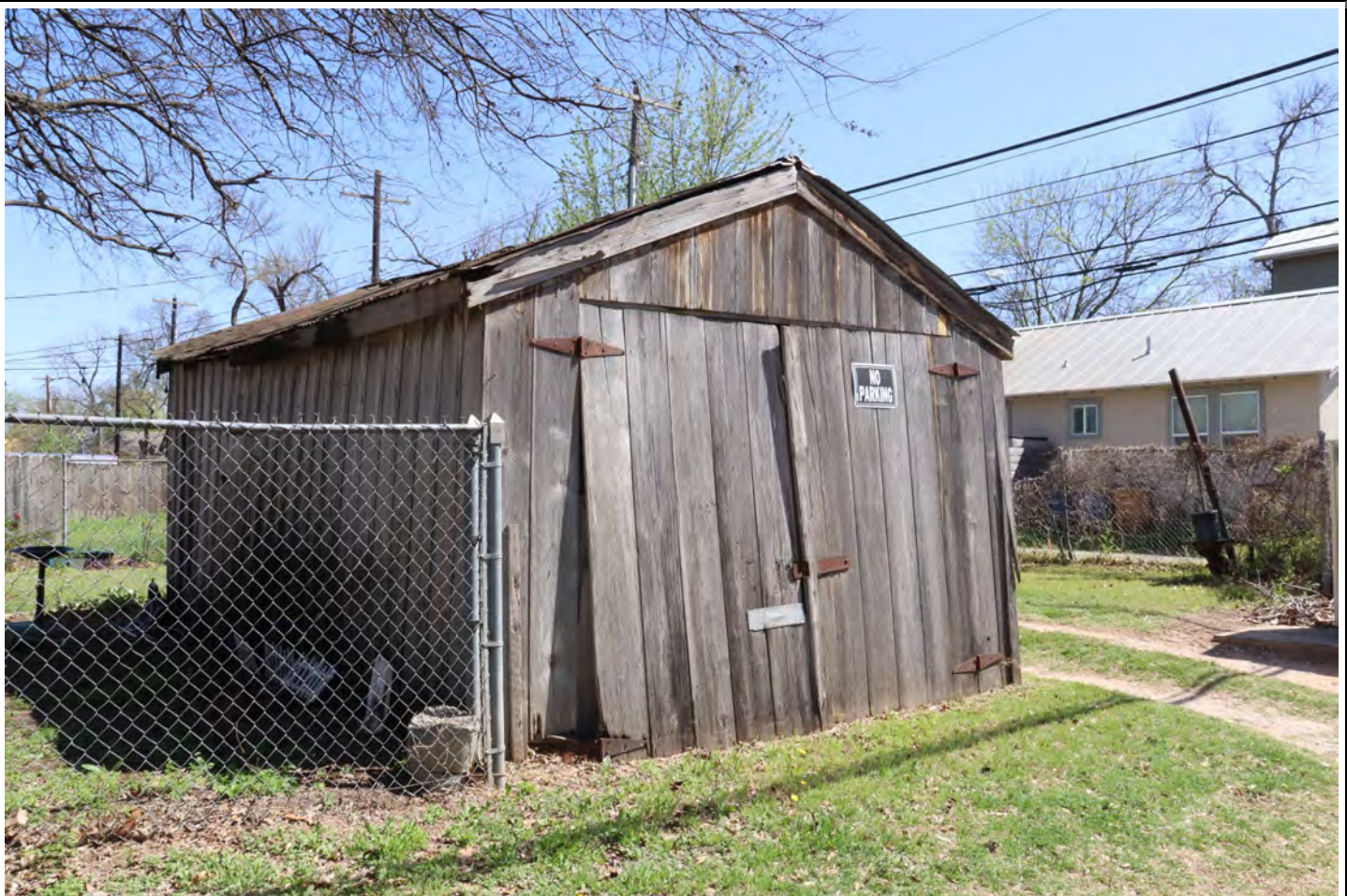
View facing southeast.
