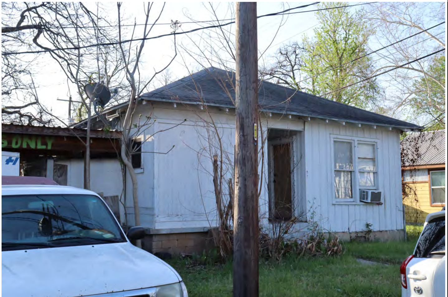
View facing southeast.
