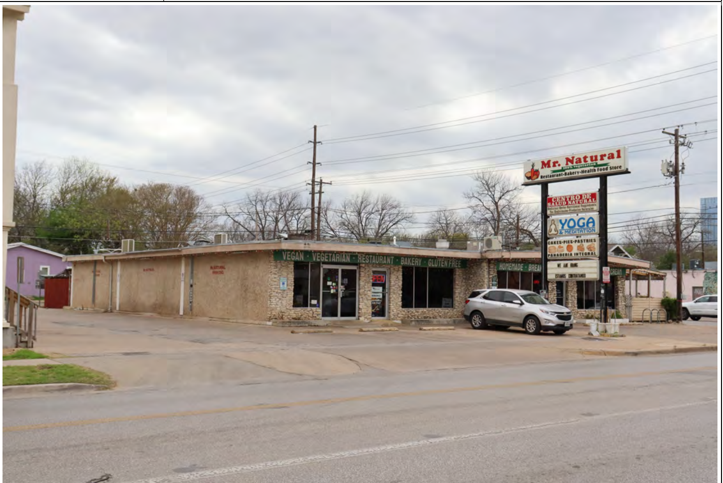
View facing southwest.
