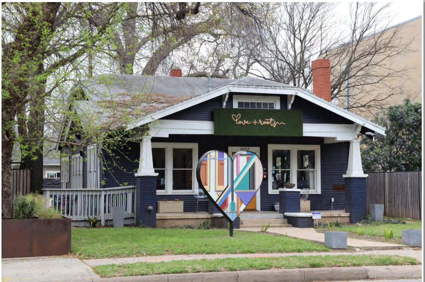
View facing southwest.
