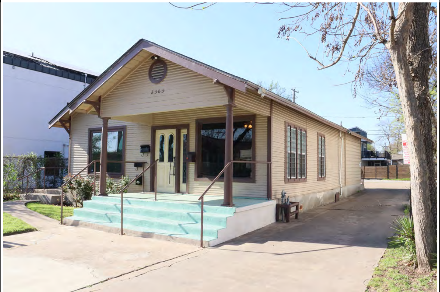
View facing southeast.
