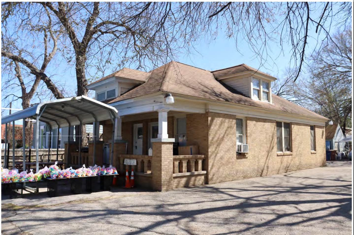
View facing southeast.
