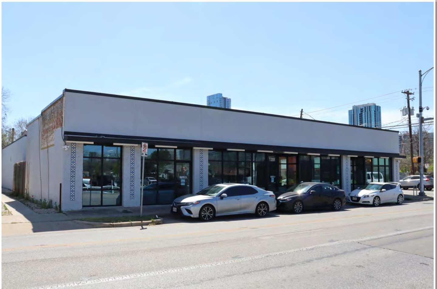
View facing southwest.
