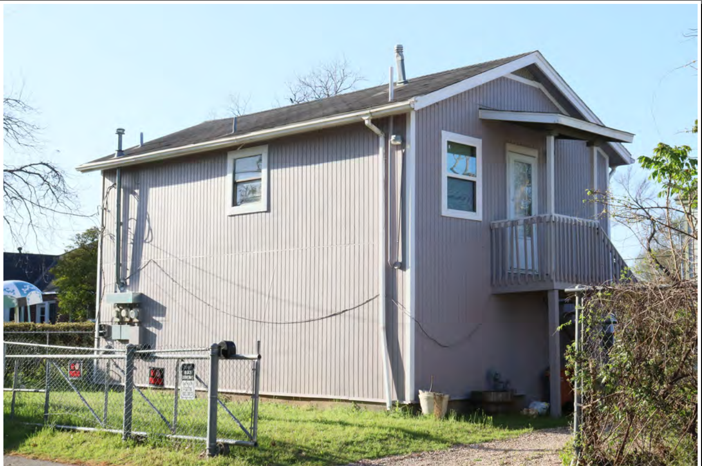
View facing southeast.
