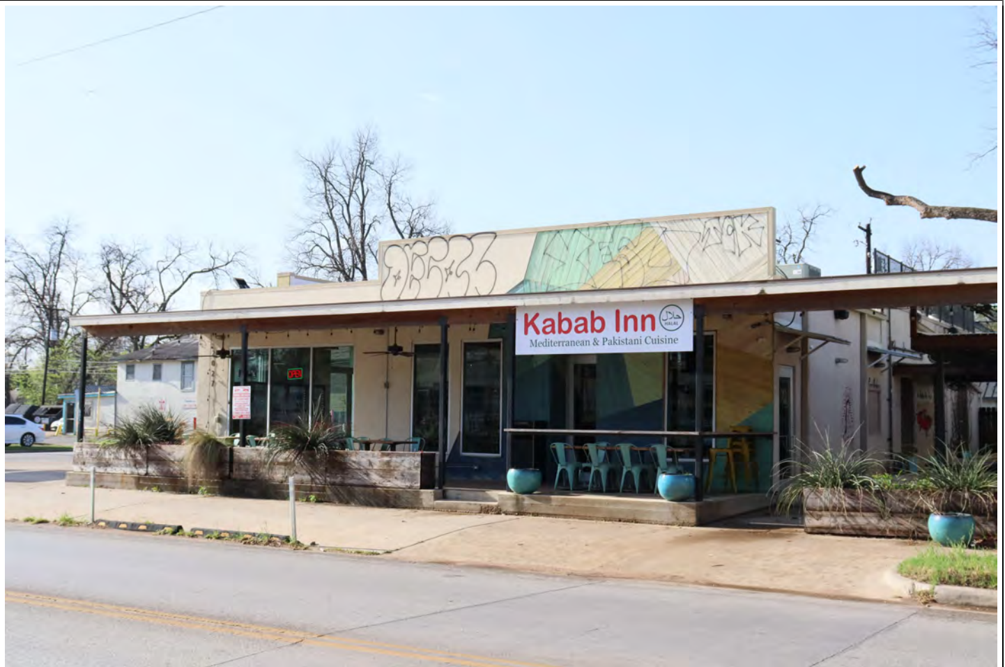
View facing southeast.
