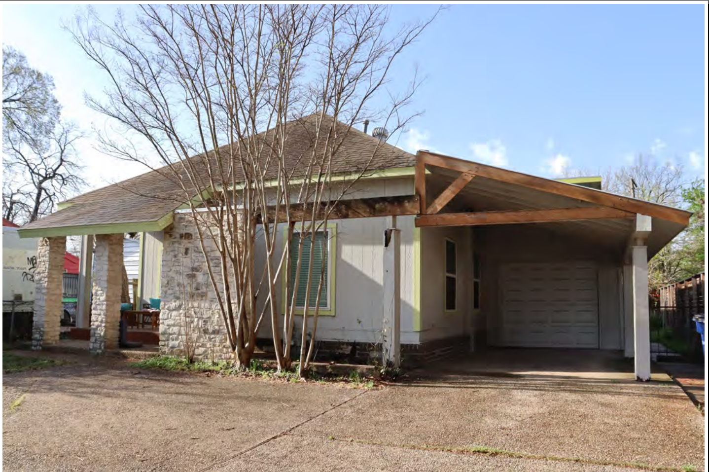
View facing southeast.
