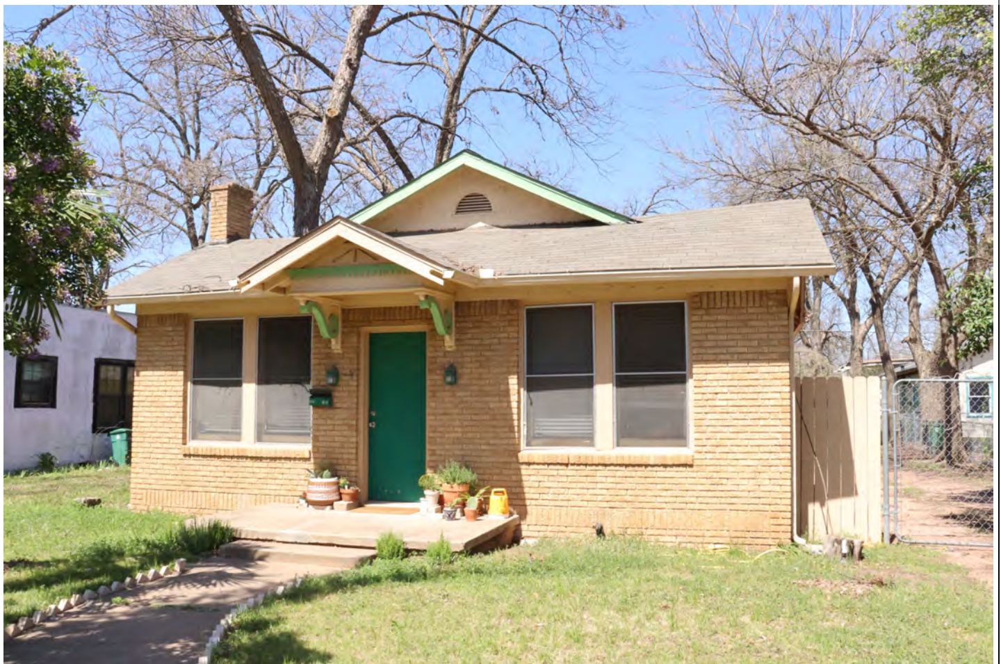
View facing north.
