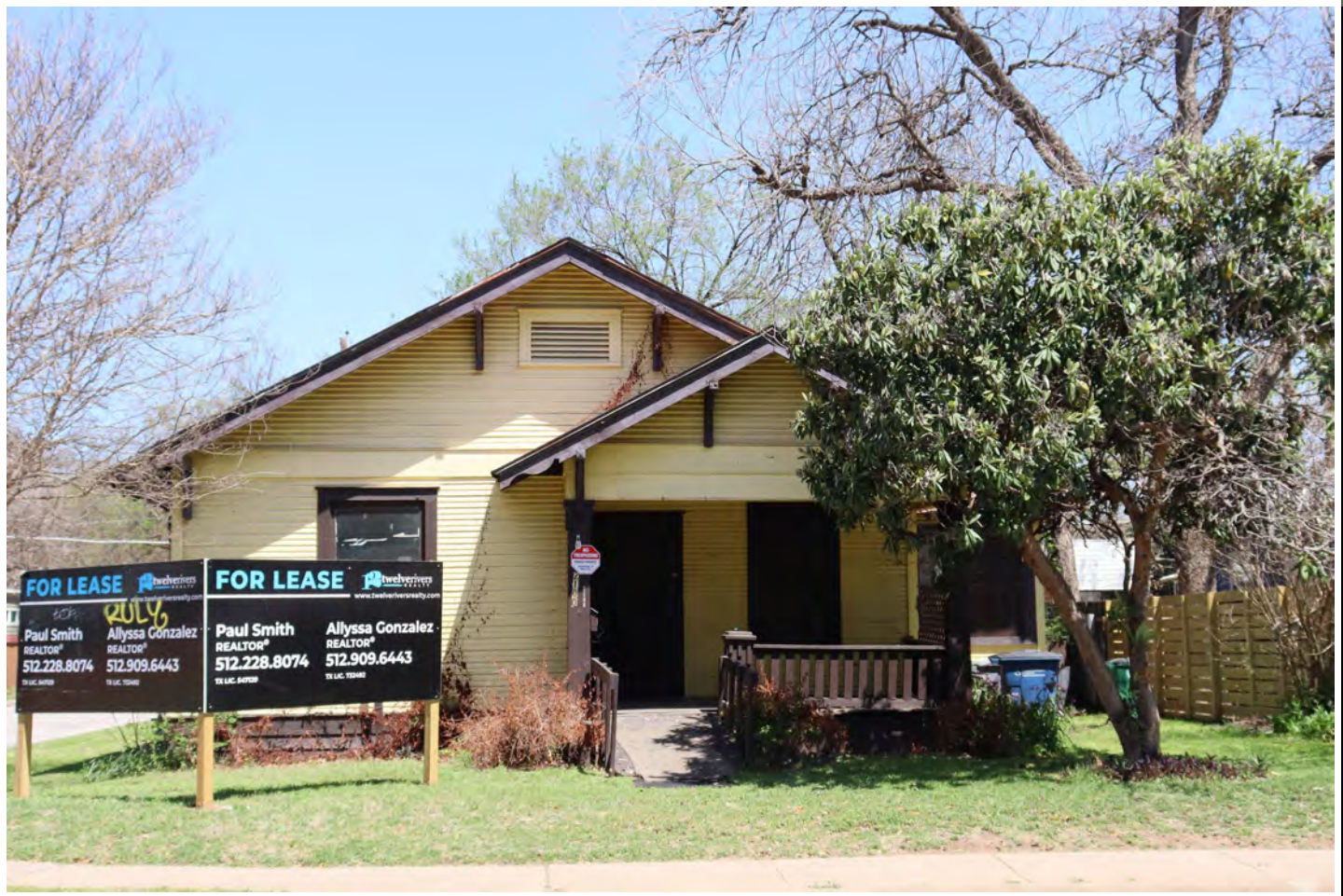
View facing north.
