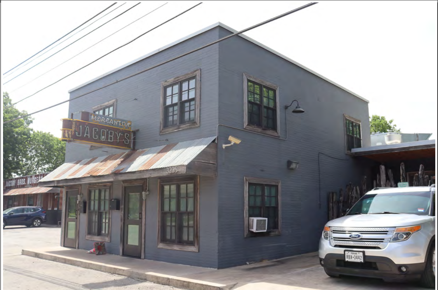
View facing southeast.
