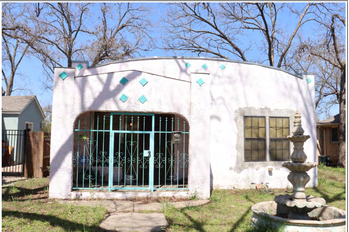
View facing north.
