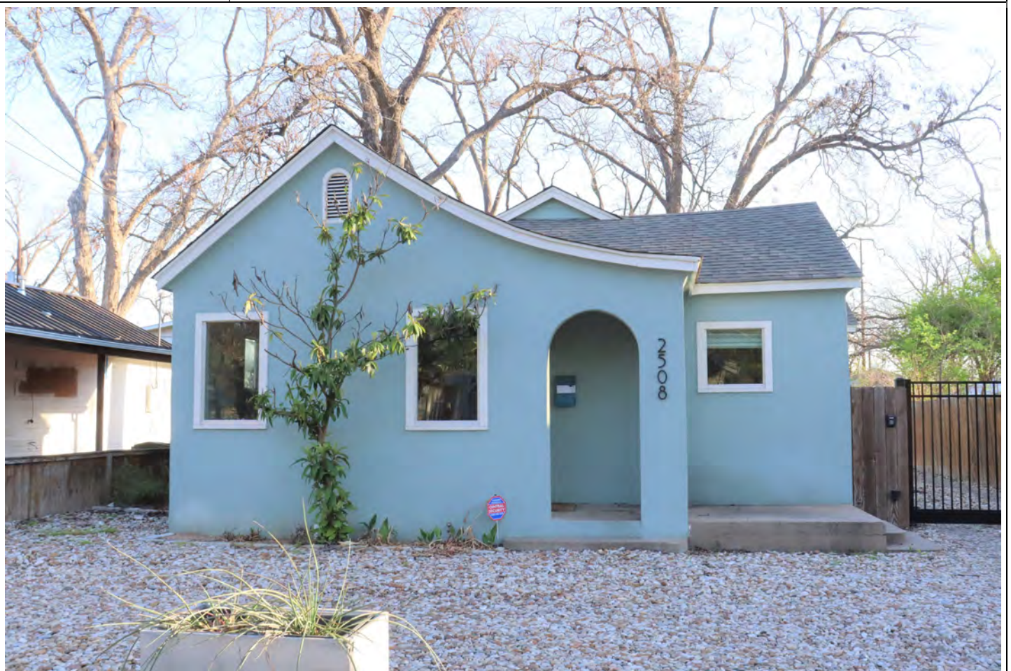
View facing north.
