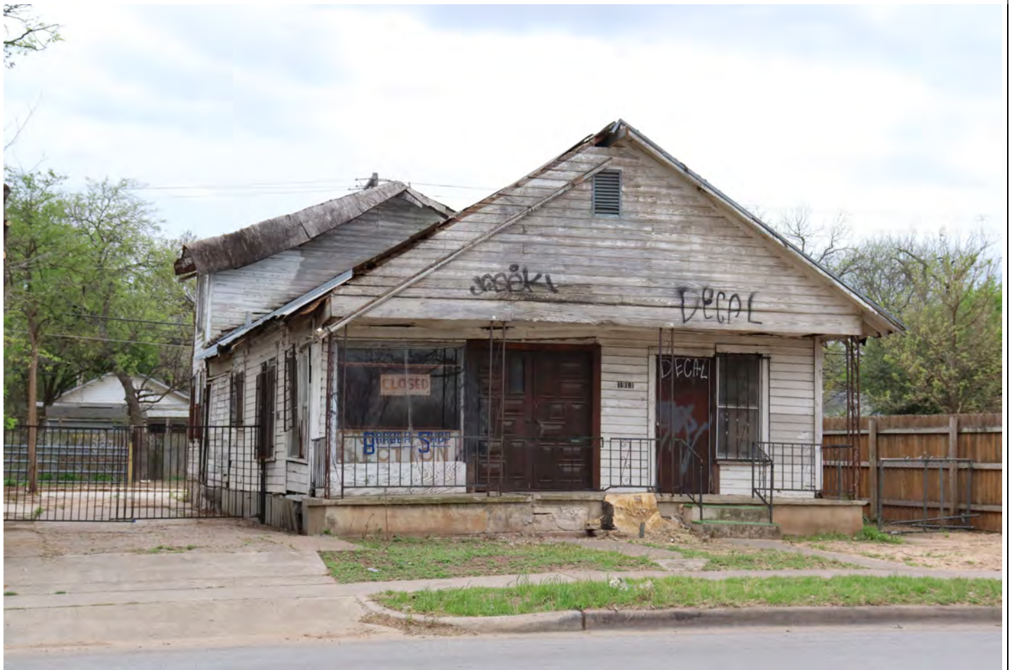
View facing southwest.
