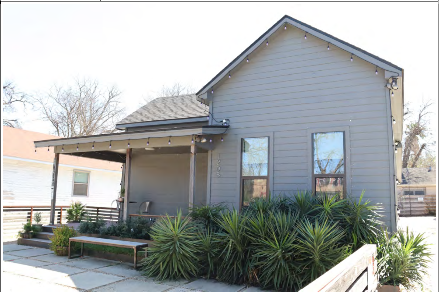
View facing southeast.
