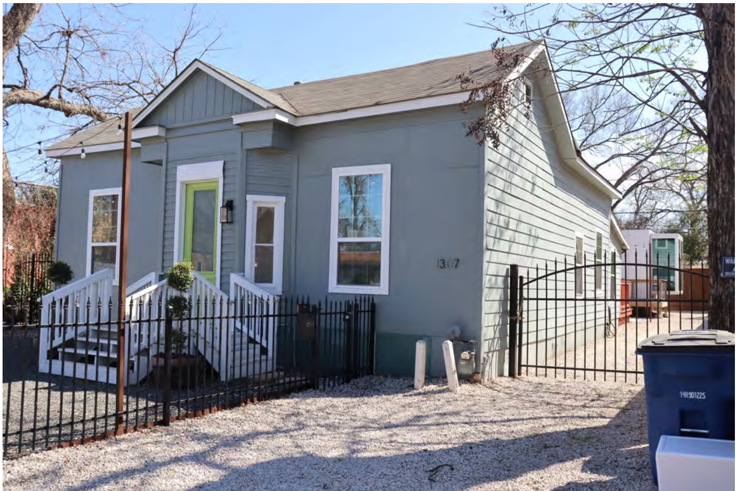
View facing southeast.
