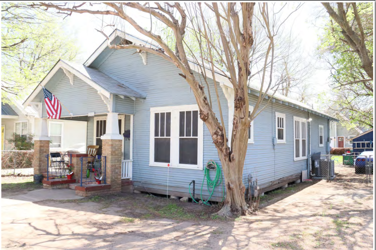
View facing southeast. Showing relationship between 1131A (left) and 1131B (back and right).
