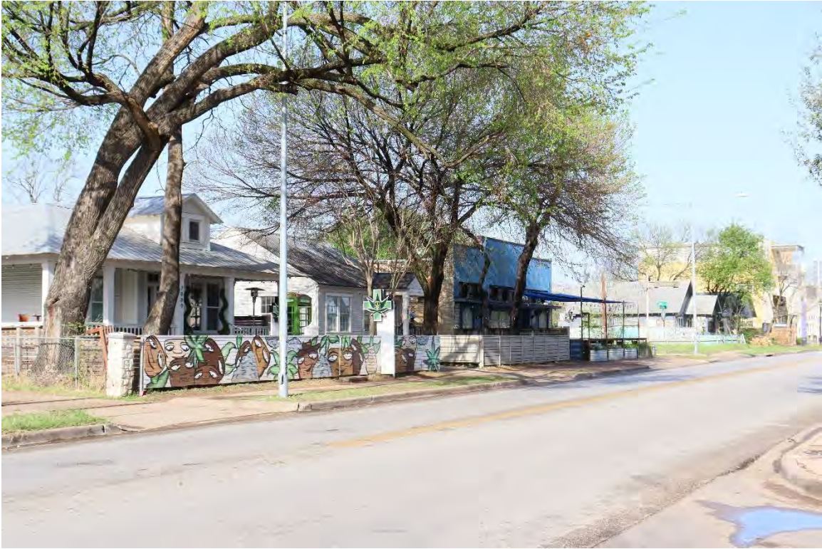
2000 block, view facing southwest. Resources 1070-1072 (right to left) visible.
