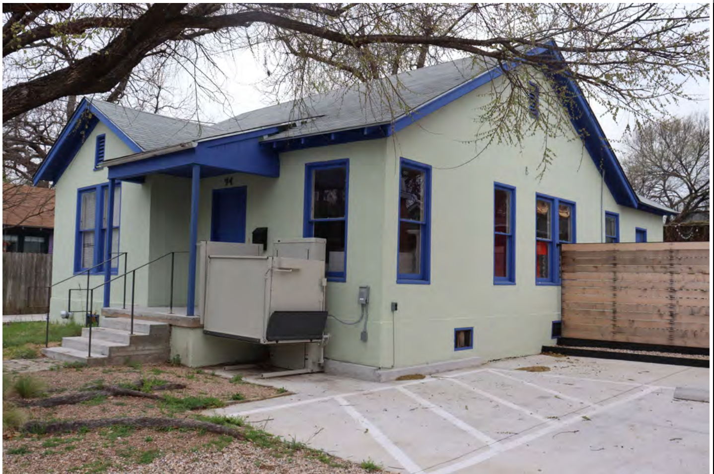
View facing southwest.
