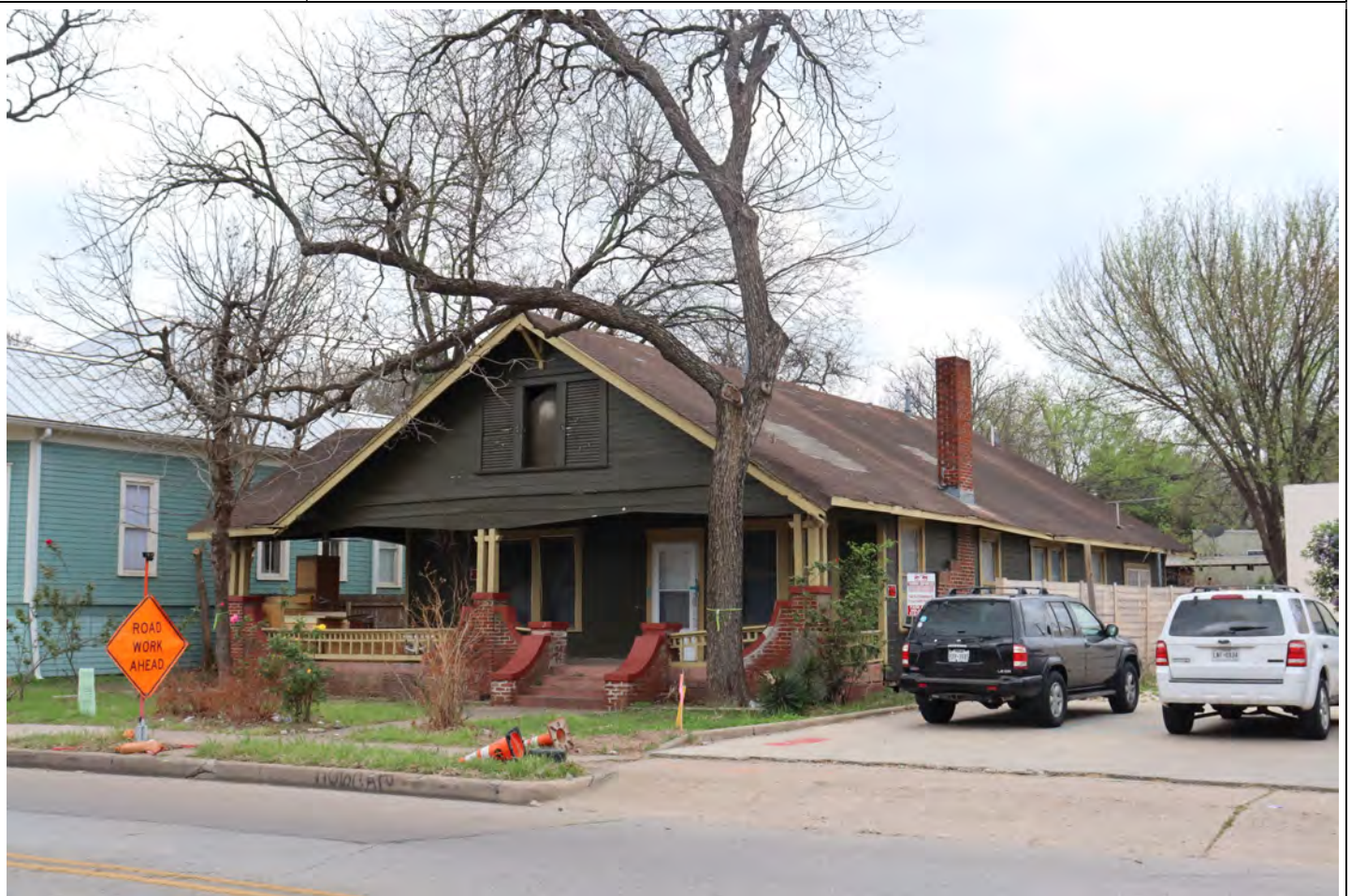
View facing southeast.
