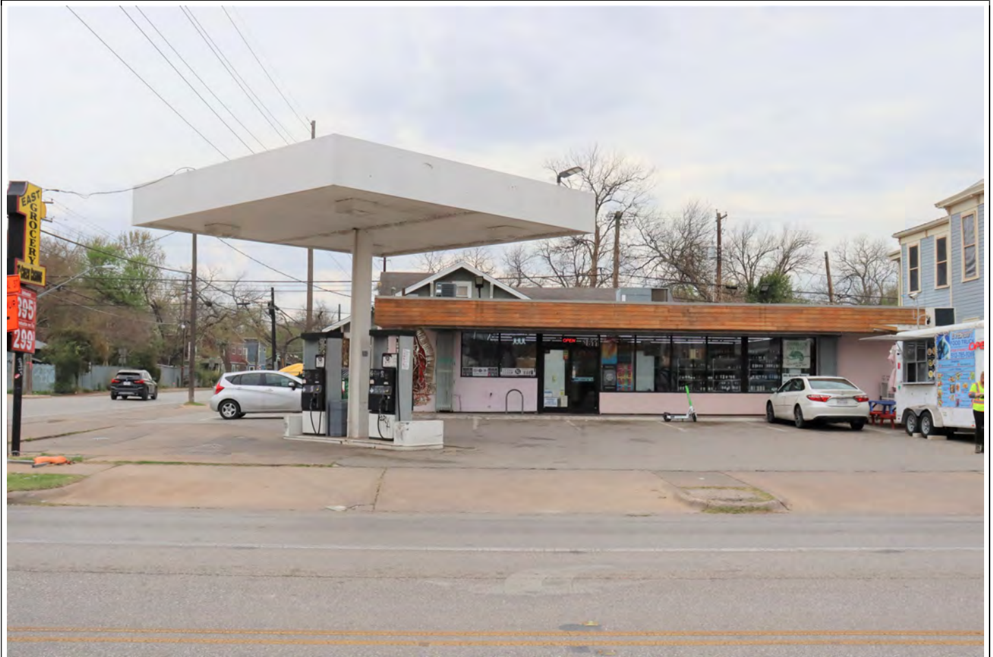
View facing southwest.
