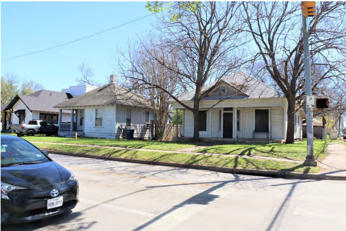
2200 block, view facing southeast. Resources 1098-1100 (right to left) visible.
