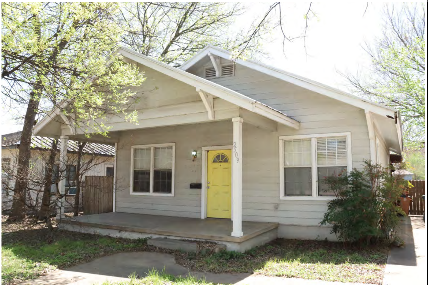
View facing southeast.
