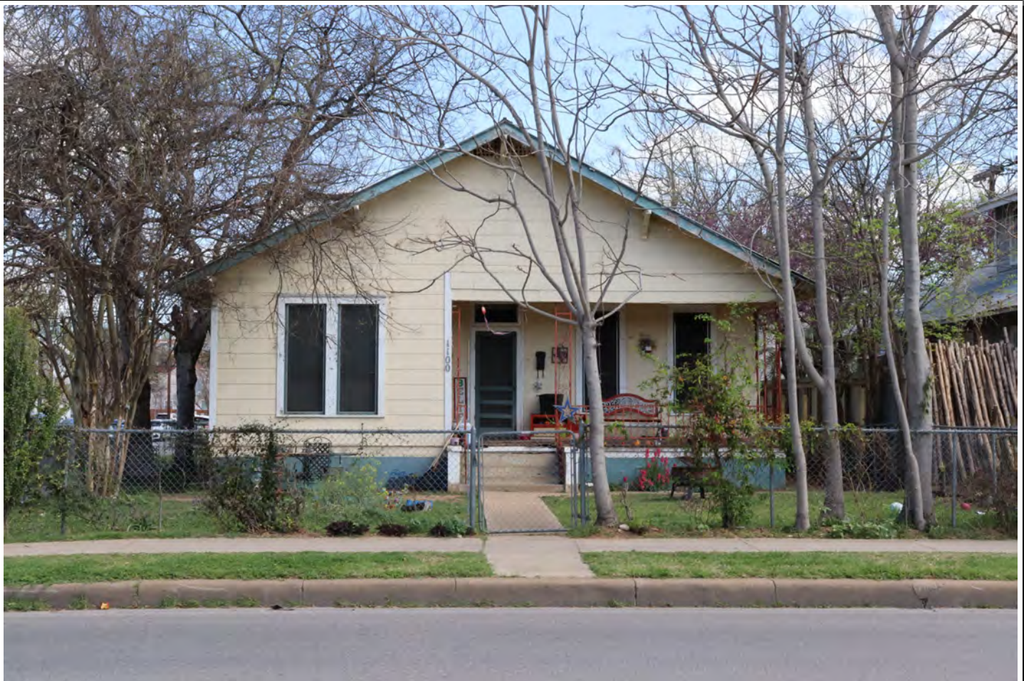
View facing north.
