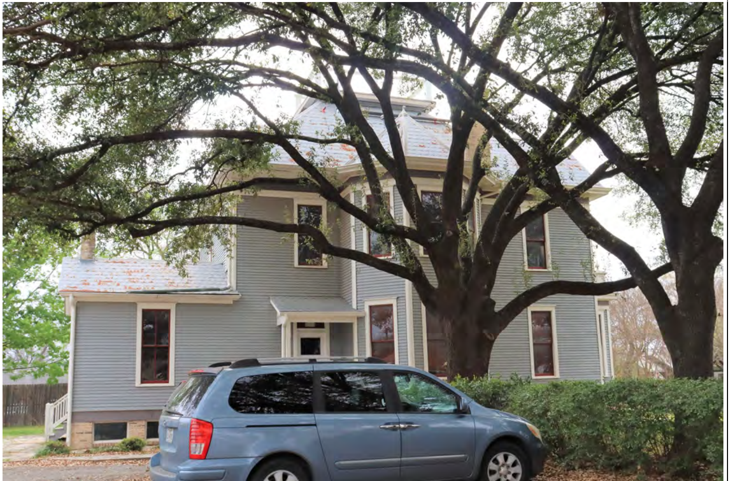
View facing southeast.
