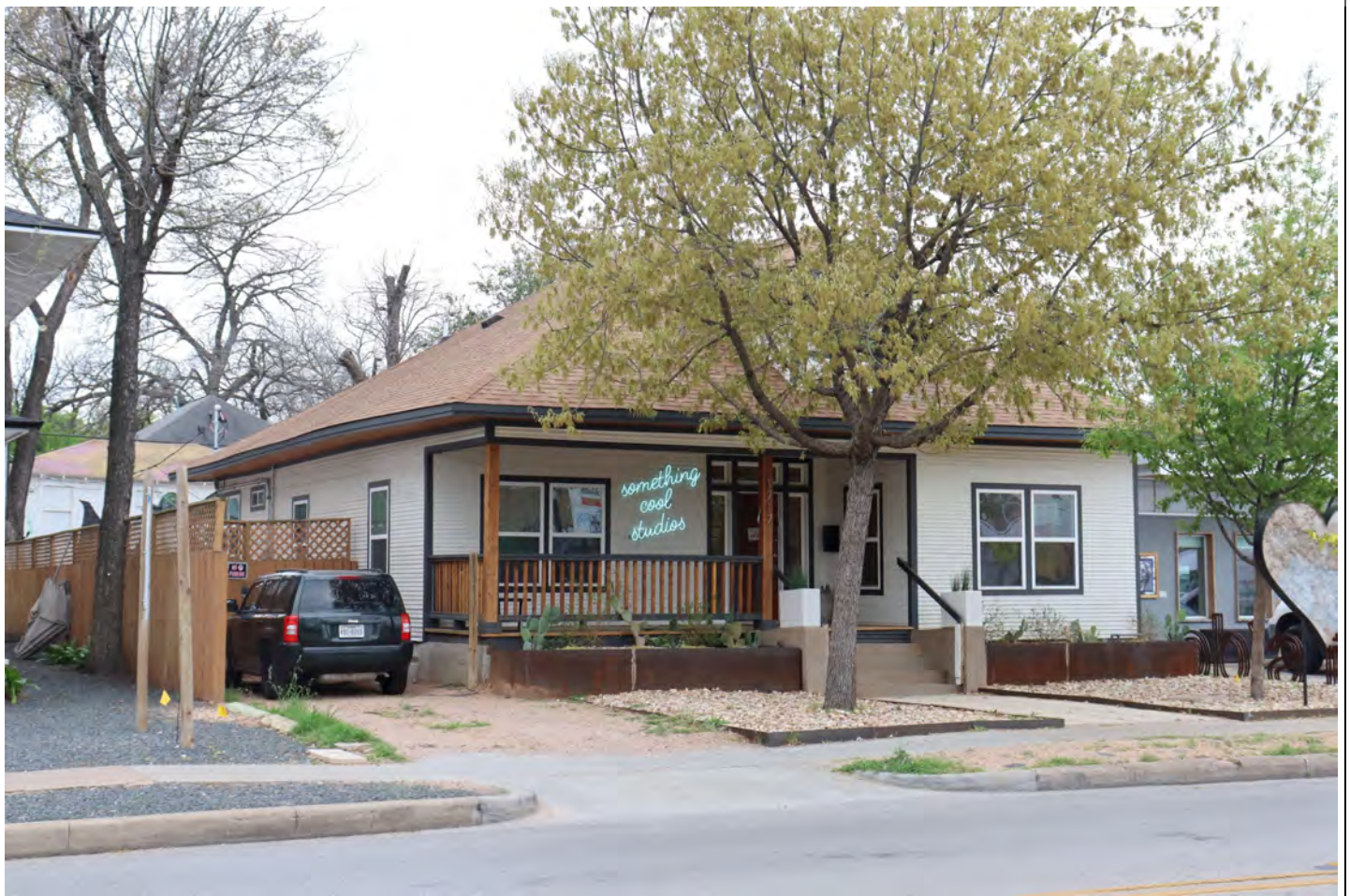
View facing southwest. Showing relationship between 1053A (right) and 1053B (back and left).
