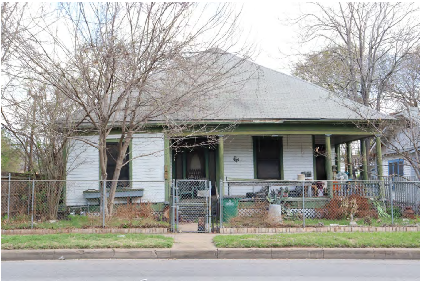
View facing north.
