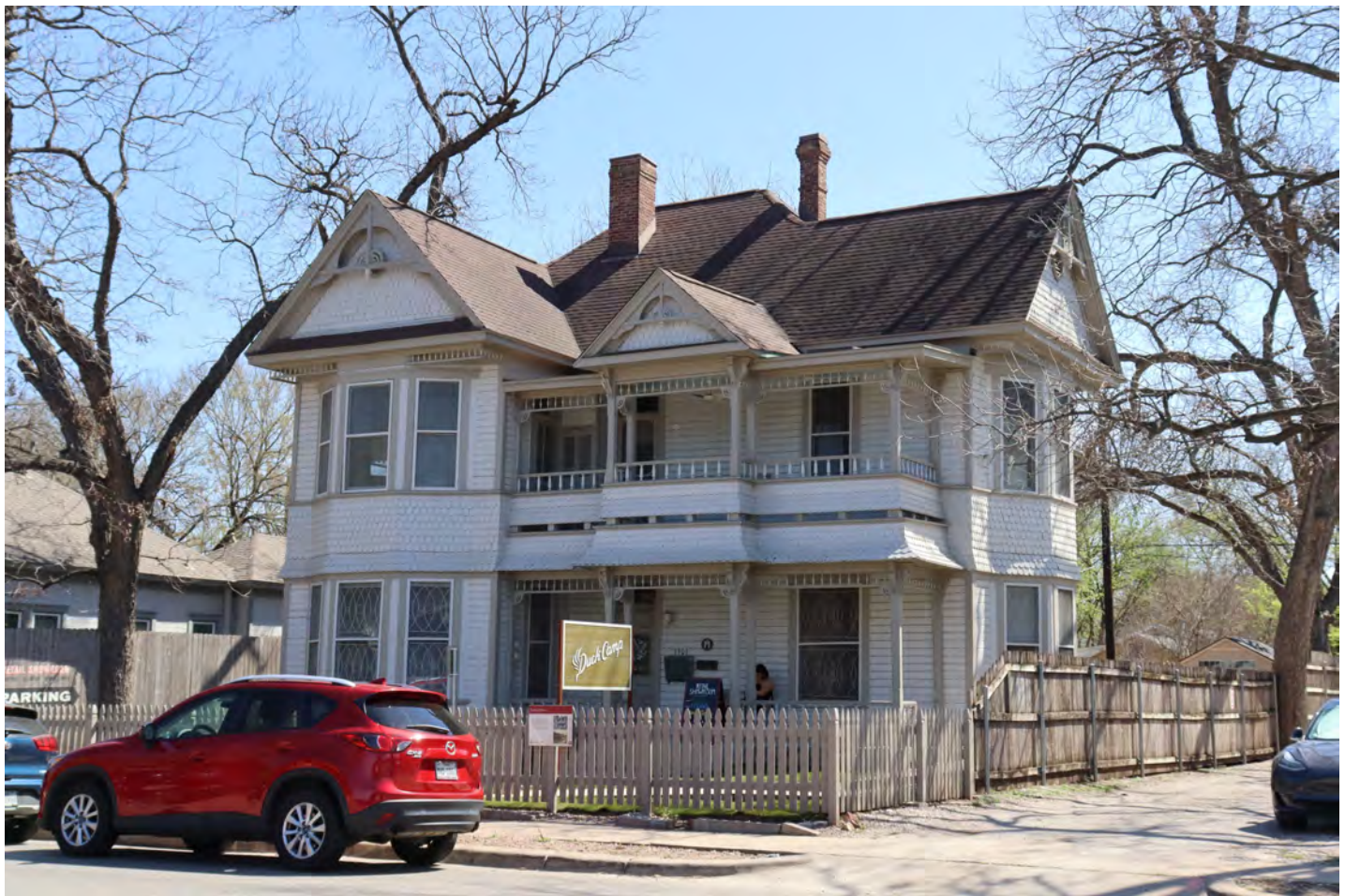
View facing southeast.
