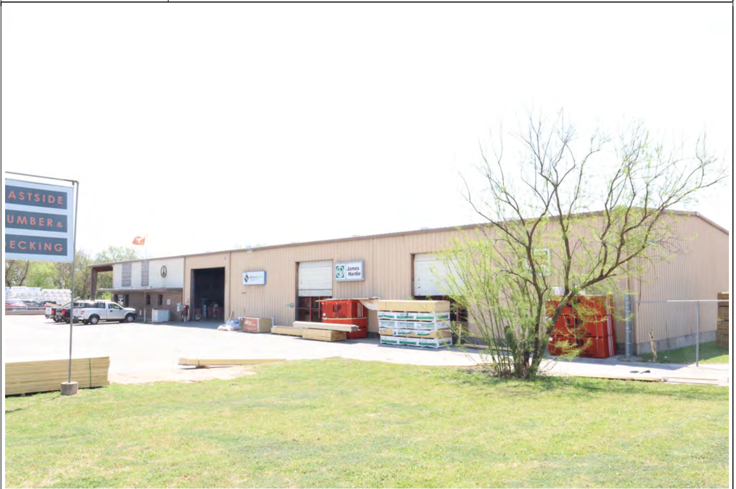
View facing southeast.
