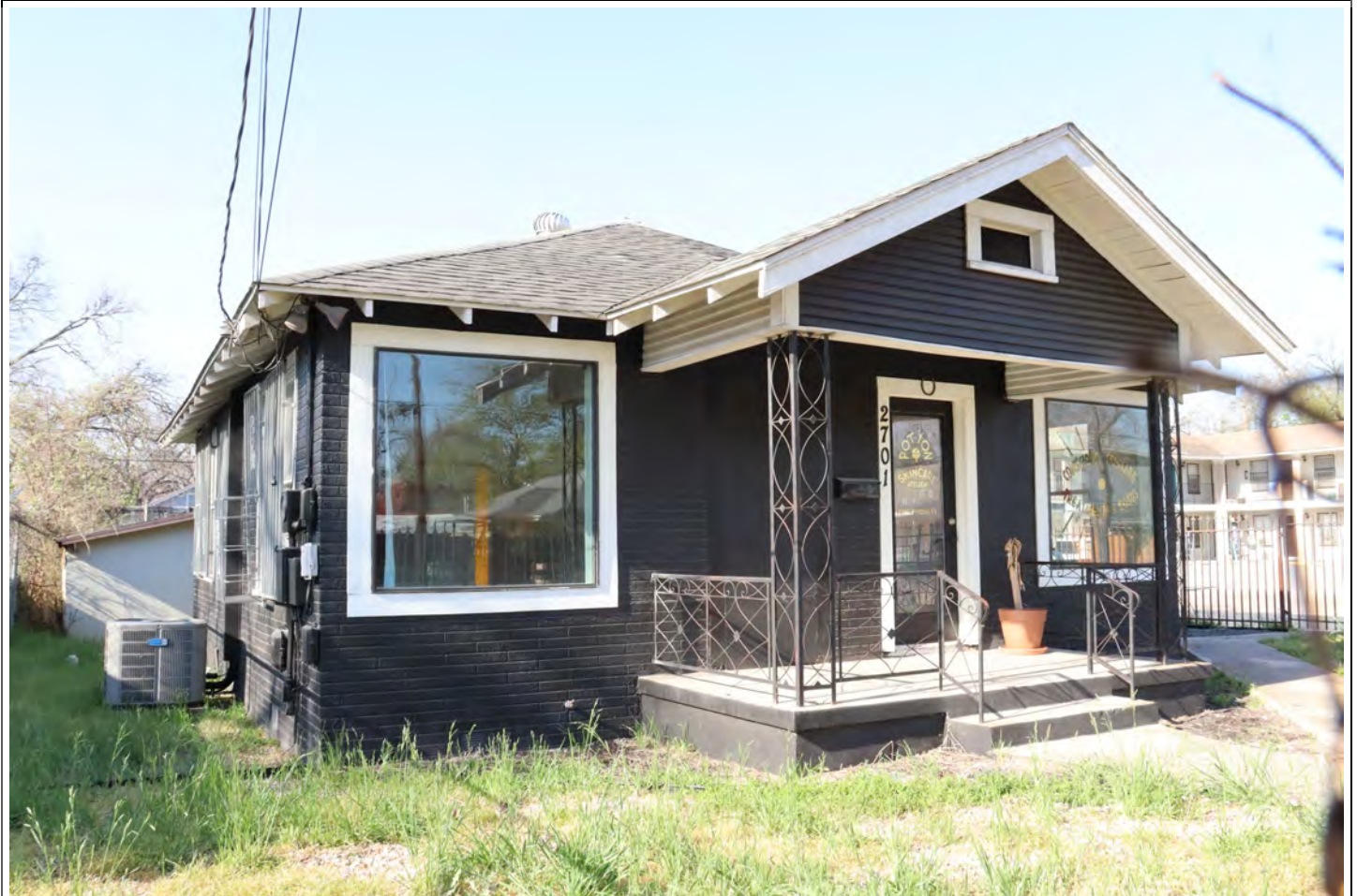
View facing southwest.
