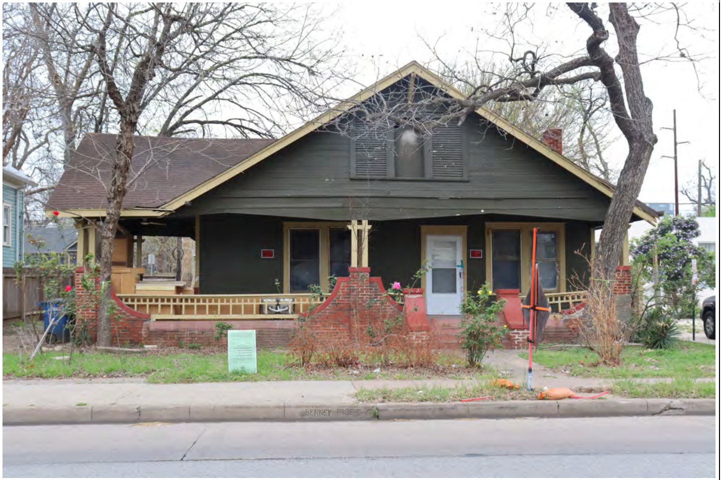
View facing southwest.
