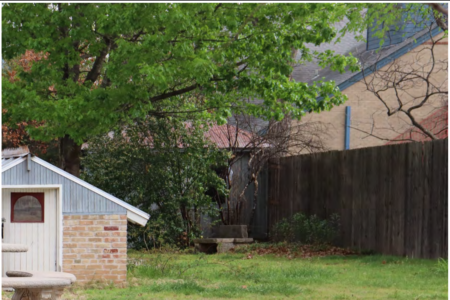
View facing northeast. Showing relationship between 1041D (left) and 1041E (right).
