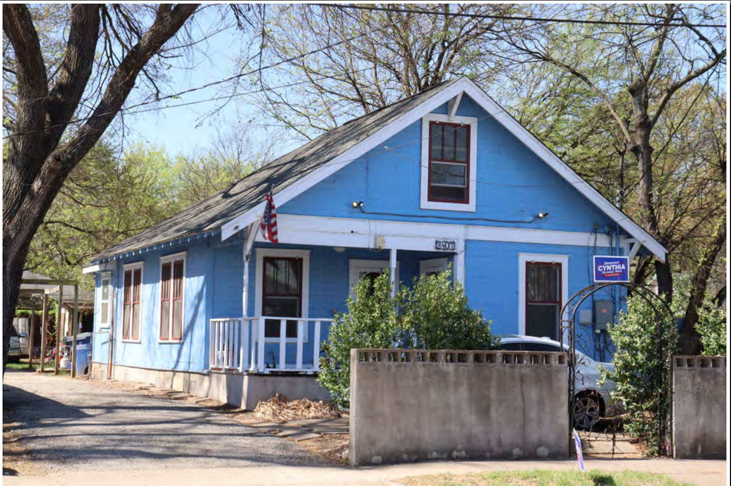
View facing southeast.
