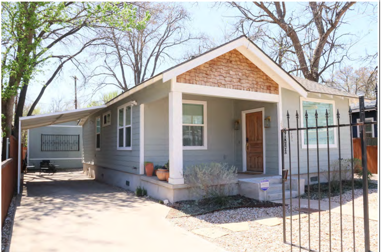
View facing southwest.
