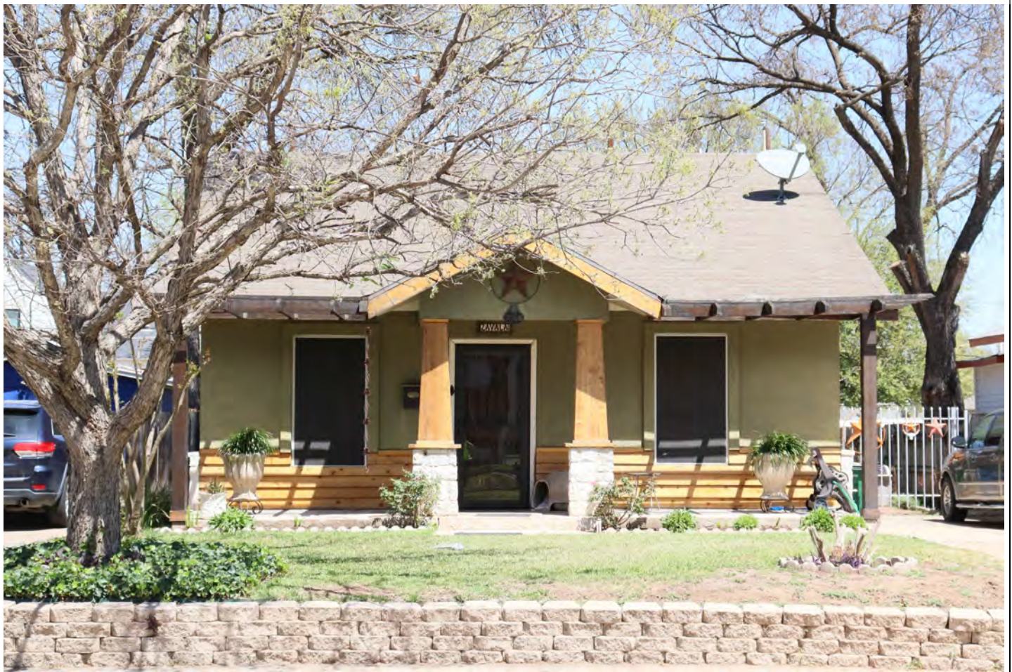
View facing north.
