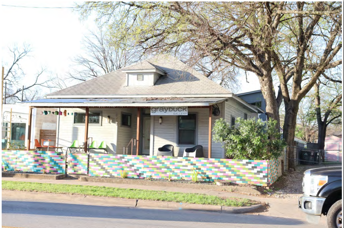
View facing southeast.
