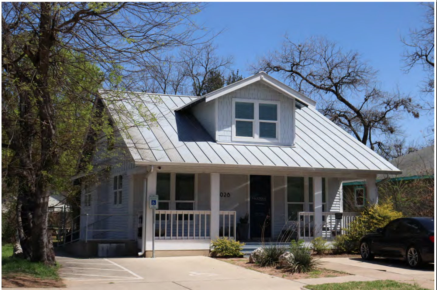
View facing northeast.
