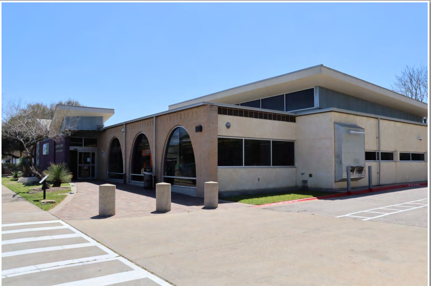
View facing southeast.
