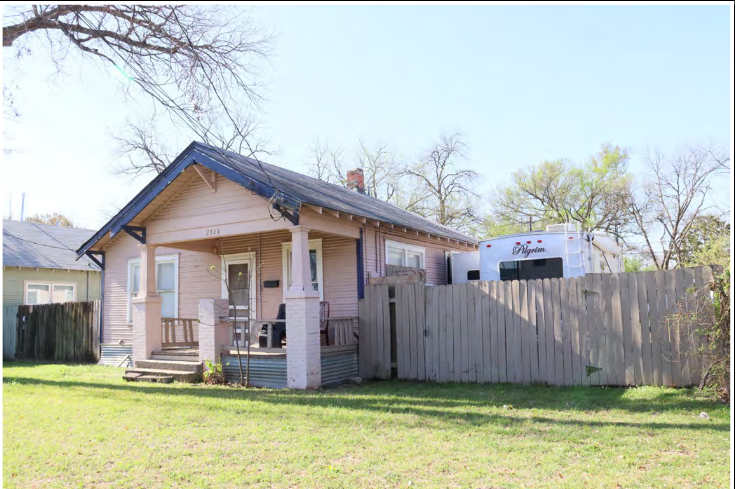
View facing southeast.
