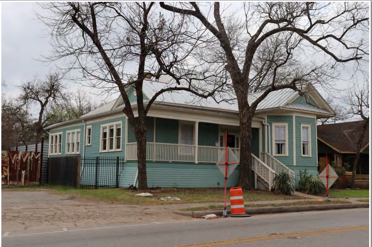
View facing southwest.
