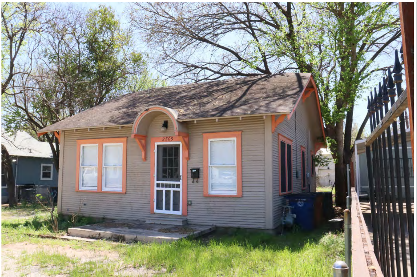
View facing southeast.
