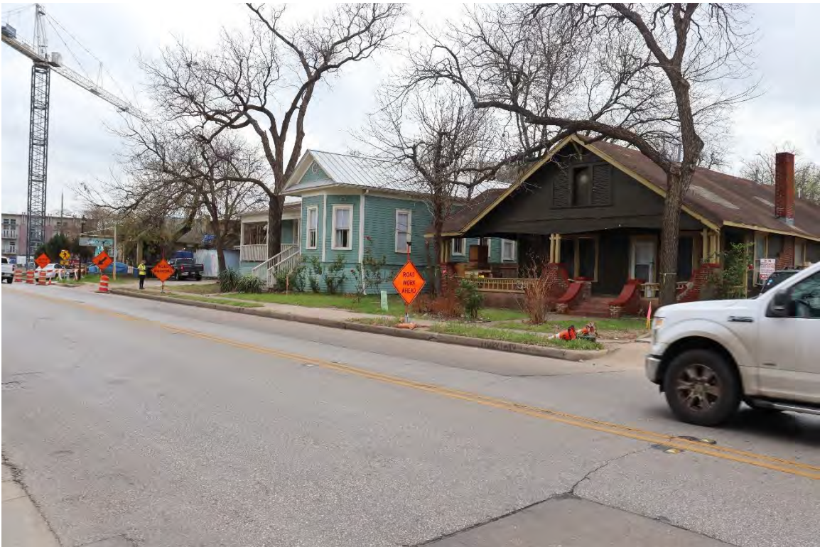
1400 block, view facing southeast. Resource 1037 (right) and 1038 (left) visible.
