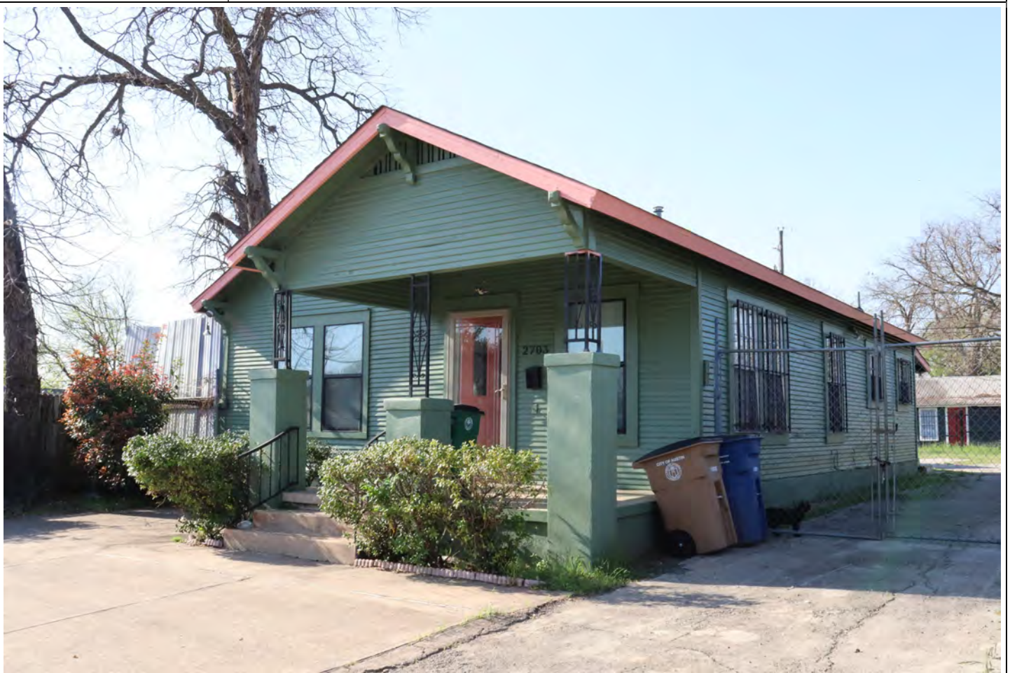
View facing southeast.
