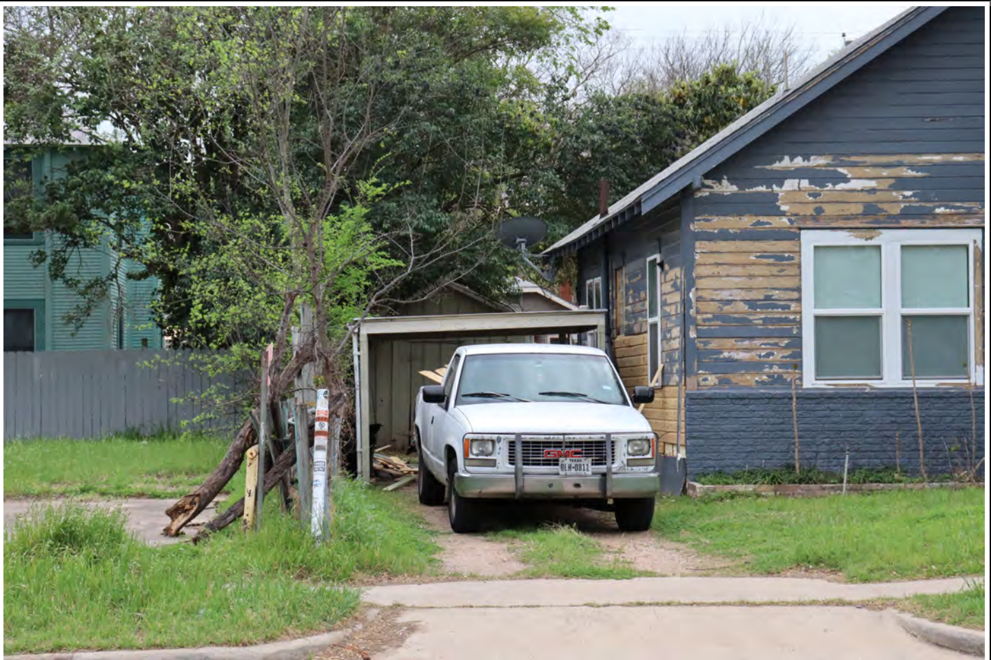
View facing southwest. Showing relationship between 1063A (right) and 1063B (back and left).
