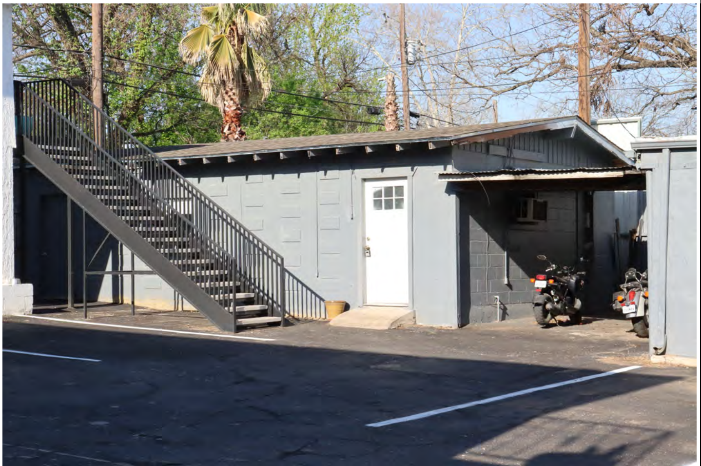
View facing southwest.
