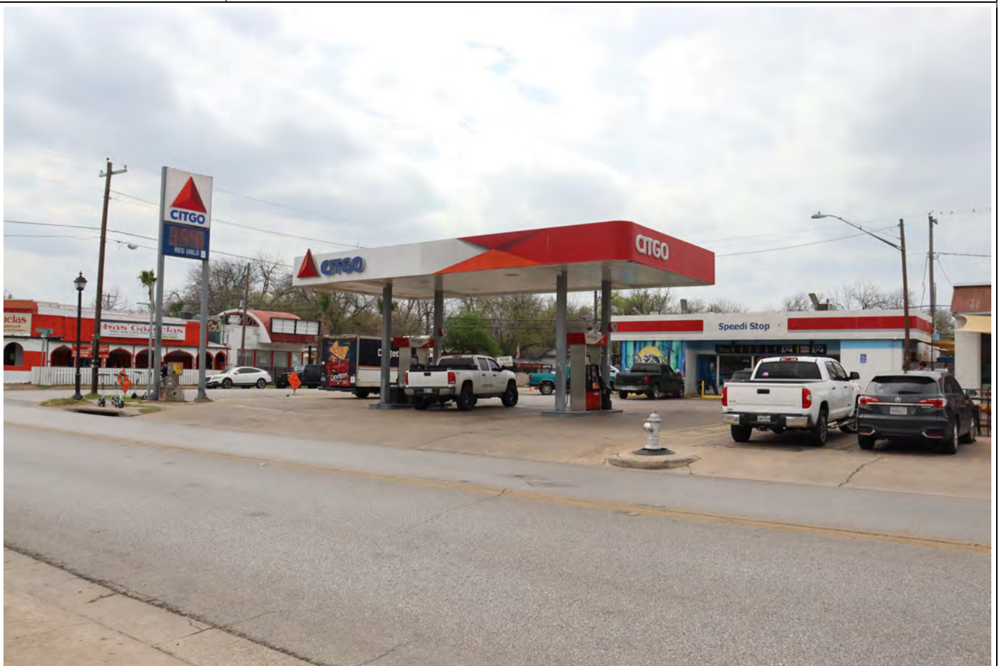
View facing southwest.
