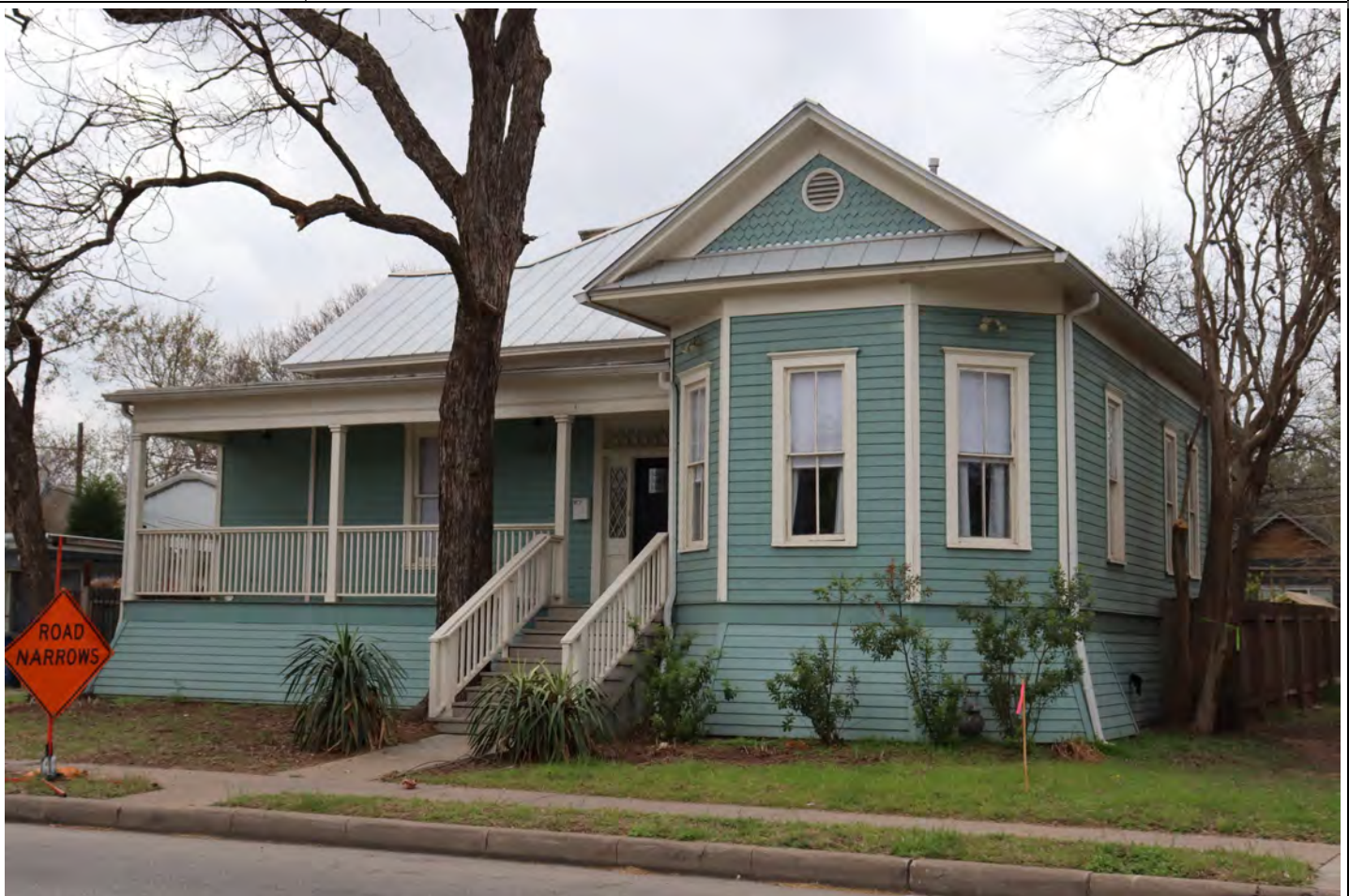
View facing southeast.
