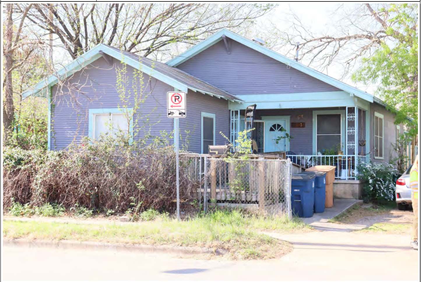
View facing southeast.
