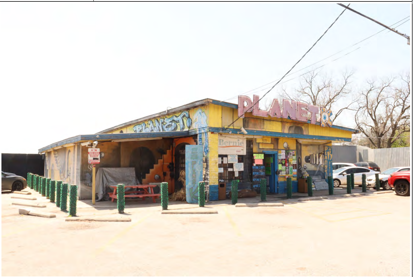
View facing southwest.
