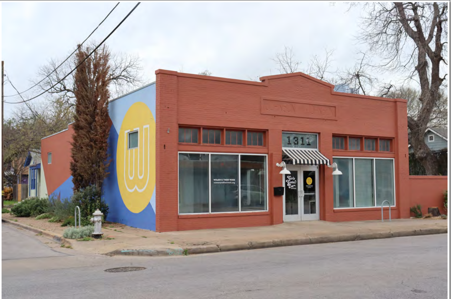
View facing southwest.
