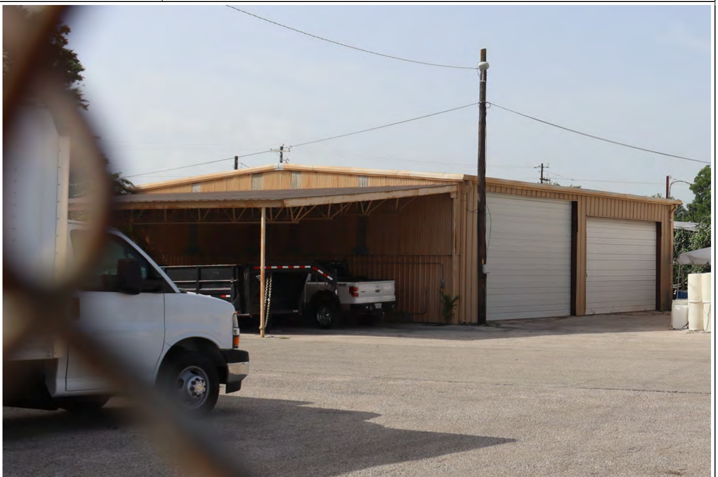
View facing southwest.
