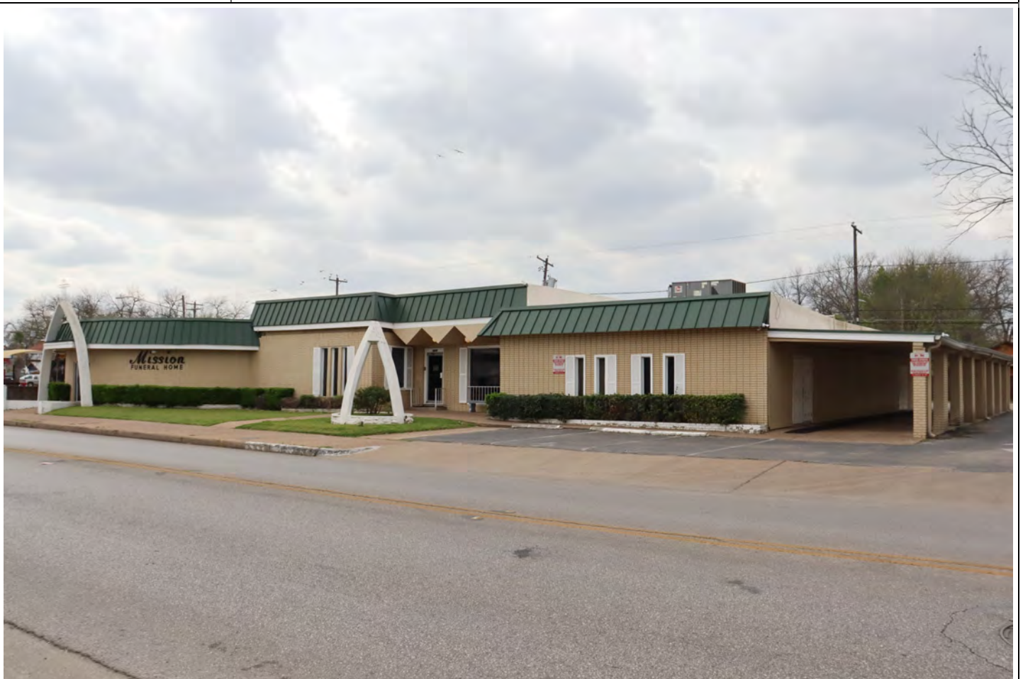
View facing southeast.
