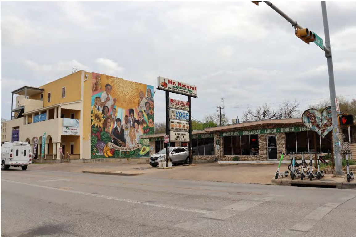
1900 block, view facing southeast. Resource 1061 at right.
