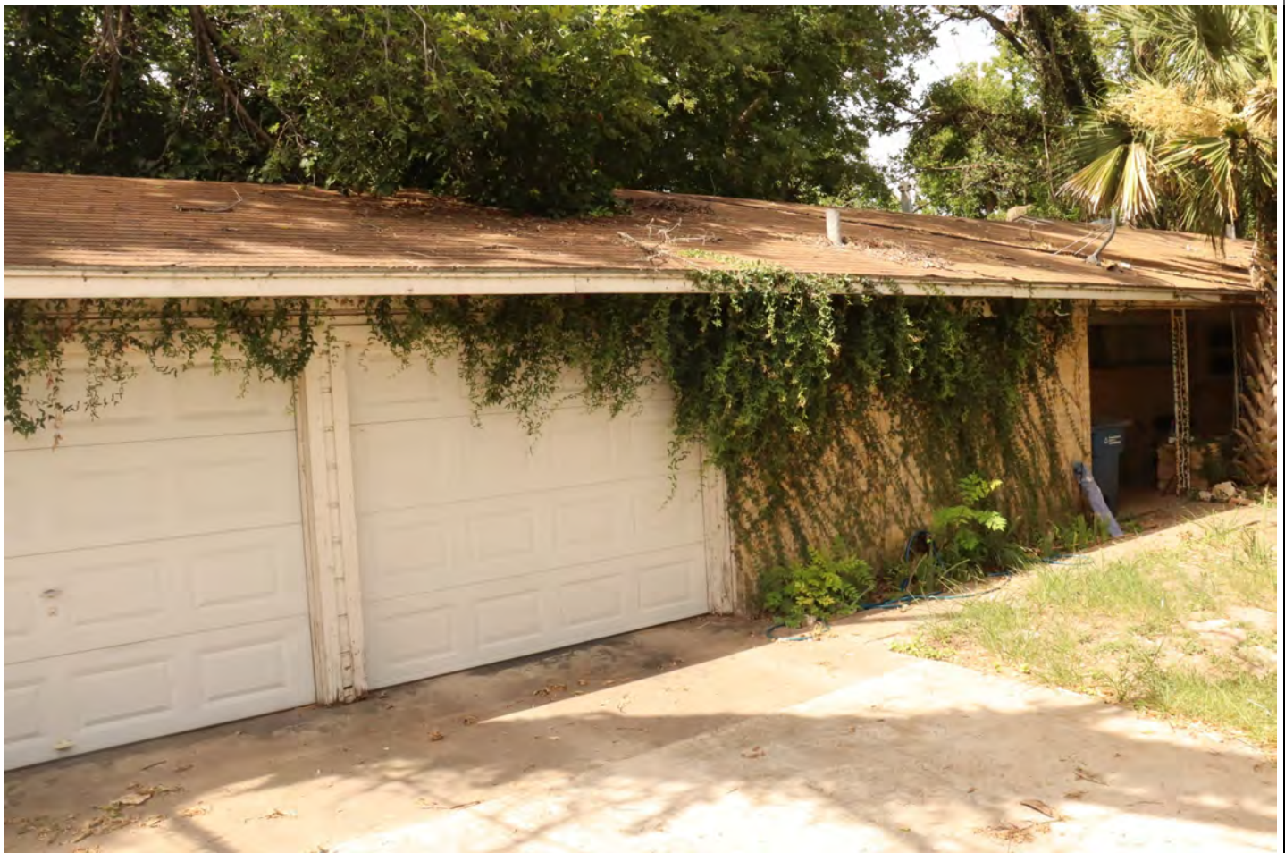
View facing southwest.
