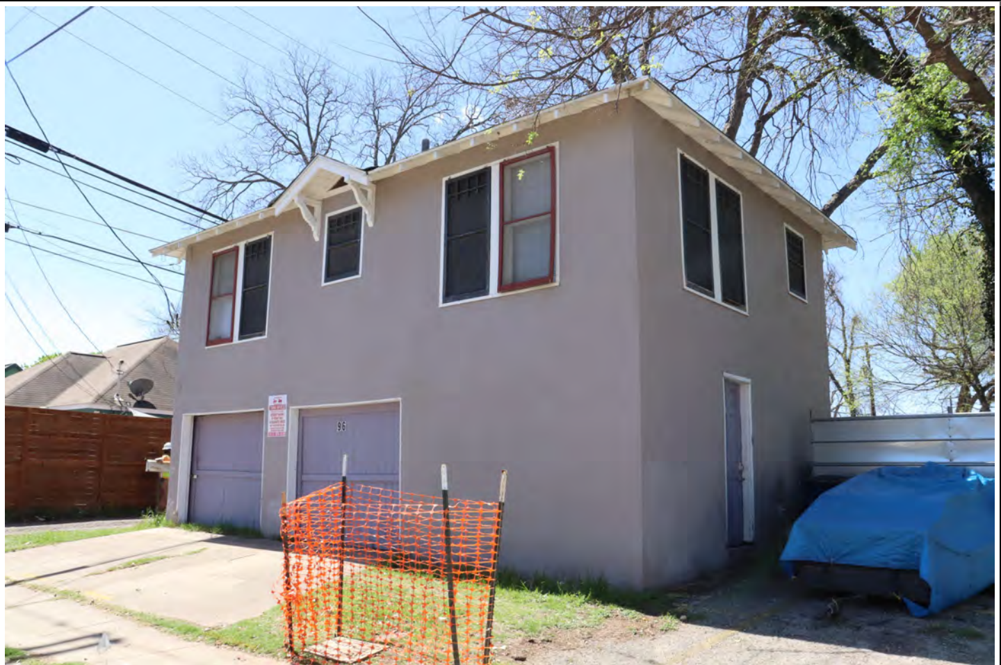
View facing southwest.
