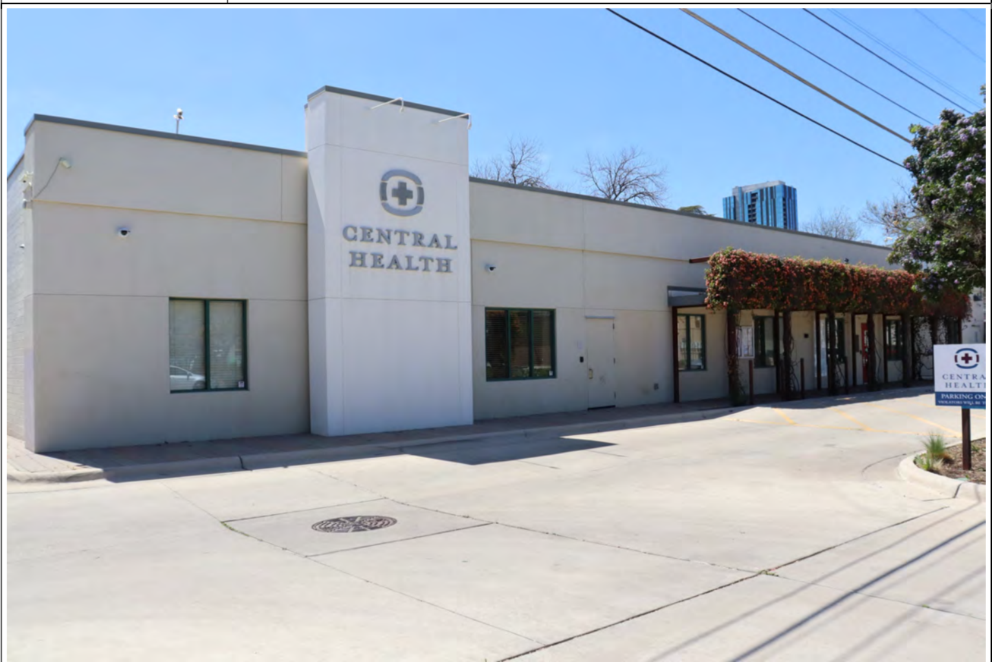
View facing southwest.
