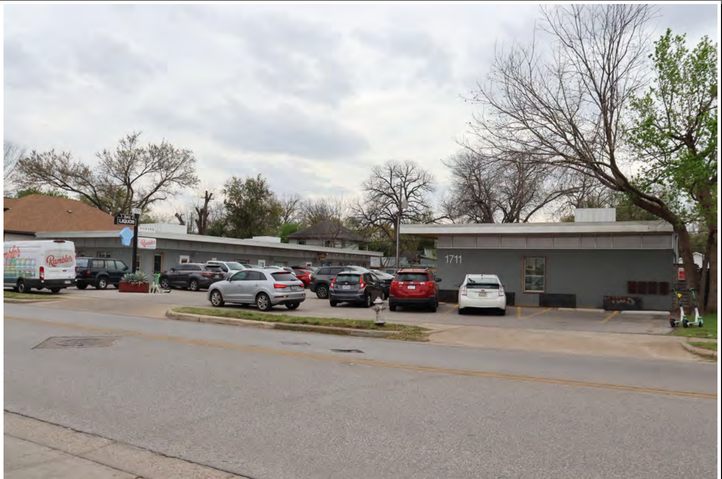
View facing southwest.
