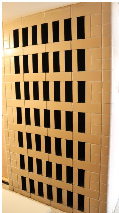
Interior pierced glazed brick wall.
