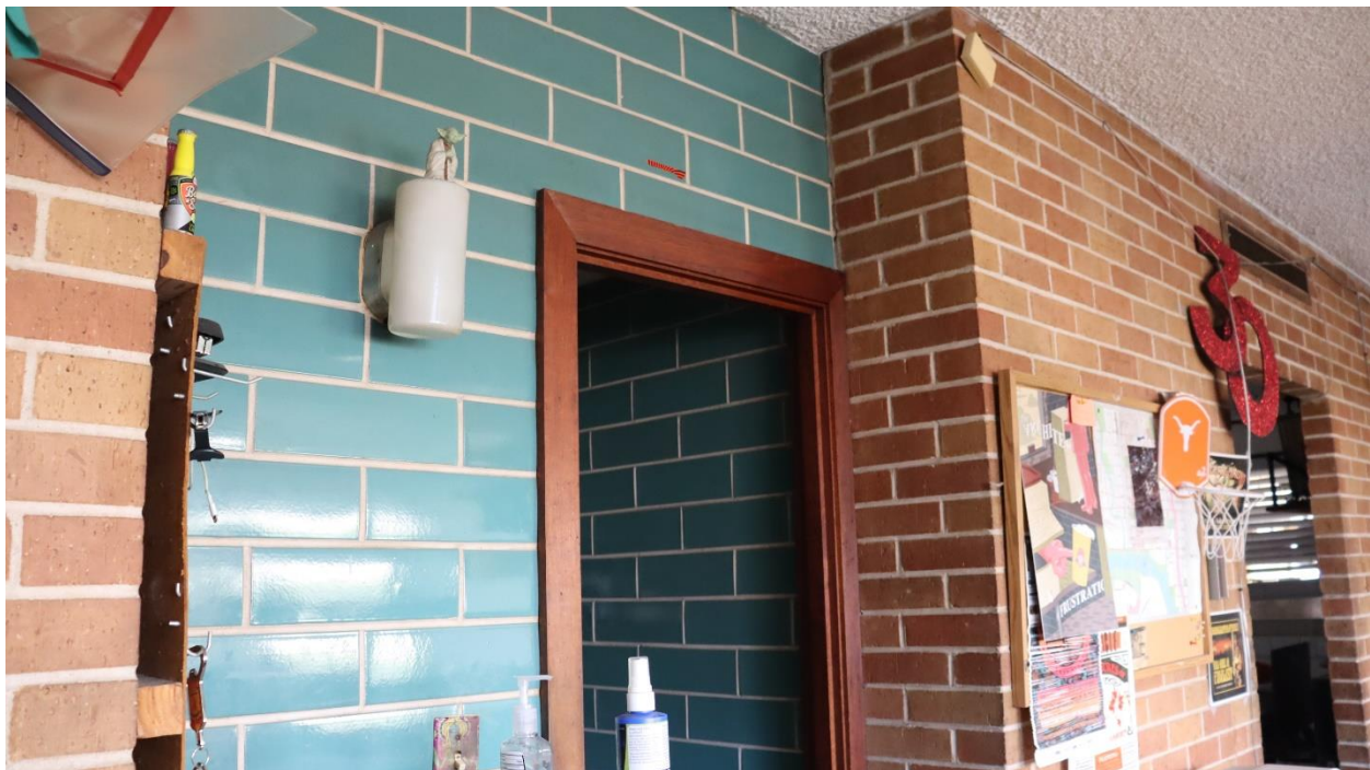
Interior office showing use of three kinds of brick.
