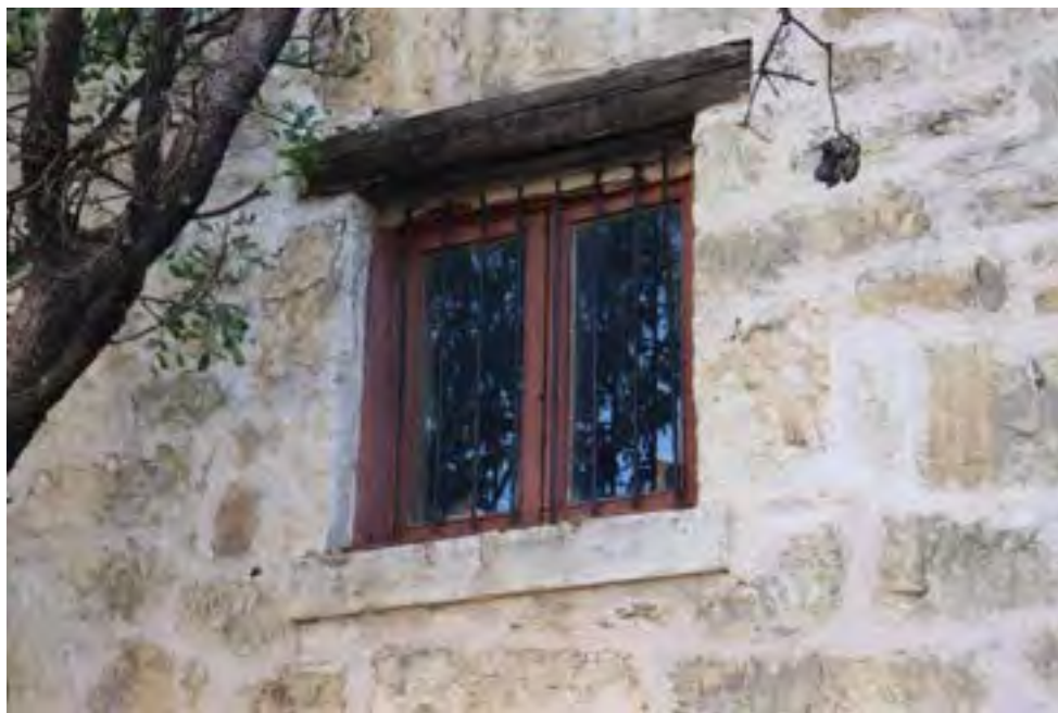
Detail of wooden lintel on west elevation, view facing northeast.
