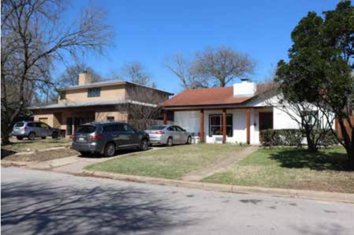
Bentwood Road. Outside project APE. View facing north.
