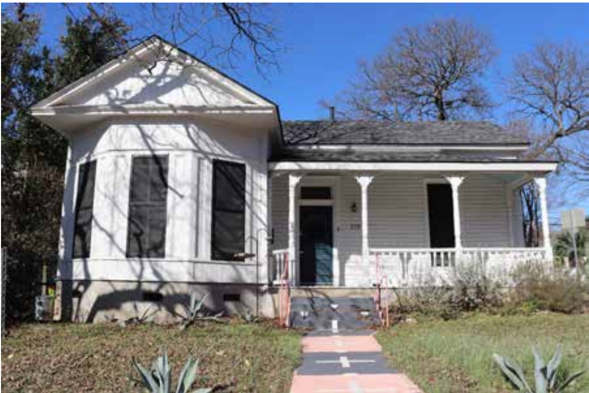
Resource 334, Contributing: 910 East 14 th Street. View Facing northwest.
