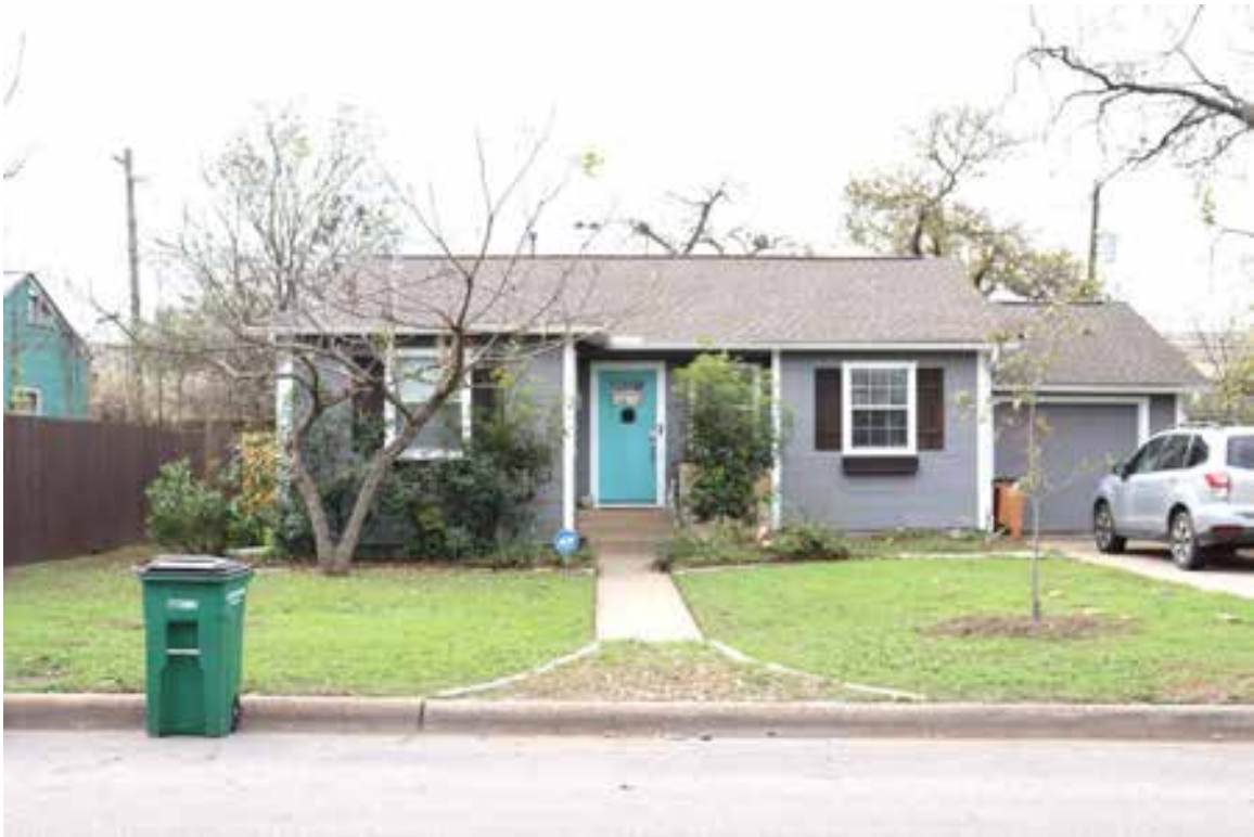
Resource 160: 1035 East 43 rd Street. View facing southwest.
