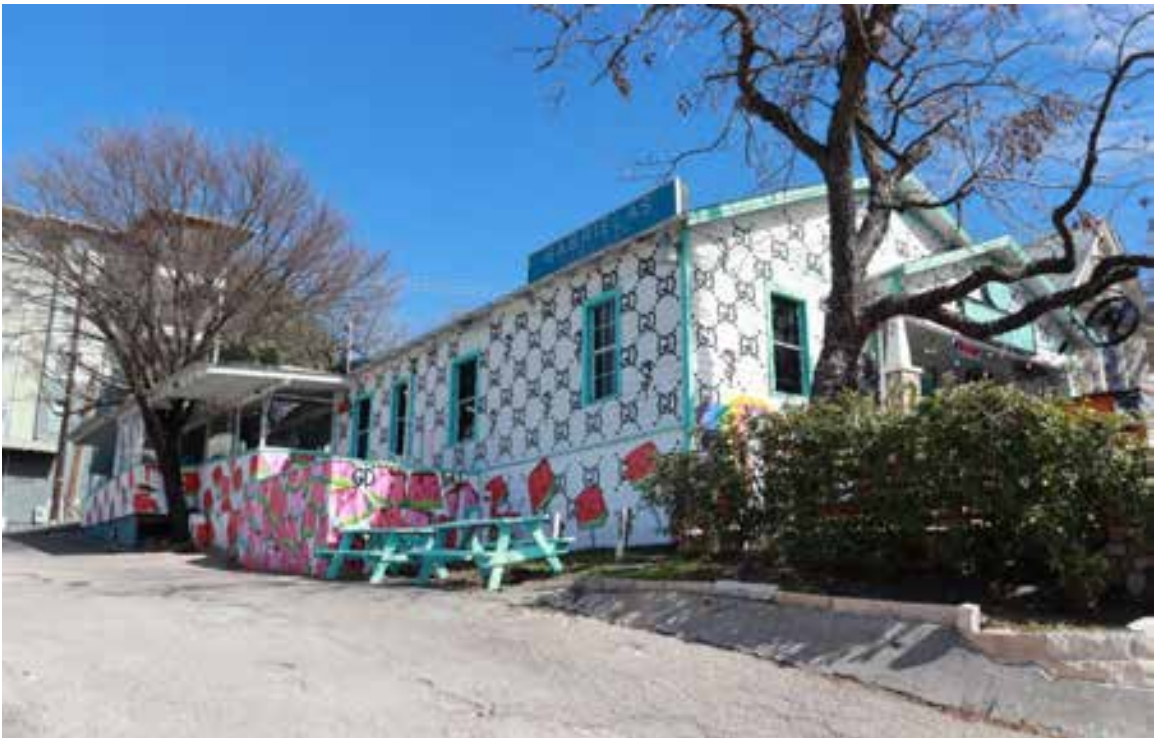
Resource 366: 900 East 7 th Street. View facing northeast.
