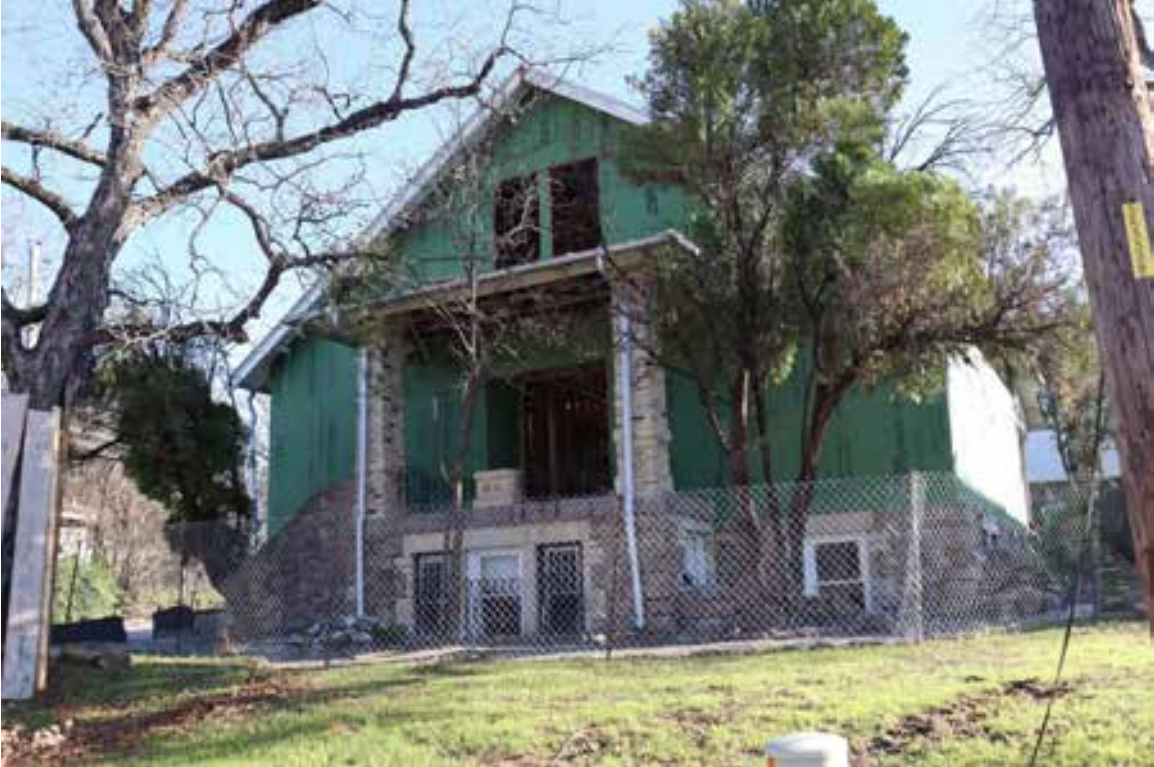
Resource 322: 811 East 15 th Street. View facing southeast.
