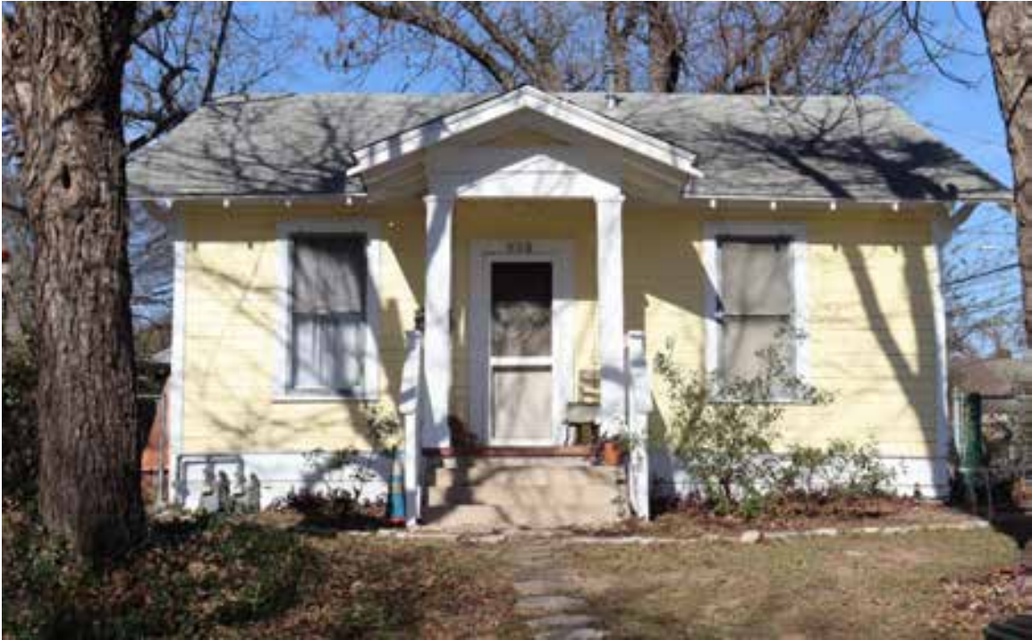
Resource 441A: 908 Taylor Street. View facing northeast.
