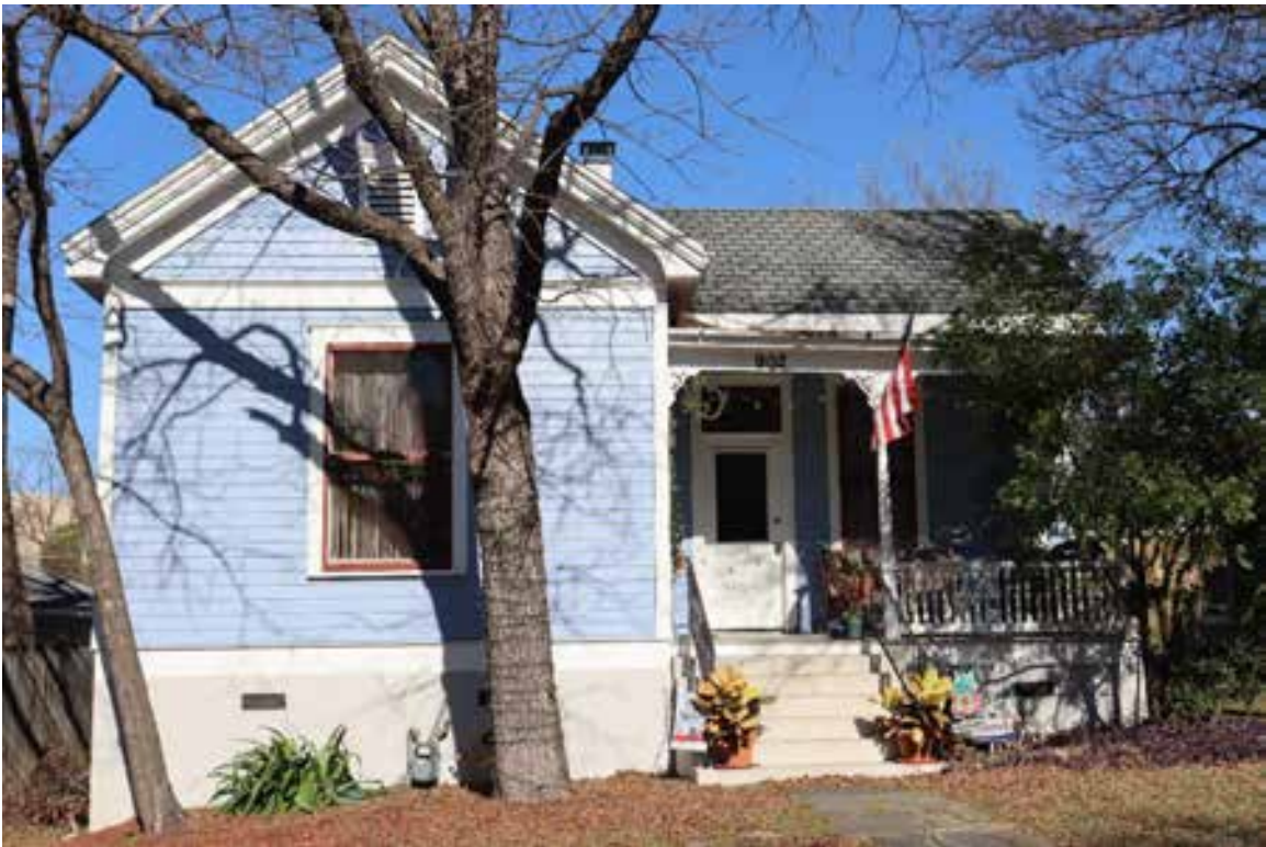
Resource 330, Contributing: 902 East 14 th Street. View facing northwest.
