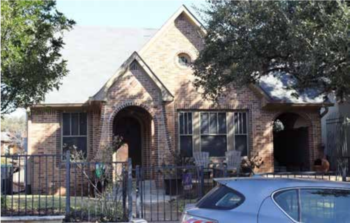
Resource 471, Contributing: 1016 Hardwood Place. View facing northeast.
