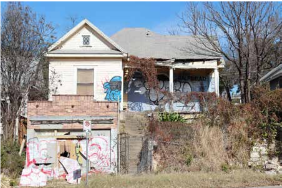
Resource 368: 904 East 7 th Street. View facing northeast.
