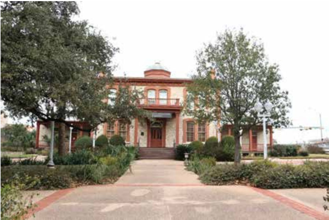
Resource 320A, Contributing: 709 East MLK Jr. Boulevard. View facing north.
