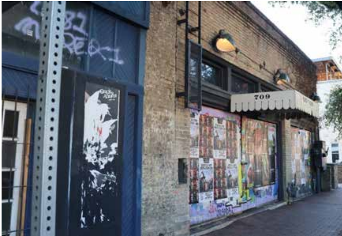
Resource 383, Contributing: 709 East 6 th Street. View facing west.
