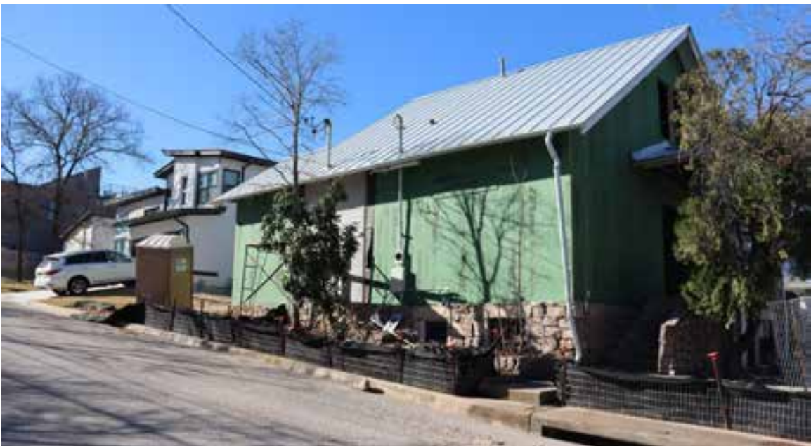
Intersection of East 16 th and Waller Streets. Resource 322. View facing southwest.
