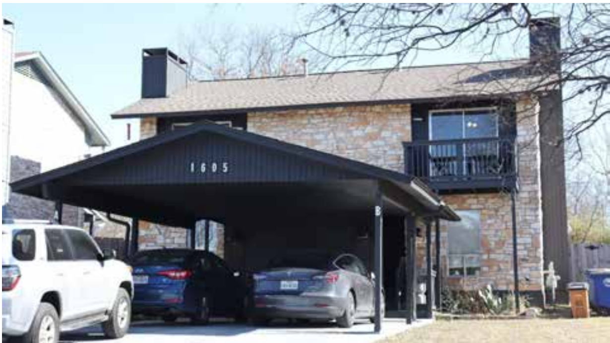
Resource 507: 1605 Summit Street. View facing southwest.
