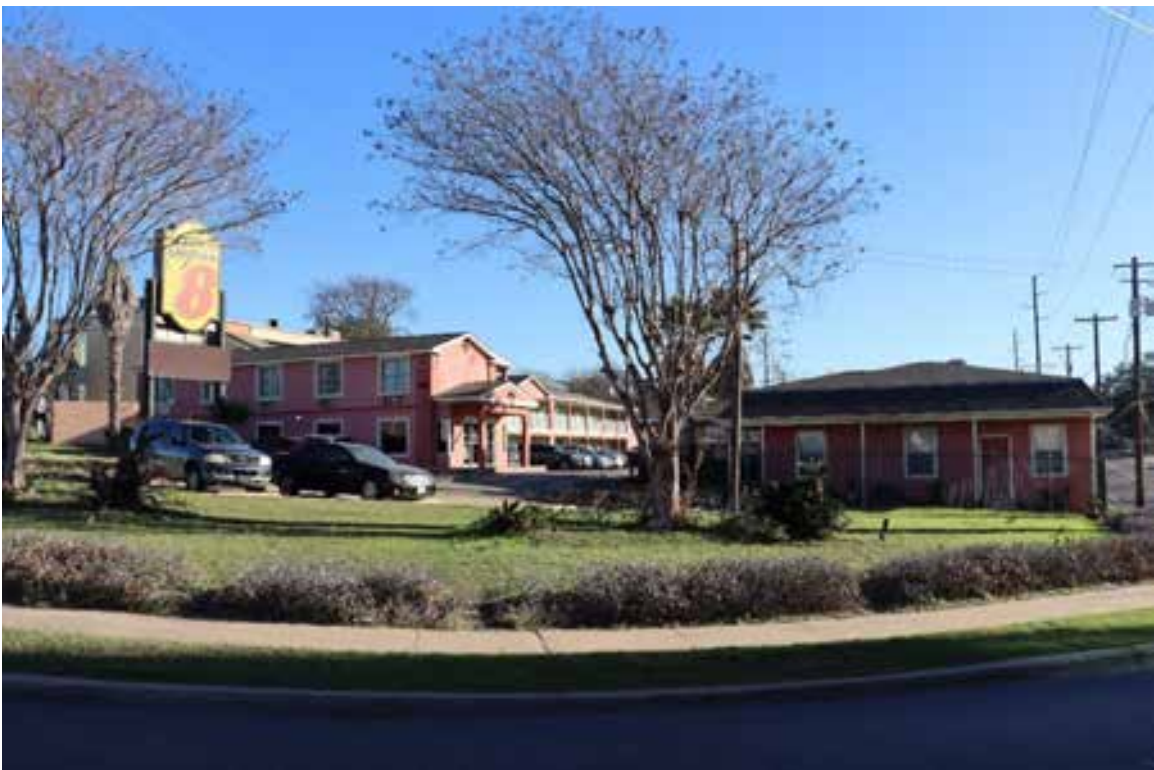
Resource 347: 900 East 12 th Street. View facing northeast.
