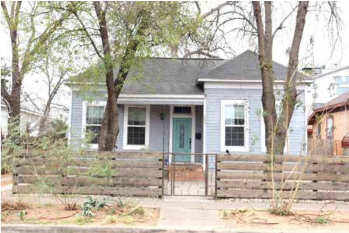
Resource 411: 903 East 2 nd Street. View facing southwest.
