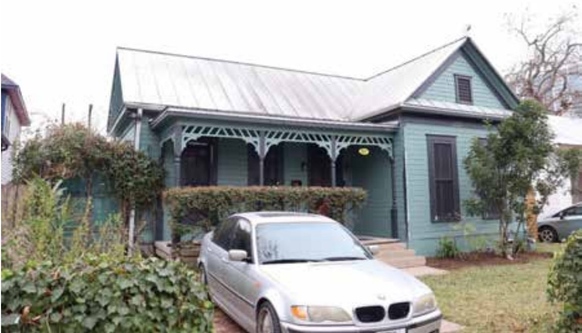
Resource 413: 907 East 2 nd Street. View facing southwest.
