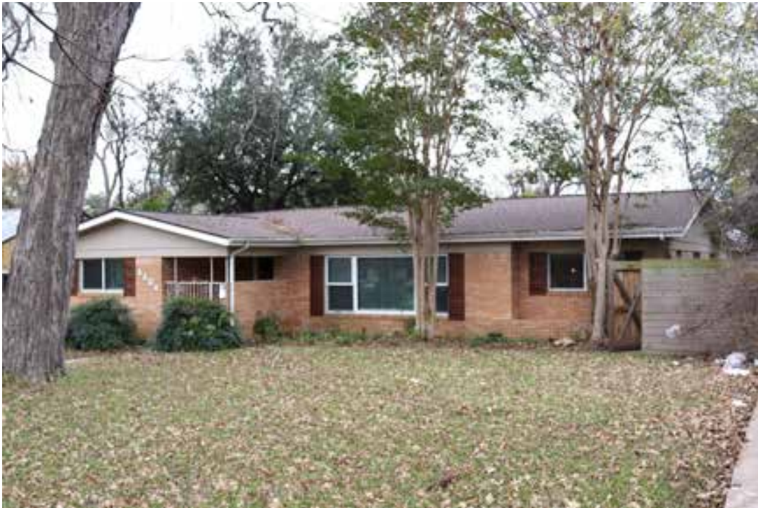
Resource 146: 4404 Airport Boulevard. View facing southwest.
