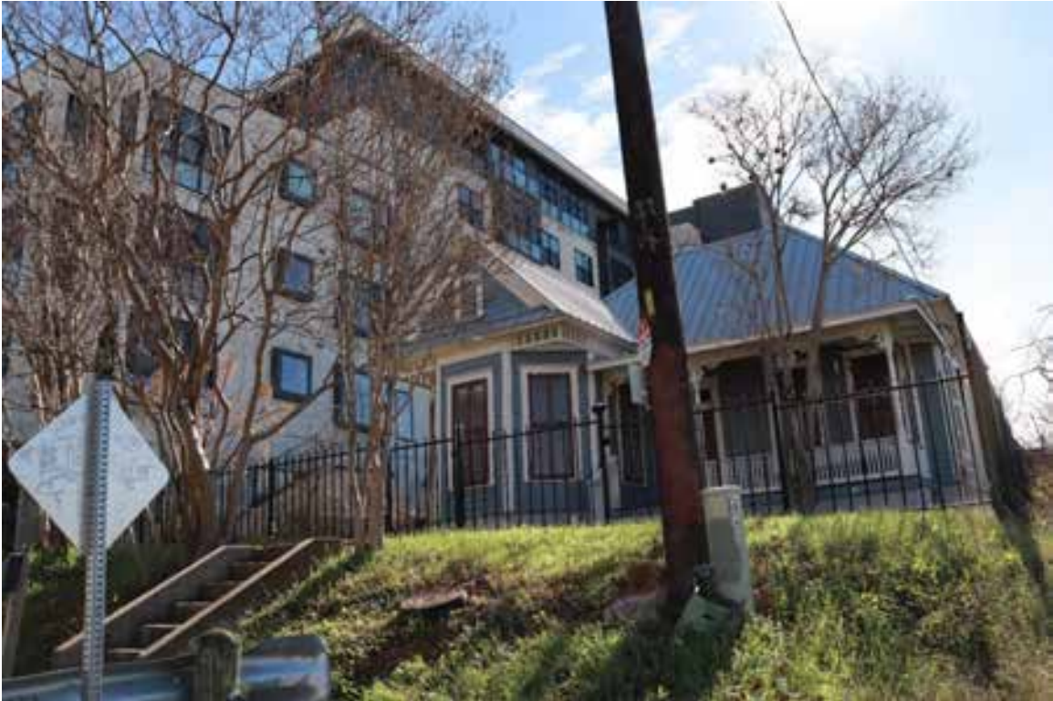
Resource 360: 809 East 9 th Street, and non-historic-age infill (left). View facing southeast.
