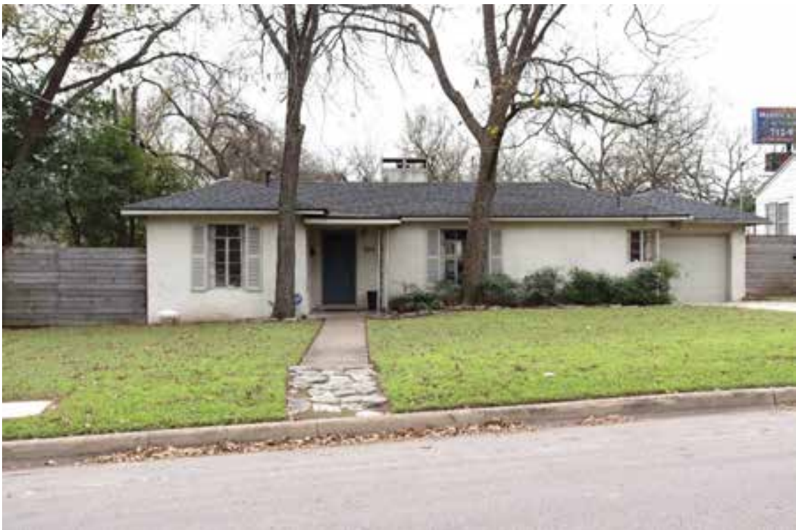
Resource 116: 1103 Bentwood Road. View facing southwest.
