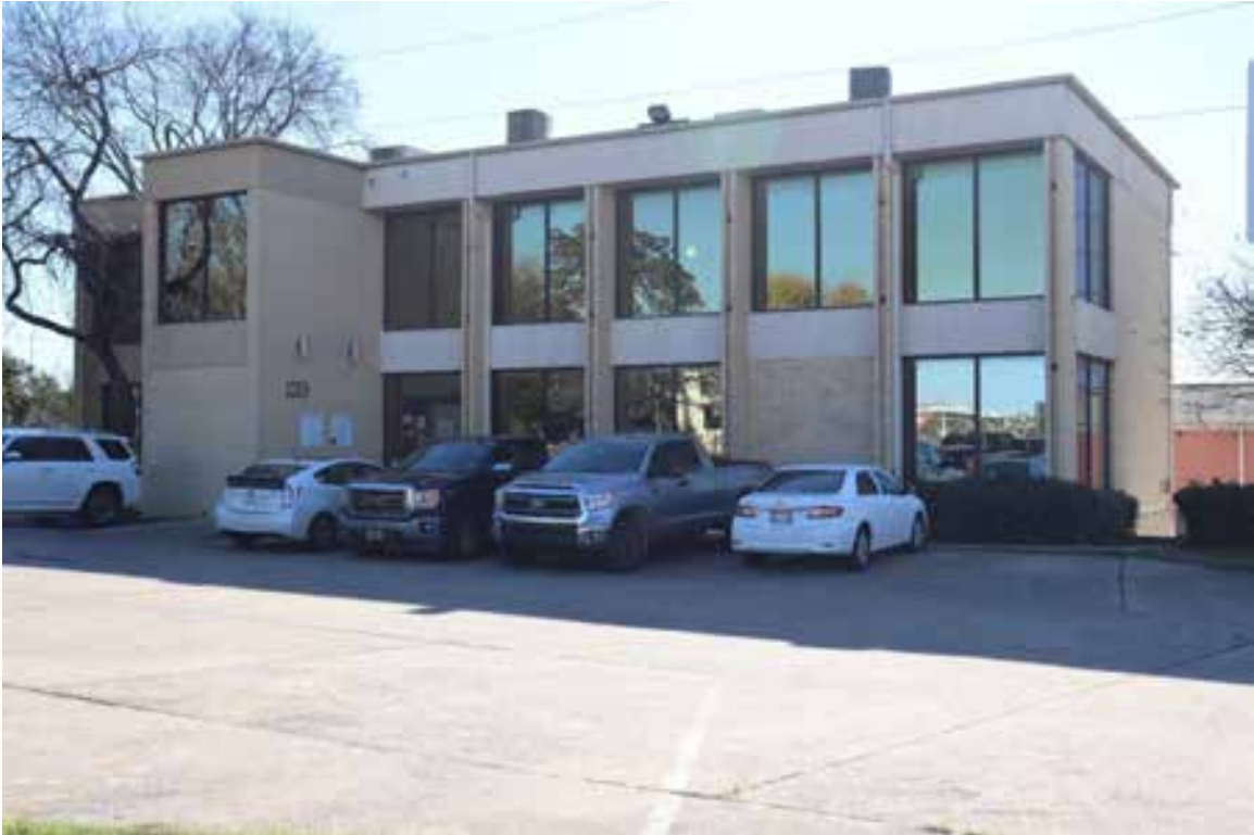
Resource 340: 809 East 13 th Street. View facing southeast.
