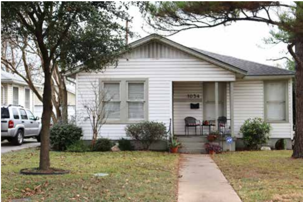
Resource 132: 1034 East 44 th Street. View facing northeast.
