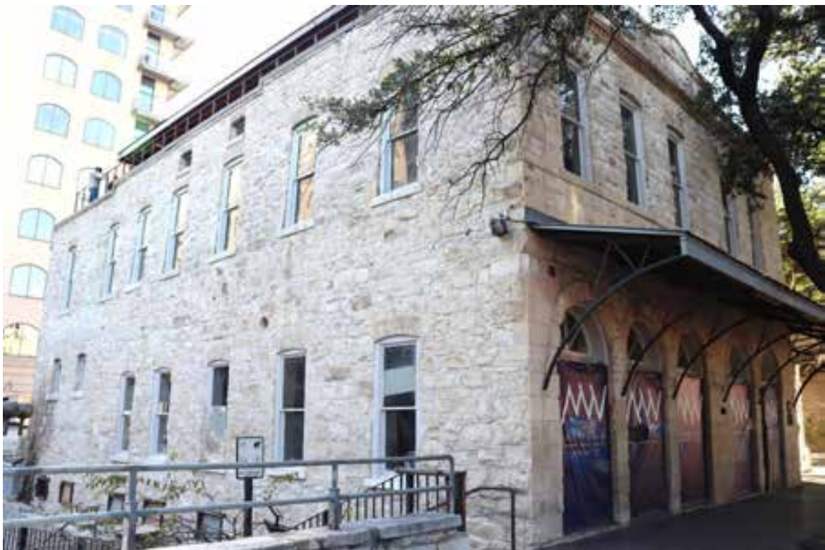
Resource 382, Contributing: 701 East 6 th Street. View facing west.
