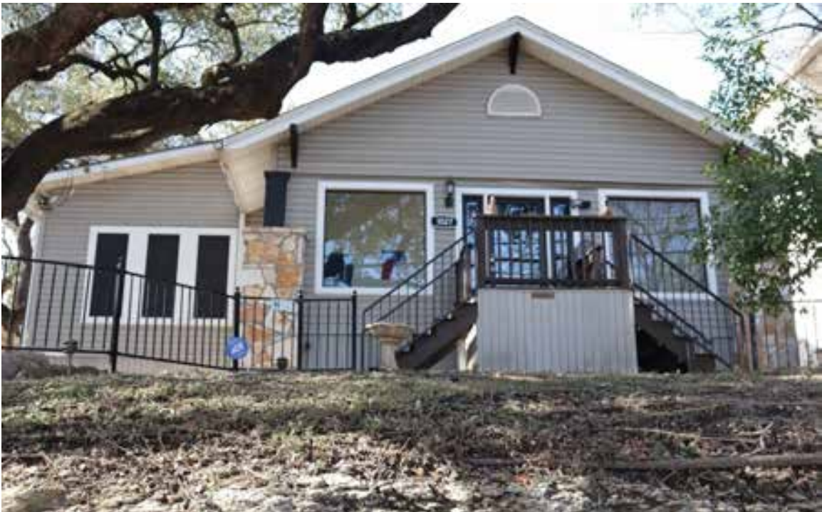
Resource 470, Noncontributing: 1027 East Riverside Drive. View facing southwest.
