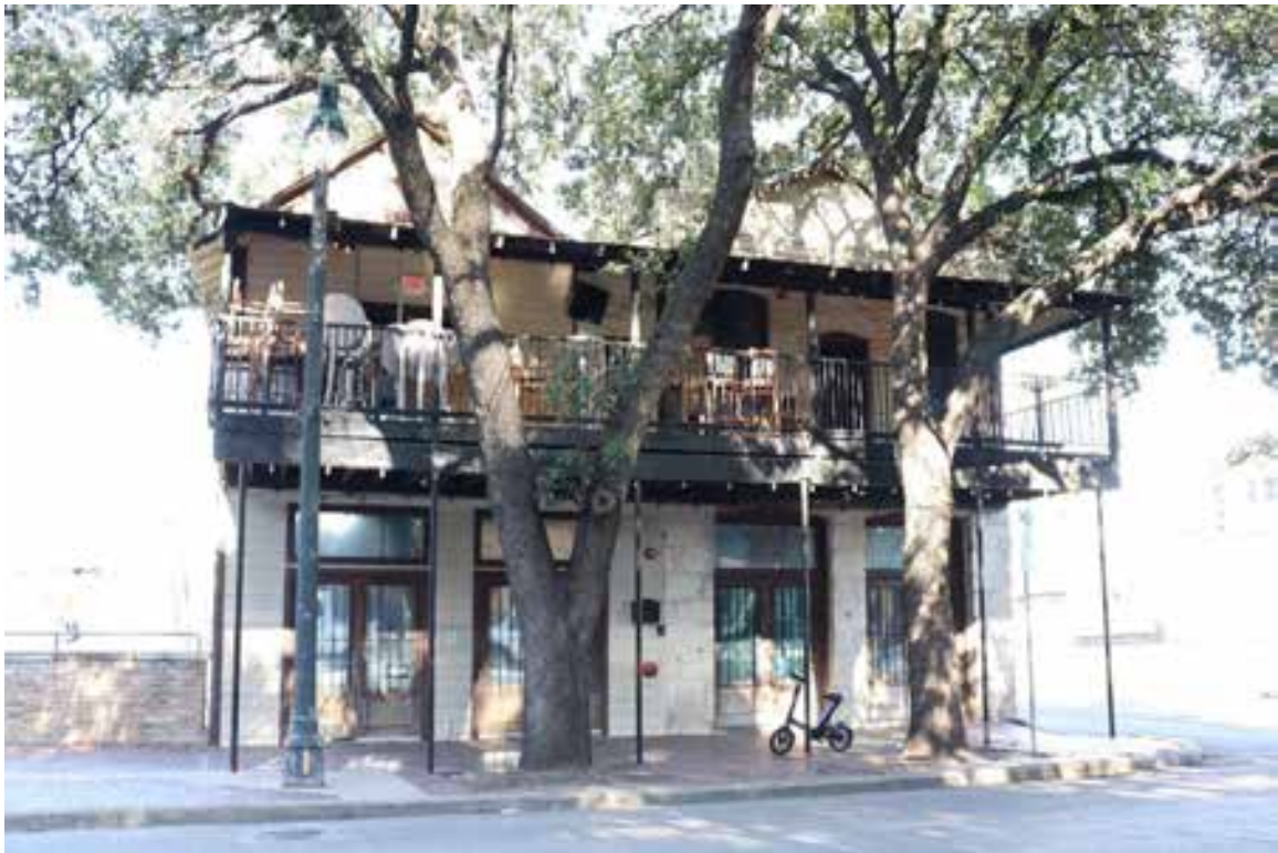
Resource 378, Contributing: 706-708 East 6 th Street. View facing east.
