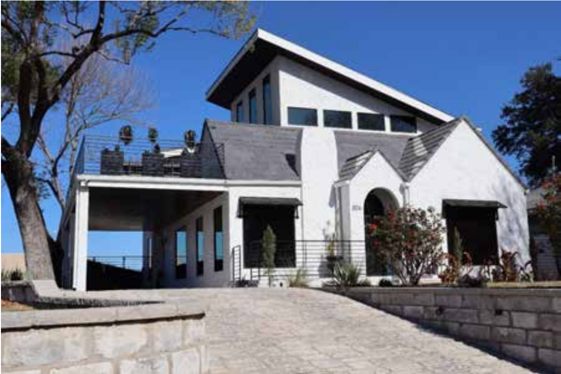
Resource 337: 806 East 13 th Street. View facing northeast.
