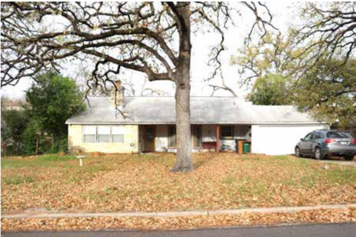
Resource 166, Contributing: 4204 Bradwood Road. View facing west.
