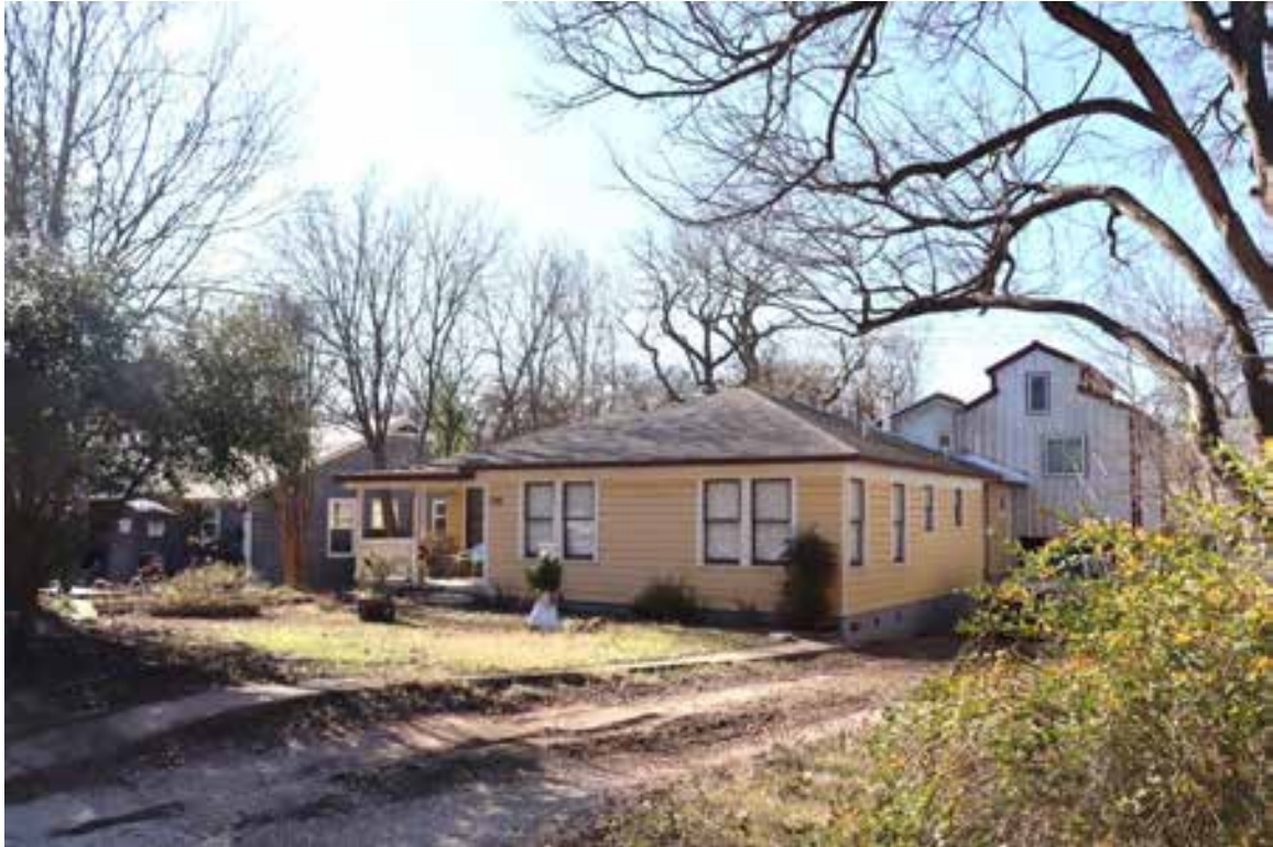
Dancy Street (3200 block). Outside project APE. View facing southwest.
