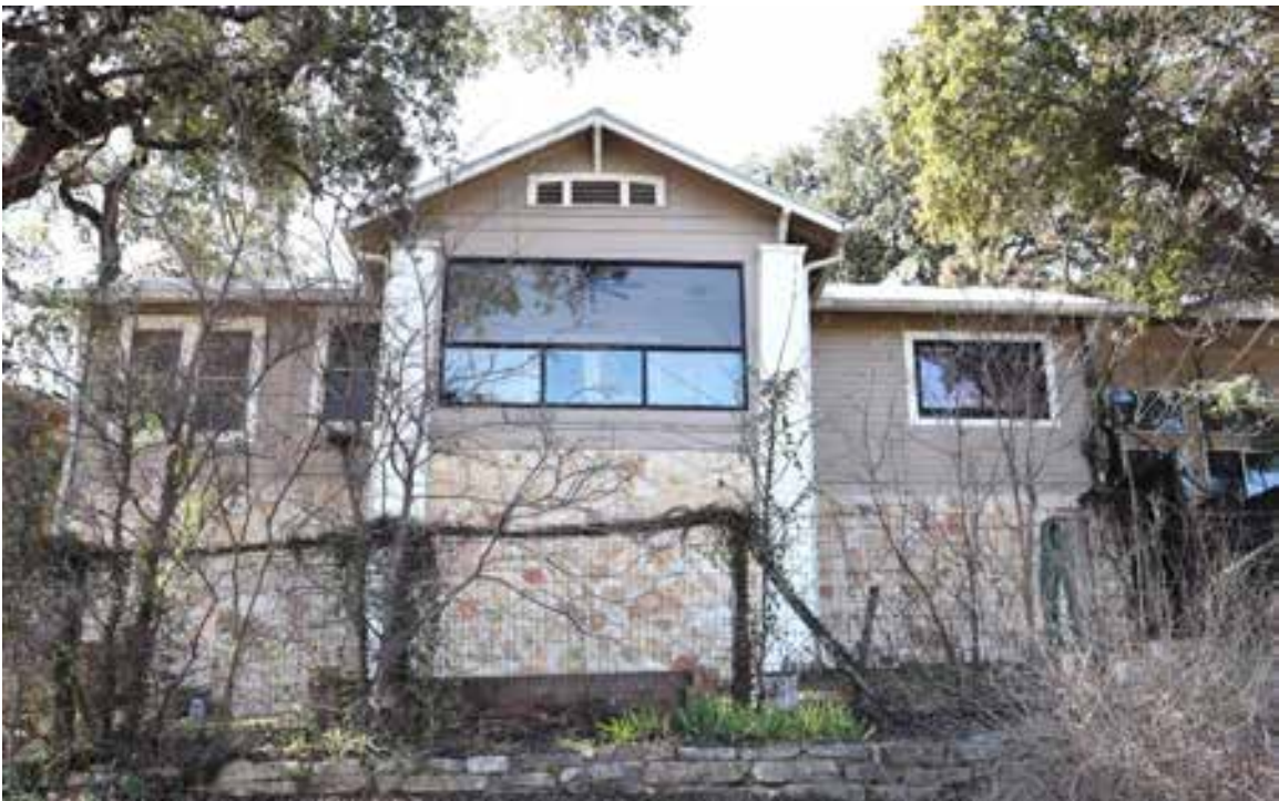
Resource 467, Noncontributing: 1013 East Riverside Drive. View facing southwest.
