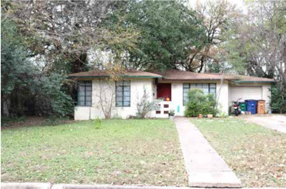
Resource 118: 4510 Elwood Road. View facing northwest.
