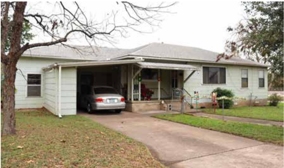
Resource 127: 1028 Ellingson Lane. View facing northeast.
