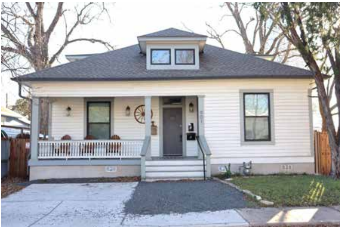
Resource 433, Contributing: 901 Spence Street. View facing southeast
