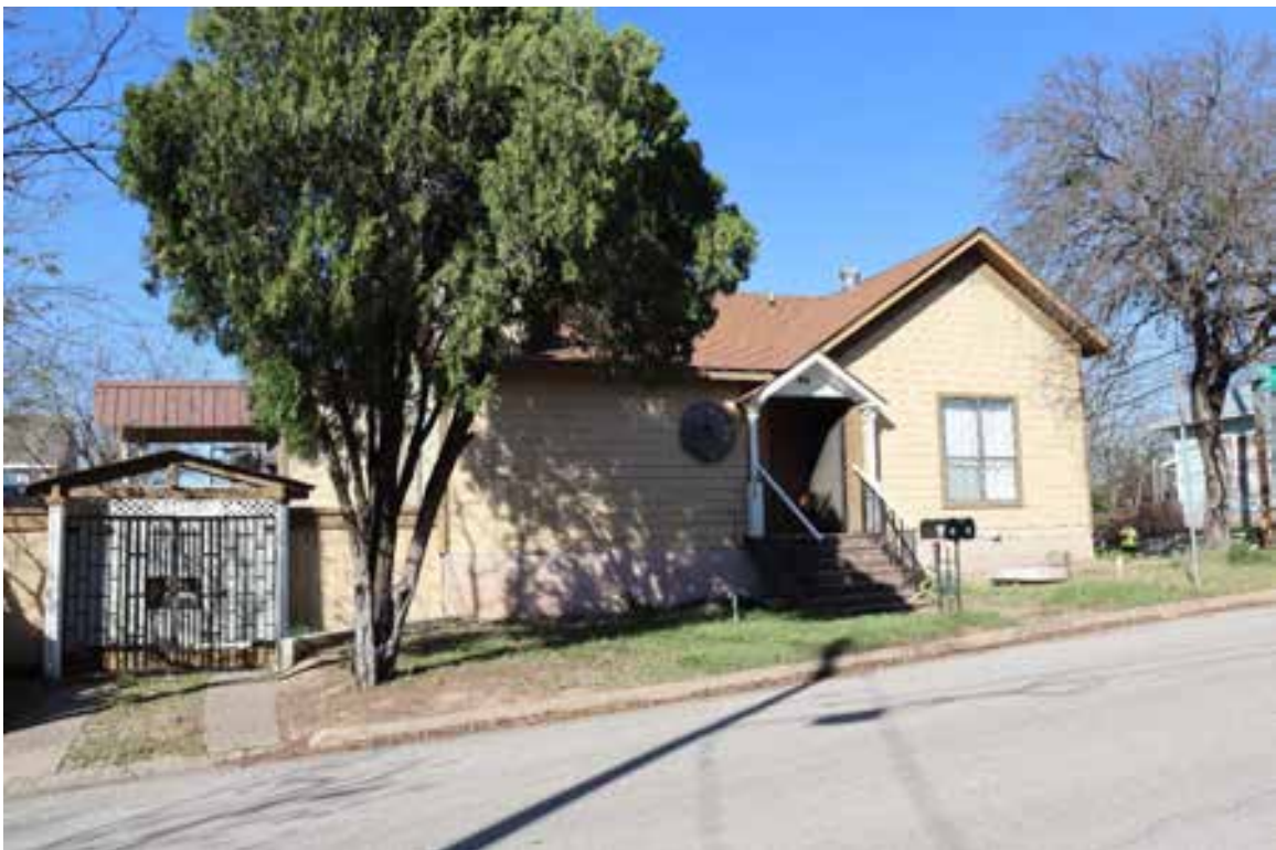
Resource 325: 910 East 15 th Street. View facing northeast.
