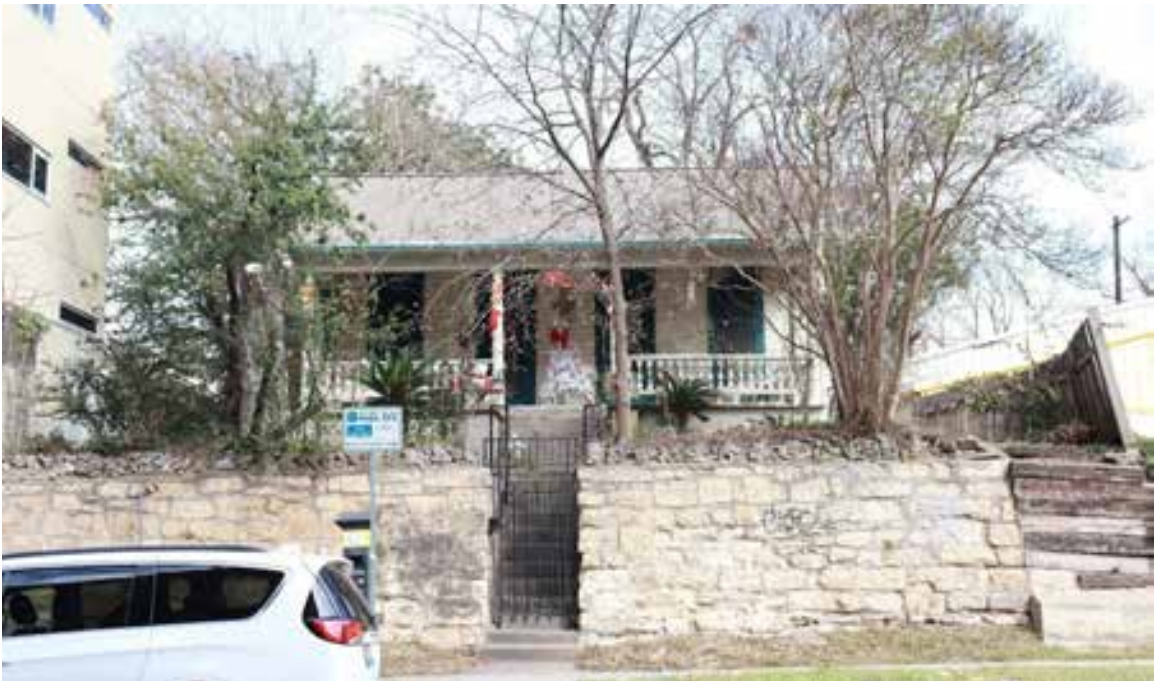
Resource 380: 906 East 6 th Street. View facing northeast.
