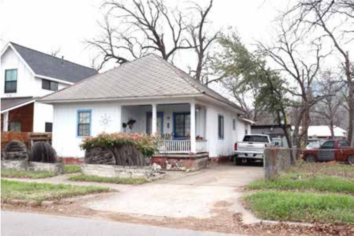
Resource 414A: 906 East 2 nd Street. View facing northwest.
