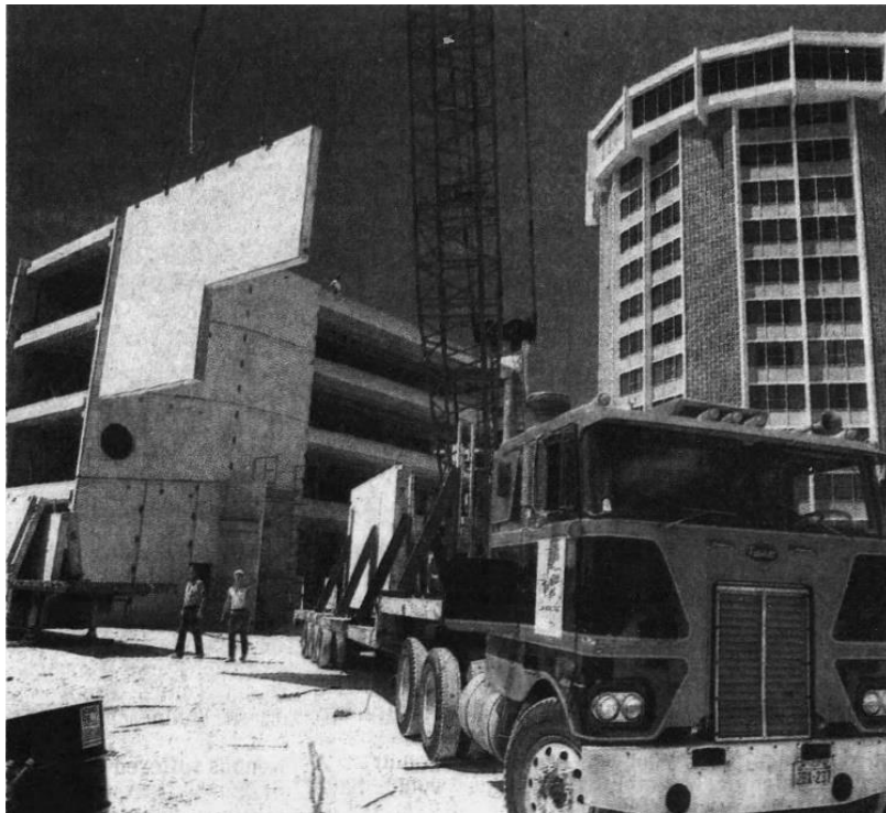
Figure 89. 1984 construction of the 11-story second building. Note the original windows and vertical bands on the 1966 building. 418
