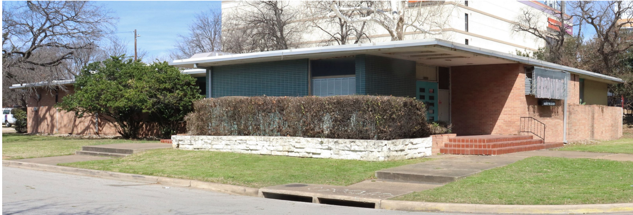
Elgin Butler Brick Company Main Office (Austin Chronicle): 4001 North I-35
