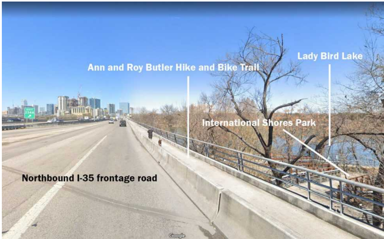
Photo 1: A view of the Ann and Roy Butler Hike and Bike Trail adjacent to the northbound I-35 frontage road bridge over Lady Bird Lake. International Shores Park and the Ann and Roy Butler Hike and Bike Trail in the park are seen on the right. This photo faces north. Photo by Google Street View 2021.
