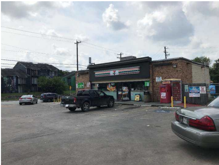
Photograph 44: A view of Map ID 332, 7-Eleven 12702, an LPST (3 listings) and PST site. This site is of moderate risk to the project.
