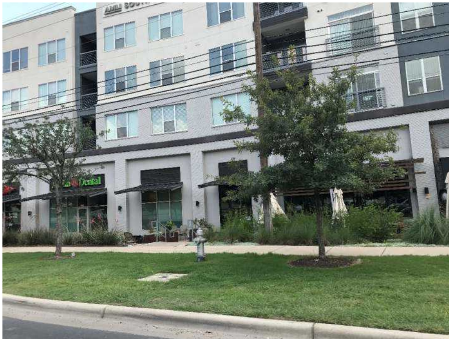
Photograph 48: A view of Map ID 281, formerly named Diamond Shamrock 236, an LPST and PST site. This site is of moderate risk to the project.
