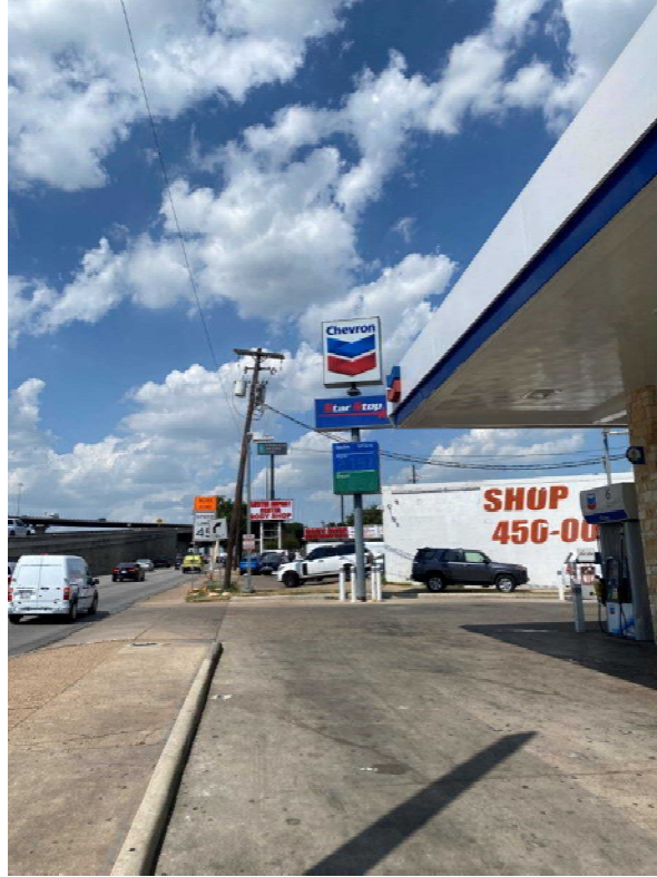
Photograph 3. A view of Map ID 63, Chevron. This site is a PST and LPST site. Partial ROW acquisition is planned for this site and is of low risk to the project.
