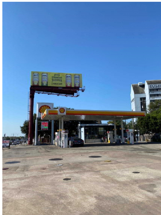
Photograph 2. A view of Map ID 83, Shell Food Mart. This site is a PST and LPST site and is of low risk to the project.
