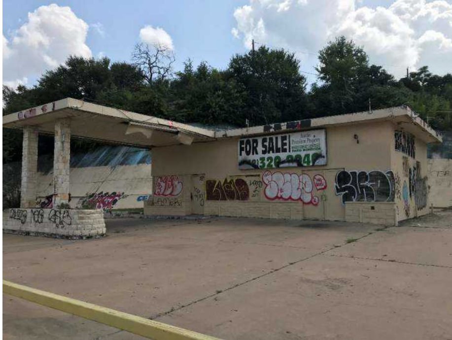
Photograph 47: A view of Map ID 100, Gulf Service Station, a HISTGWCC and VCP site. This site is of moderate risk to the project.
