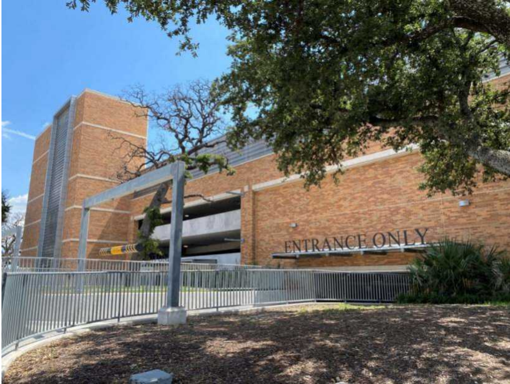
Photograph 23: A view of Map ID 55, which lists a FRSTX site. This location is of no risk to the project.
