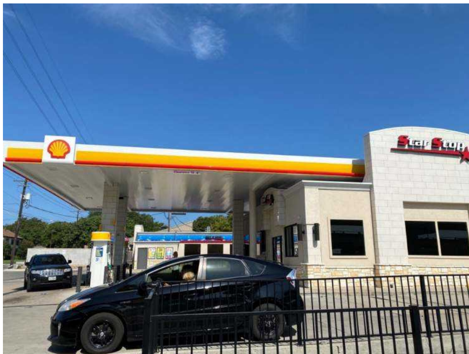
Photograph 16. A view of Map ID 4, Star Stop 35, an active PST site. ROW acquisition is planned for the site and is of low risk to the project.
