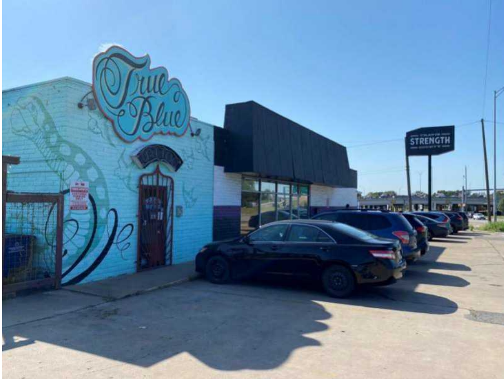
Photograph 11. A view of Map ID 37, Highland Market. The site is an LPST, PST, and IHW site. Partial acquisition is planned for the site and is of high risk to the project.
