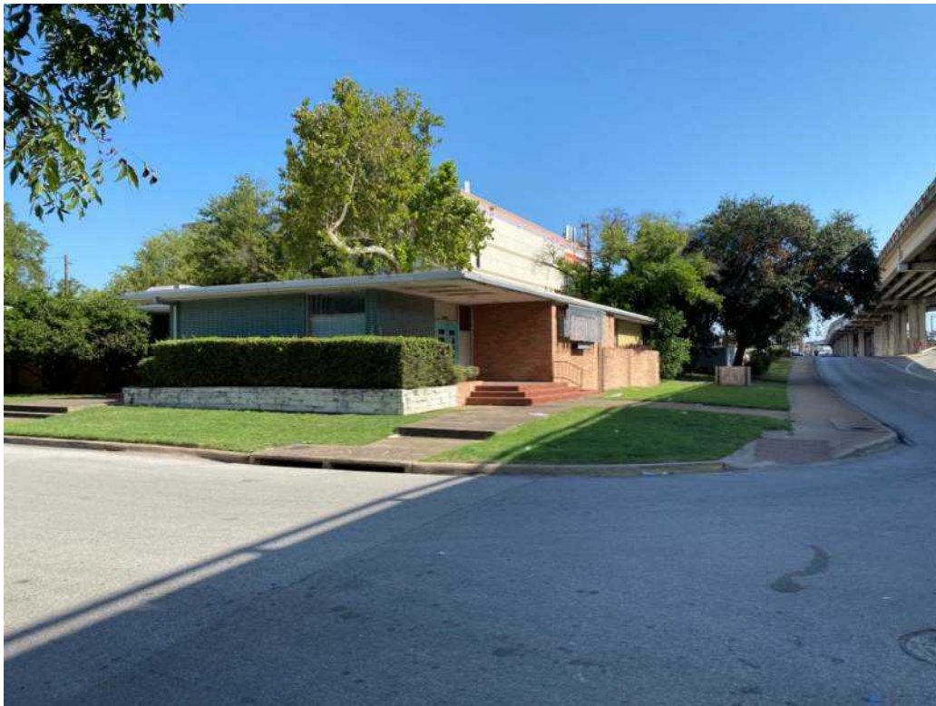
Photograph 14. A view of Map ID 14, Elgin-Butler Brick, a former PST site. ROW acquisition is planned for the site and is of low risk to the project.
