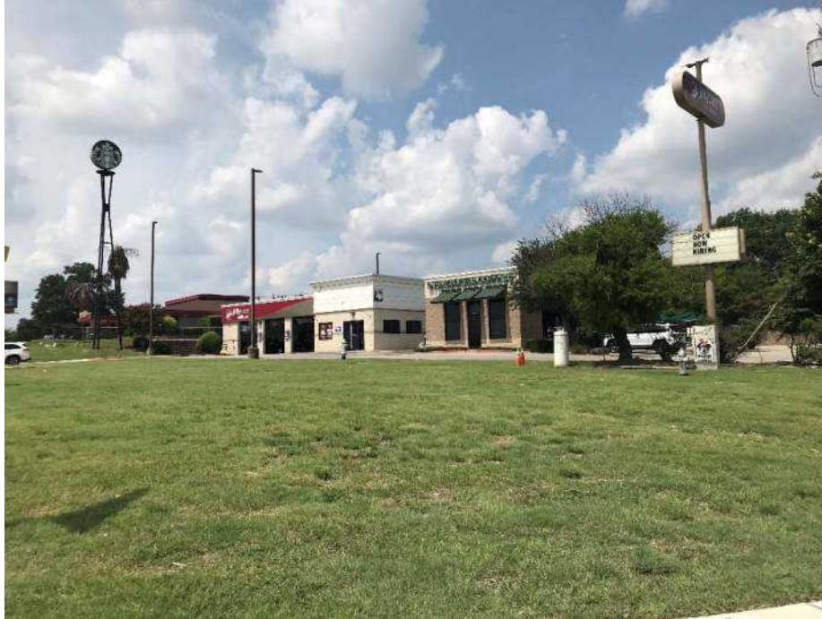
Photograph 45: A view of Map ID 114, Jiffy Lube #3042, an LPST and PST site. This site is of no risk to the project.
