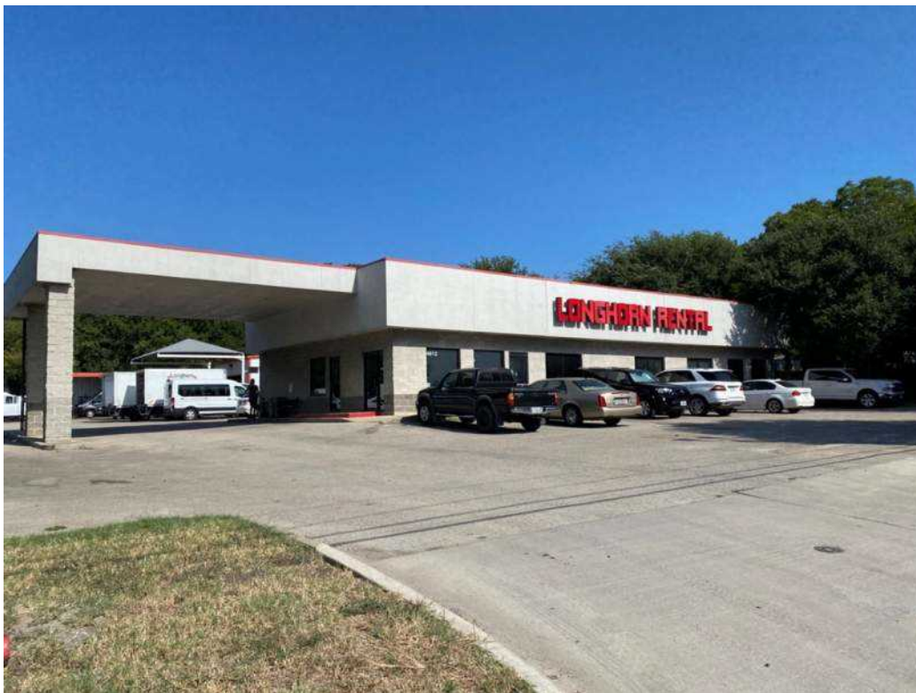
Photograph 10. A view of Map ID 79, Longhorn Rental. The site is a PST site and is no risk to the project.
