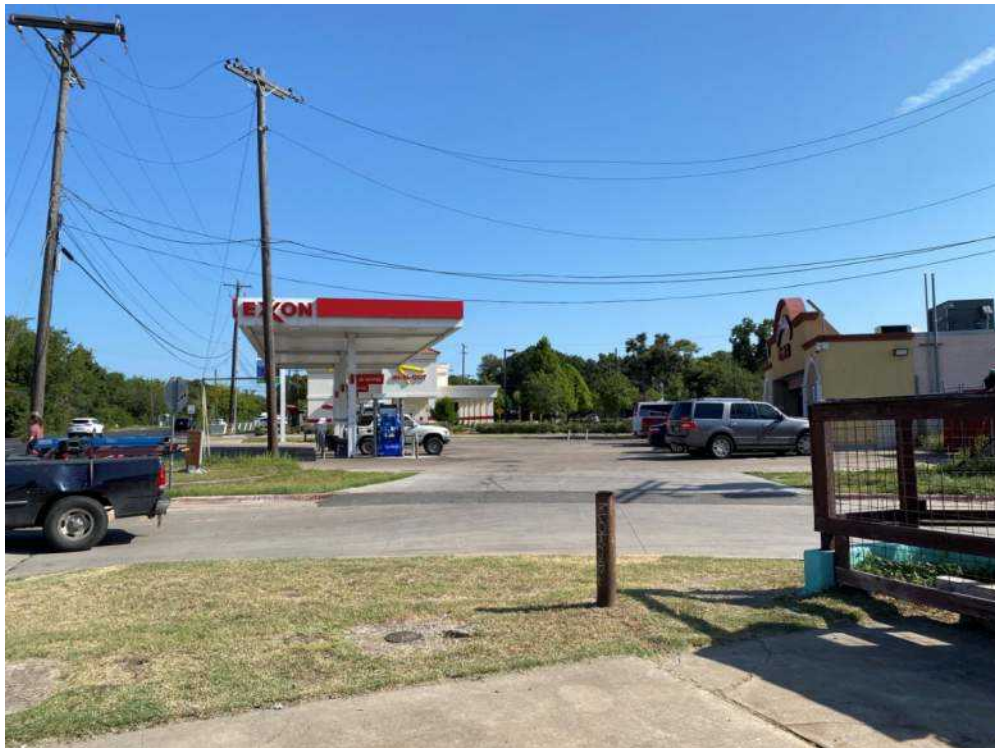
Photograph 12. A view of Map ID 37, Exxon, an active PST site. Partial acquisition is planned for the site and is of high risk to the project.
