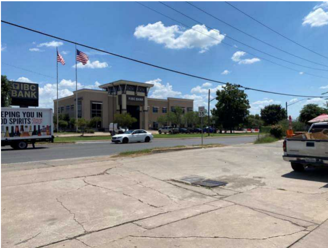
Photograph 38: A view of Map ID 7, Former Espinoza Service Station. The site is a PST, LPST, and GWCC site. This site is of moderate risk to the project.
