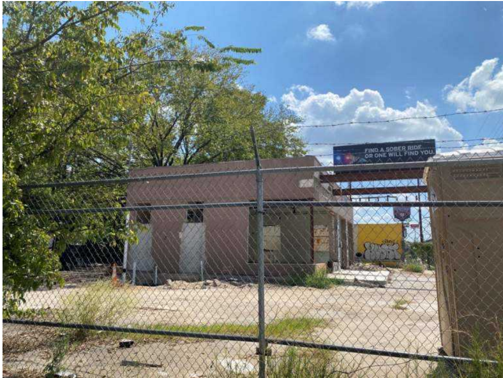
Photograph 19. A view of Map ID 1, W and G Automotive, a PST and LPST site. ROW Acquisition is planned for the site and is of high risk to the project.
