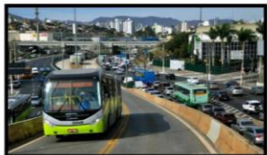
Example of dedicated bus lane for bus rapid transit.
