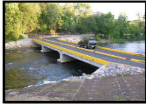
Example of a concrete bridge (not representative of all possible project types).
