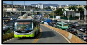
Example of dedicated bus lane for bus rapid transit.
