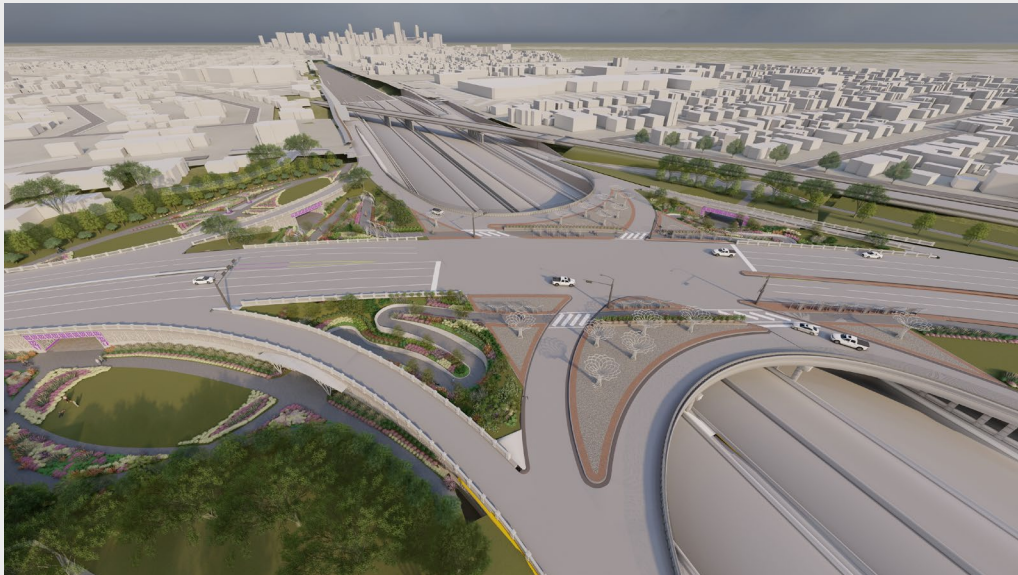
September 2023 Design: Single-Point Urban Interchange (SPUI)
